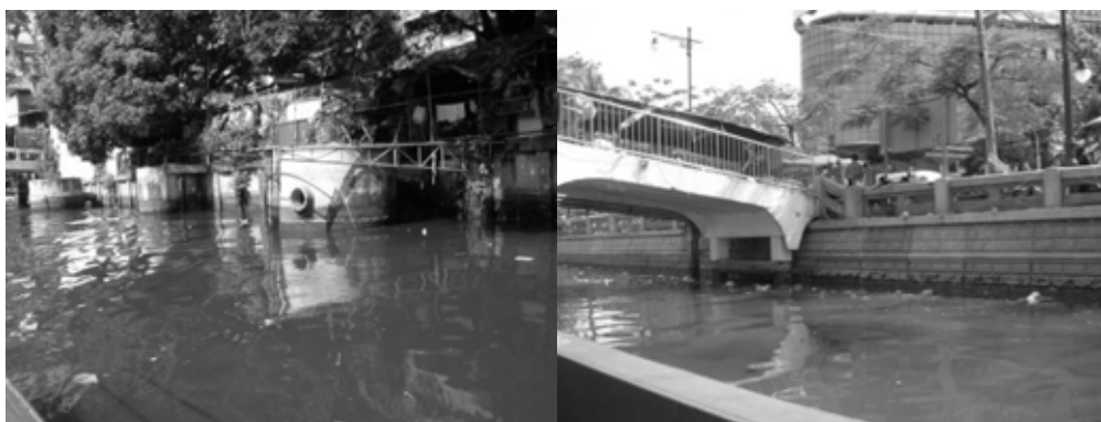
Photo A3.14 Interceptor
