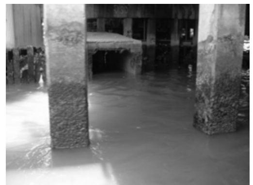
Photo A3.3 Drain Culvert
