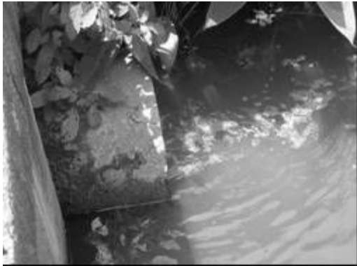
Discharge from interceptor chamber in dry weather
