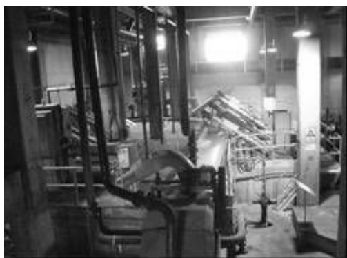
Dynamic separator (swirl grit chamber)
