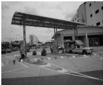
BRT vehicle depot (expansion of WWTP)
