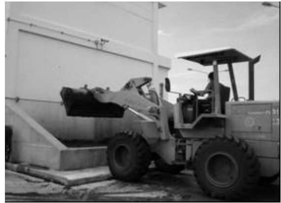
Dumping of sludge cake
