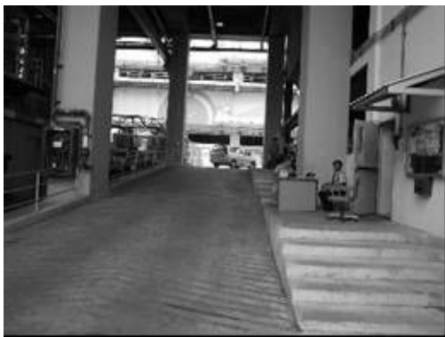
Approach and connecting bridge
