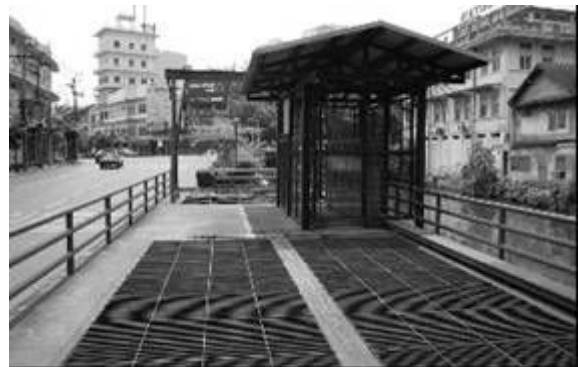
Relay pumping station (pump pit, control panel)
