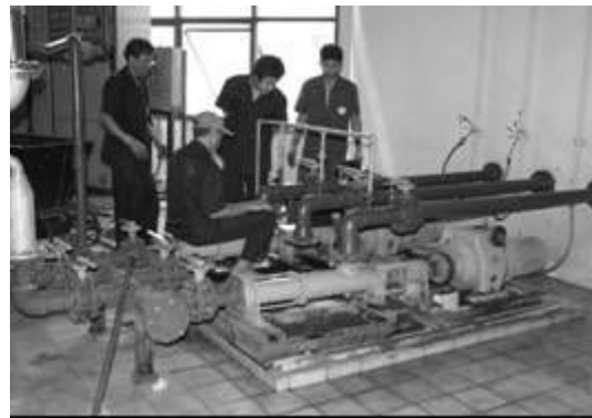
Pump maintenance by BMA staff
