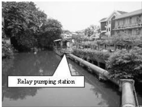
Relay Pumping station and force main
