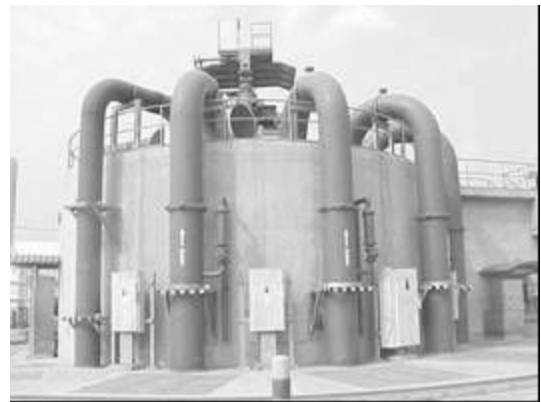
Pumping station (pump pit)
