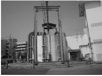
Treatment Process Flow Pump pit
