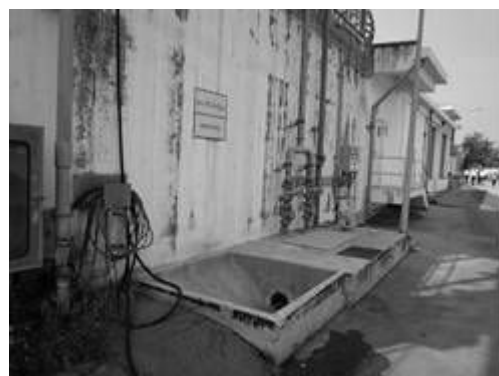
Septic tank sludge receiving pit
