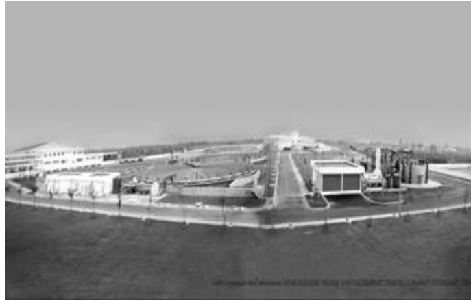
Panoramic view of WWTP
