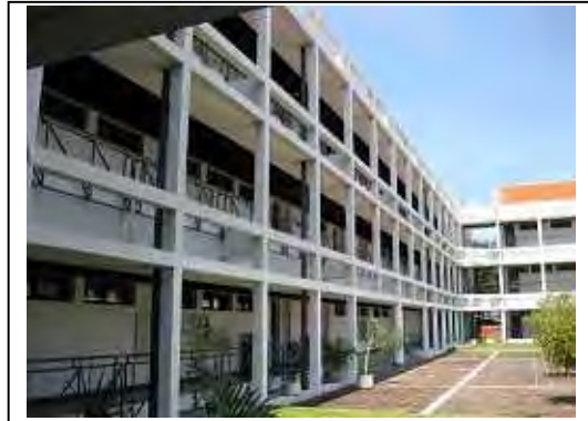
D3 Buildings provided by Japan's Grant Aid in 1980's
