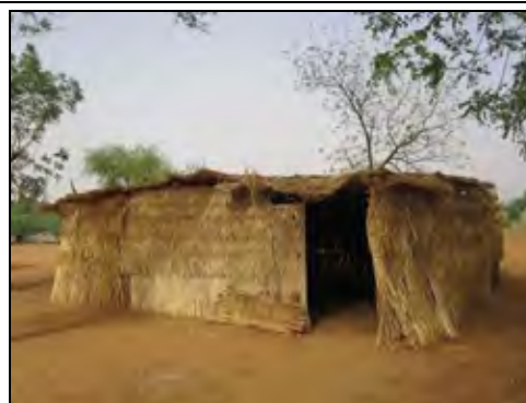
A thatched classroom constructed based on a school activity plan in Biliangue Primary School in Tahoua Region
