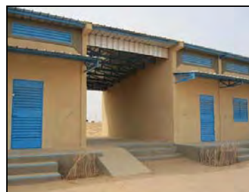
Photo 2 Classroom building constructed by MCC
