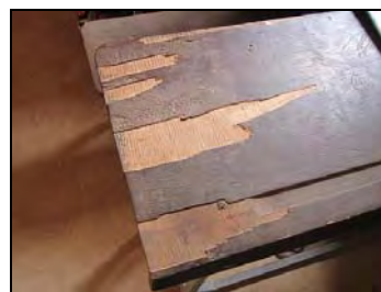
Photo 5 Surface of the desk peeled off
