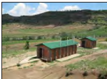
Photo 5 Pit Latrine Buildings
