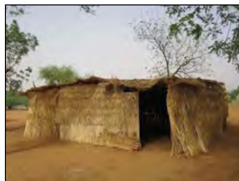
Photo 2 A thatched classroom constructed based on a school activity plan in Biliangue Primary School in Tahoua Region
