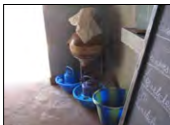
Photo 5 Hand Washing Basins
