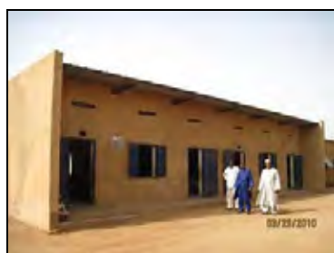
Photo 1 Typical classroom building constructed by the project (Konni Department, Tahoua Region)
