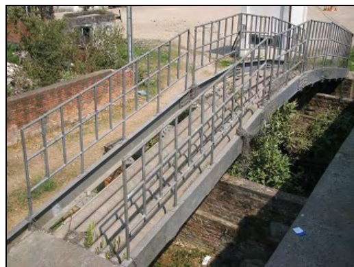
Photo 4: Underground Transmission Line Cable (at river-crossing point)
