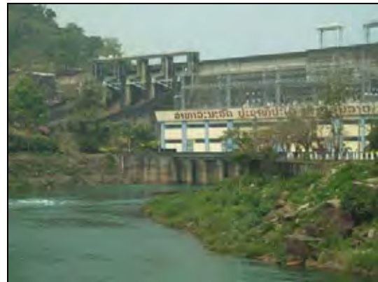
Photo 3: Full View of Nam Ngum I Hydropower Station
