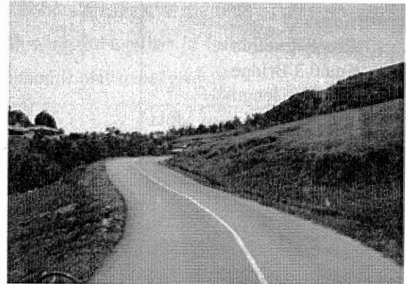
Rehabilitated Dili-Cassa Road
