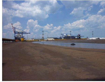
Figure 8: Dent at Berth No.32 41
