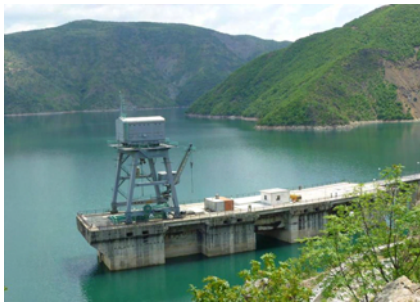
Figure 6: Intake (Reservoir Dam at Fierza Hydropower Station)
