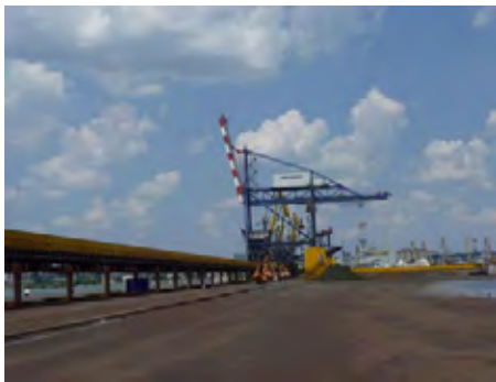
Figure 5: Berth No. 32 (in the far back is the ship unloader procured for the project)
