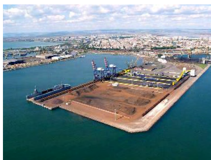
Terminal 2A at the Port of Bourgas
