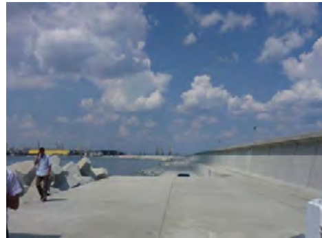
Figure 6: Breakwater Constructed by the Project
