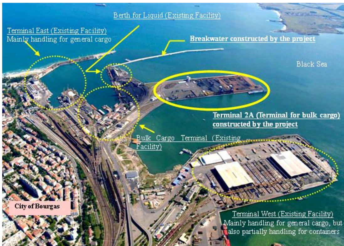
Figure 1: Project Site (1) - The Whole Port of Bourgas
