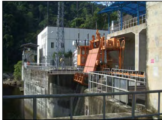
Sipansihaporas Hydroelectric Power Plant
