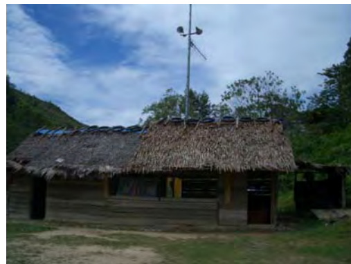
Structure with discharge warning system
