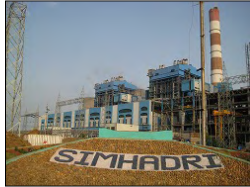
Simhadri Thermal Power Plant
