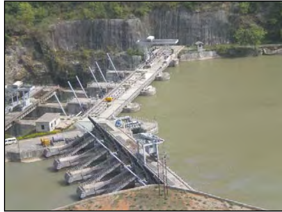
Photo: Water Intake Dam
