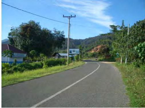
Access road constructed under the project
