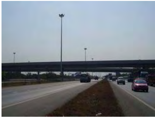
Interchange connecting between North-South Road and Route 345
