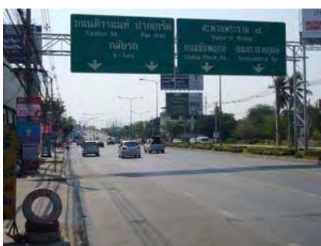
Starting point of the East-West Road (West bound)
