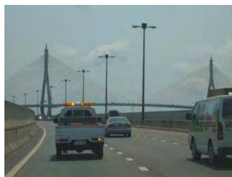
Chao Phraya River Crossing Bridge North-South section
