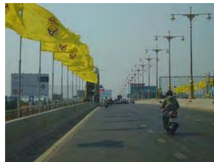
Pak Kret Bridge
