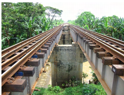
Existing (left) and newly-constructed (right) steel bridges
