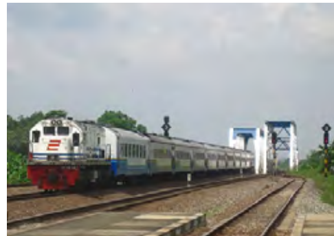
Express train passing over the new track and bridge
