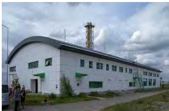
Figure 1 Power Supply Facility Built by the Project
