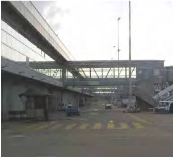
New Passenger Terminal Pier No.1 Built by the Project
