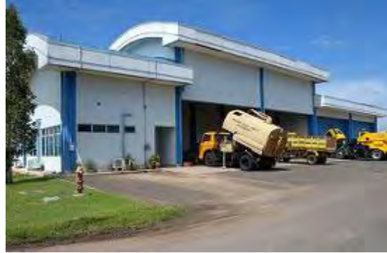
Figure 5 Maintenance and Control Building Built by the Project
