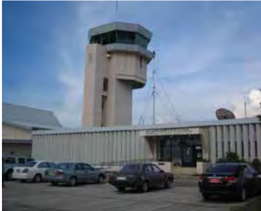
Figure 1 Control Tower Built by the Project (New Bacolod Airport)
