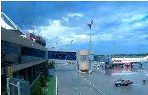
Figure 1 The Passenger Terminal Building and Aerobridge Built by the Project
