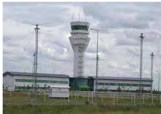
Figure 2 Control Tower Built by the Project
