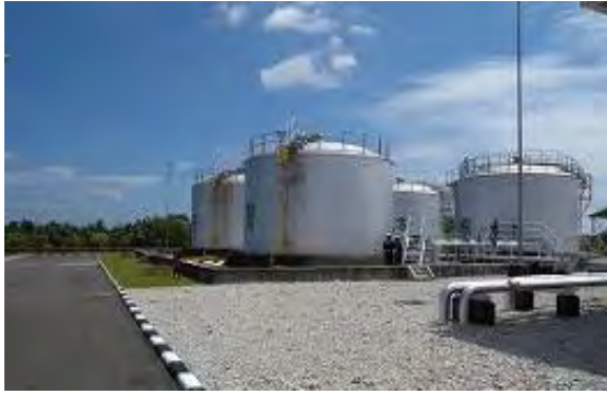
Figure 4 Fuelling System Built by the Project.
