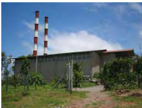
Figure 4 Incinerator Repaired by Project
