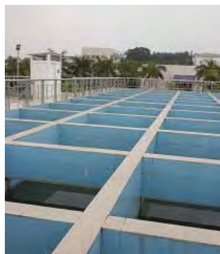
Nanning Sanjin Water Plant Flocculation Pond
