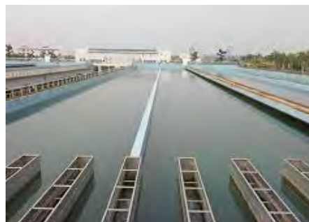
Nanning City Sanjin Water Plant Sedimentation Pond
