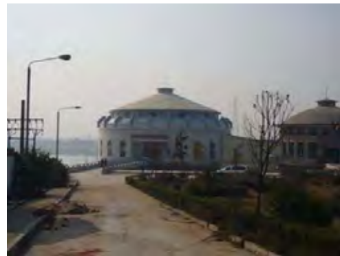
No.8 Water Plant Intake Facility
