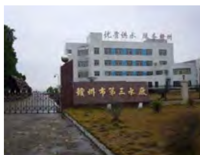
Ganzhou No.3 Water Plant
