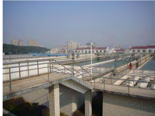
No.8 Water Plant Sedimentation Pond
