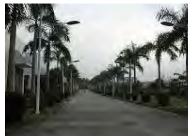
Sanjin Water Plant with green plants
