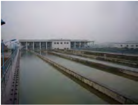
Nankang (No.2 Water Plant) Sedimentation Basin
