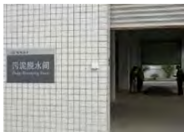
Sludge treatment facility at Sanjin Water Plant
