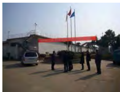
No.8 Water Plant Main Entrance
