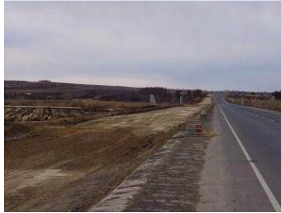
Fig. 3 Construction of Widening the Second-class Road
