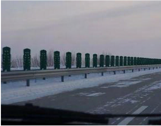
Fig. 2 Construction of Median Divider Strip on First-class Road
