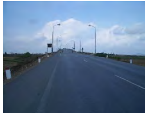
National Highway No.10
