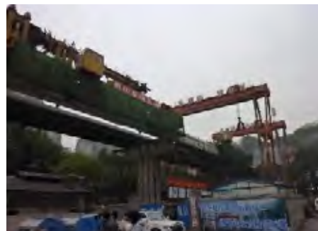
Figure 7: Monorail Line 3, which is being constructed at present
