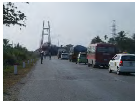
An overloaded truck, which failed to move up the approach to Kien Bridge, was stranded
