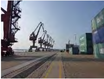
Figure 2: Berth and Cranes of this Project
