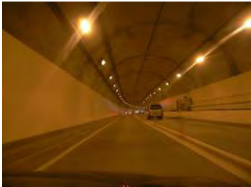
Conditions inside the tunnel
