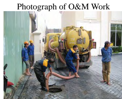
Maintenance of drain by HSDC staff
