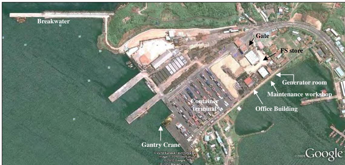
Figure 3: Key construction at Tien Sa Port
