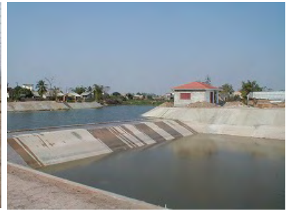
Spillway B at Yen So Pumping Station
