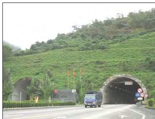
Main Tunnel (right) and Evacuation Tunnel
