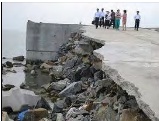
Damaged Breakwater
