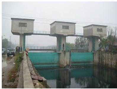
Thanh Liet Flood and Control Gate
