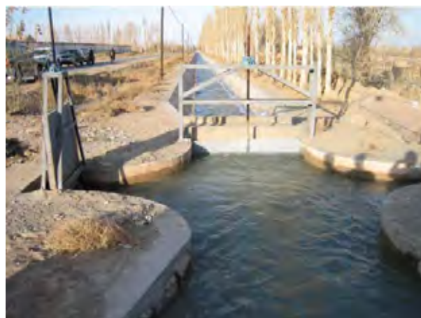
Completed canal with concrete lining
