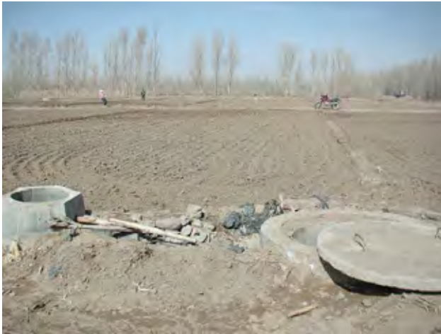
A one-mu farm is irrigated by a set of underground pipe irrigation facility whose concrete holes containing an outlet (left) and control valves (right) are installed on the ground. Farmers are doing land preparation for coming planting season.
