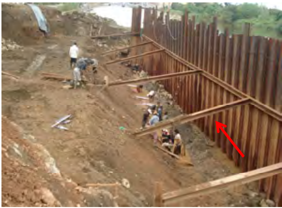
Date: September 30, 2010 Under Construction
