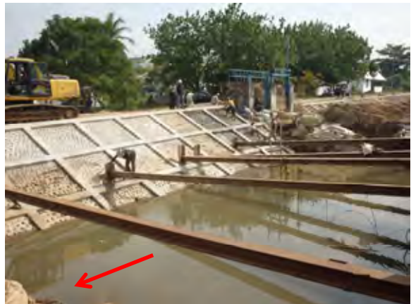
Date: January 22, 2011 Under Construction
