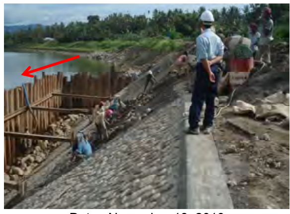
Date: November 18, 2010 Under Construction
