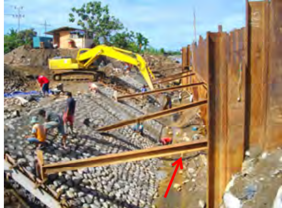
Date: October 06, 2010 Under Construction
