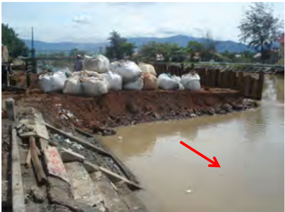
Date: December 27, 2010 Under Construction
