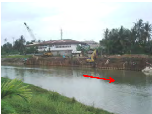
Date: October 12, 2010 Under Construction
