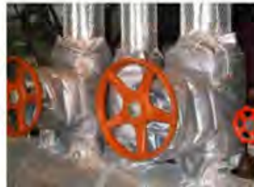
FIG.-6-2 : An Example of Insulation Jacket on Valve:
