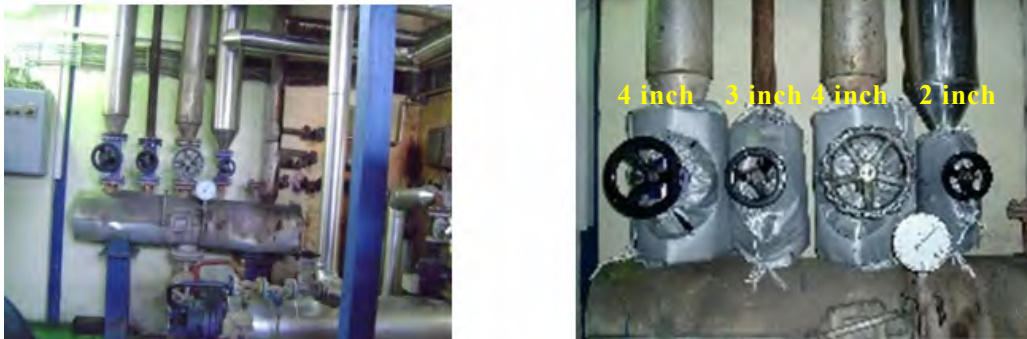
Figure 6-6 Installation of Insulation Jackets (Left: Before Installation, Right: After Installation)
