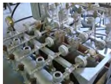
Hands-on Facility of Steam Trap
