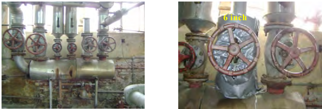
Figure 6-8 Installation of Insulation Jacket (Left: Before Installation, Right: After Installation)
