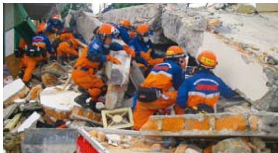
Search activities at collapsed building
