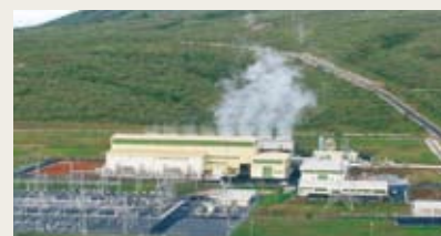
Existing Olkaria II Geothermal Power Station in operation
