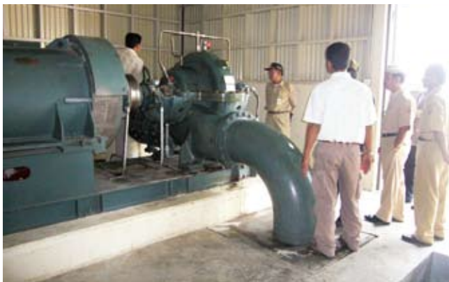
Inspection of a generator
