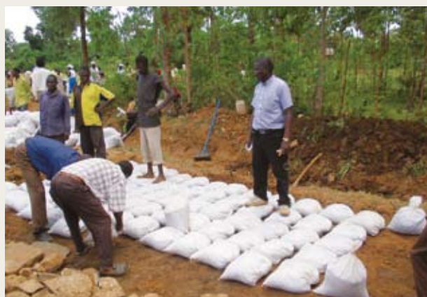
A farmers’ group restores a road in the village using sandbags. The act of cooperation helped to unify the group.
