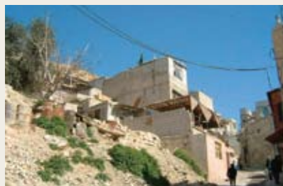
JICA conducts studies on unofficial residential areas.
