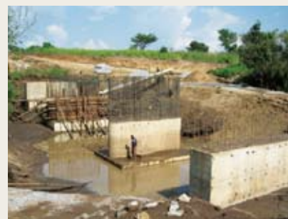
Construction site of bridge linking Otwee and Anaka
