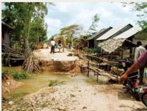
National Highway No. 1 prior to rehabilitation
