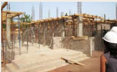
Construction of health center in progress
