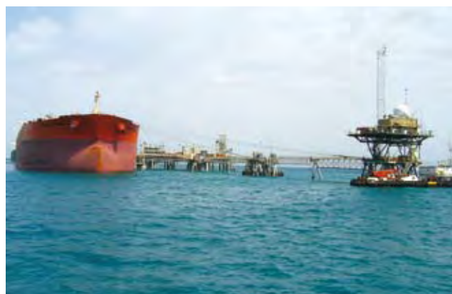
Offshore crude export terminal from which about 80% of crude oil exports are shipped from Iraq; export capacity will be doubled as a result of aid provided through an ODA Loan project.
