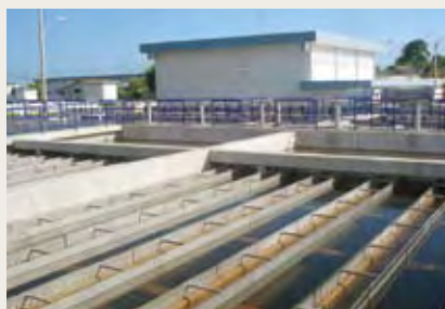
Water treatment plant after improvements
