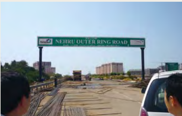
On-ramp for the Hyderabad Outer Ring Road (under construction) in India.
