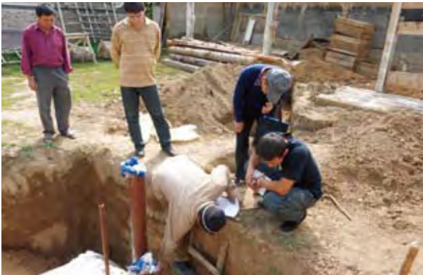
Construction of a biogas plant in the Kyrgyz Republic
