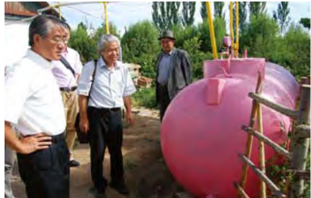
Inspection of a biogas plant
