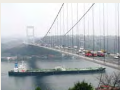
Second Bosphorus Bridge in Turkey
