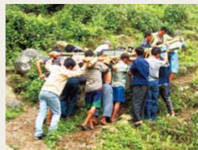
Transporting a transformer up a mountain road (Bhutan rural electrification)
