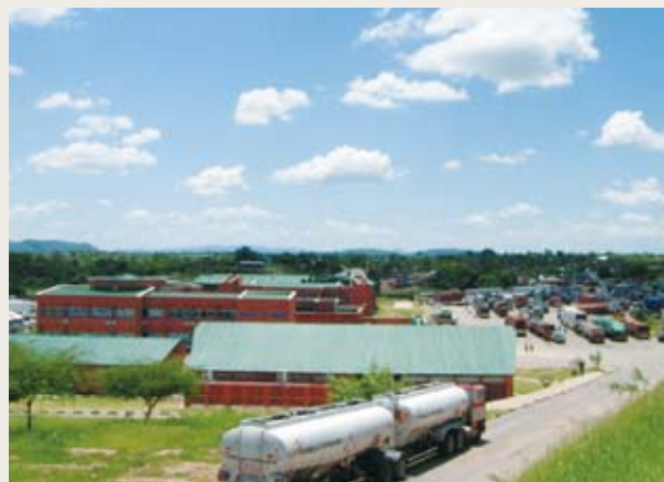
A new freight terminal completed at the Chirundu OSBP. The large reduction in border-crossing times is expected to yield various spillover effects including but not limited to improved commercial value of agricultural products, as a result of reduced transport cost.
