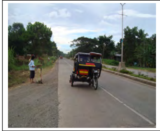
Road expanded to four lanes
