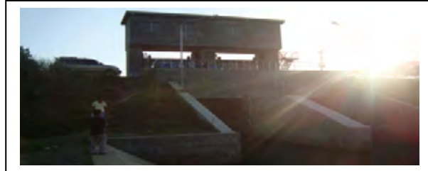
Flood Sluice Gate constructed by the Flood Control Component
