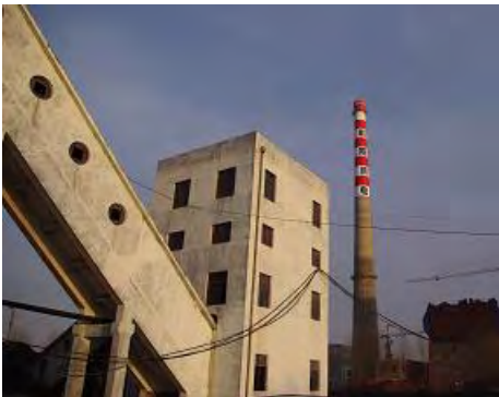
Fig. 5 Heat Supply Equipment in Jidong
