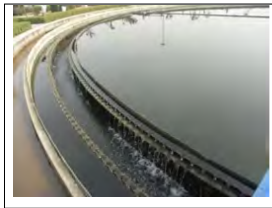
Expansion Project of Changsha No.1 Sewage Treatment Plant: Final Settling Tank
