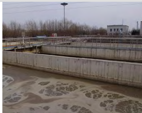
Mudanjiang Sewage Treatment Plant
