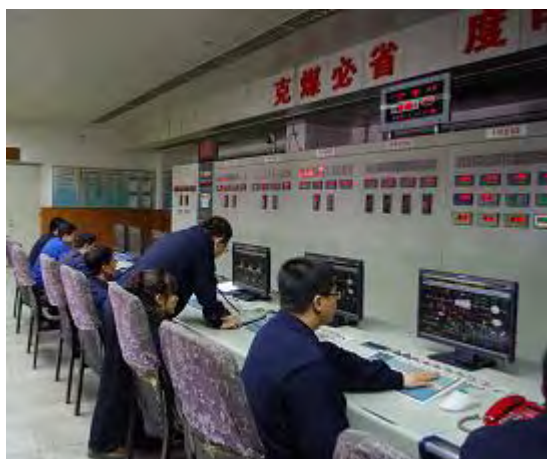
Fig. 6 3-2. Central Control Office of Mishan Heat Supply
