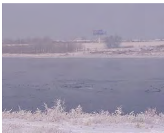
Fig. 6 Songhua River close to the sewage treatment plant in Jilin
