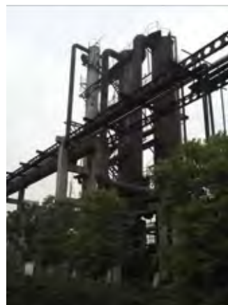
Fig. 7 Sub-project 3-2) Expansion Project of Gas Production Plant in Zhuzhou City: Added coal gas purification equipment (no longer in operation)
