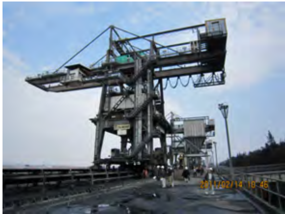
Figure 2.3-23 New unloading facility (Pha Lai)
