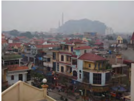
Figure 1-1 Overview of downtown in province of Ninh Binh Ninh Binh power plant presents in center of this picture.
