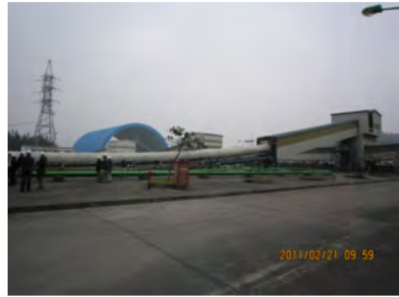
Figure 2.3-28 Stacked coal loading BC (Uong Bi)
