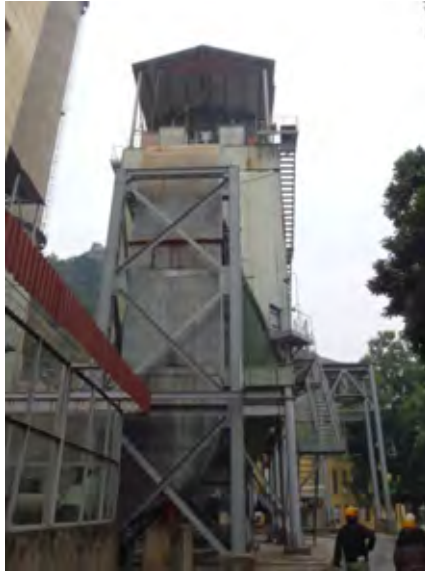
Figure 1.4-2 Dry electrostatic precipitator
