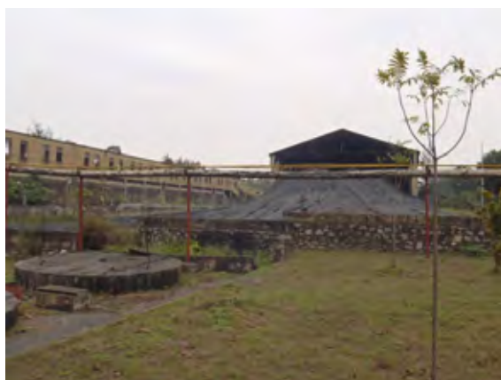
Figure 1.3-5 Overview of the roofed coal storage yard
