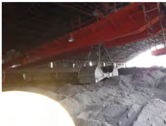
Figure 1.3-6 Inside of the roofed coal storage yard
