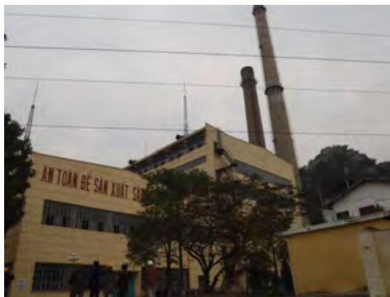
Figure 1-2 Overview of Ninh Binh thermal power plant
