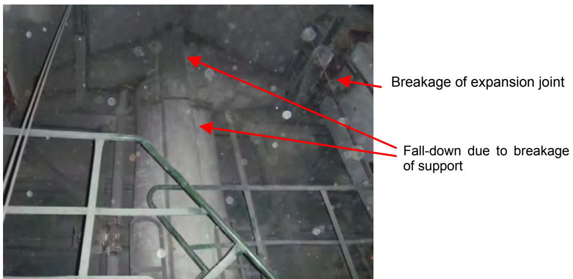
Figure 2.2-5 Duct damage
