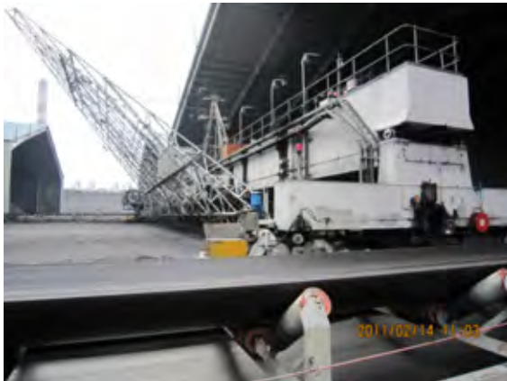
Figure 2.3-25 Stockyard (Pha Lai)
