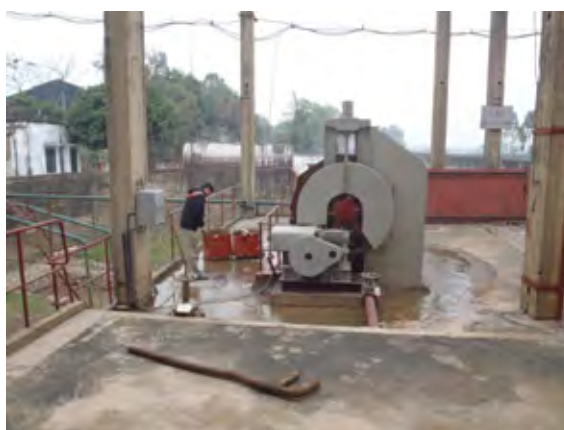
Figure 1.3-17 Rotary screen
