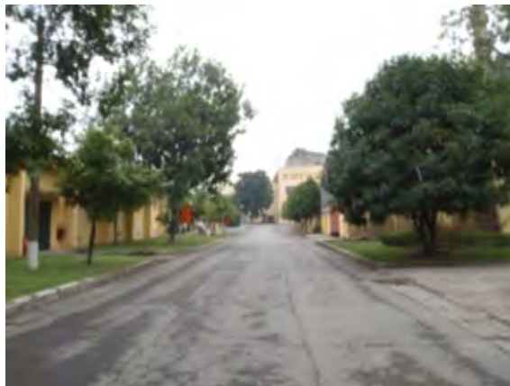
Figure 1.4-3 Main street in the power plant
