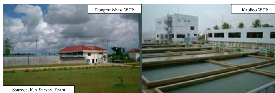
Figure 2.3.12: Dongmakkhay WTP and Kaolieo WTP
