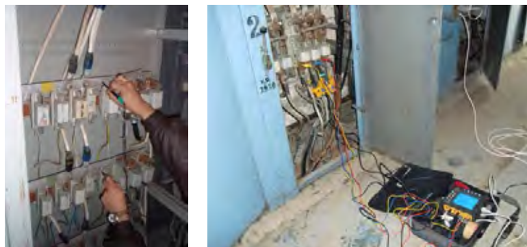
Photo Left : Measuring voltage and frequency
