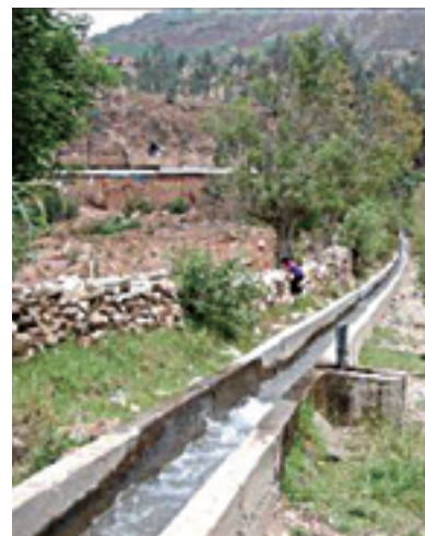
Irrigation channel constructed by this project
