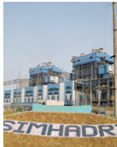
Simhadri Thermal Power Plant
