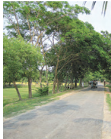
Rural road built by the project (Mymensingh District)
