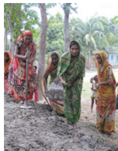
Women's group performing road maintenance work
