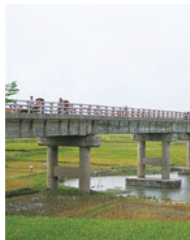
Bridge constructed by the project (Jamalpur District)
