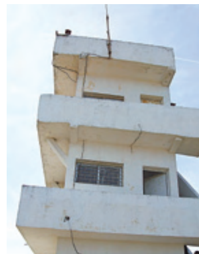
Observation tower constructed by the project
