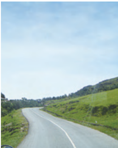
Rehabilitated Dili-Cassa Road
