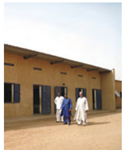
Classroom building constructed by the project (Konni Department, Tahoua Region)
