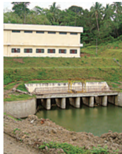
Irrigation pumping station on the East bank of Agusan River
