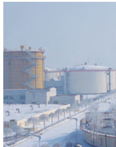
Sewage treatment facility
