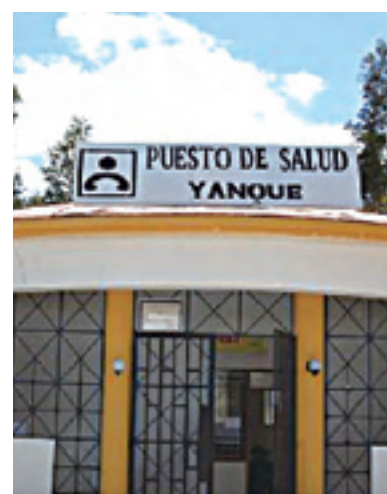
A new health post that was built following the earthquake
