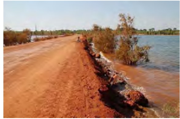
After height of embankment 26 th Nov. 2010
