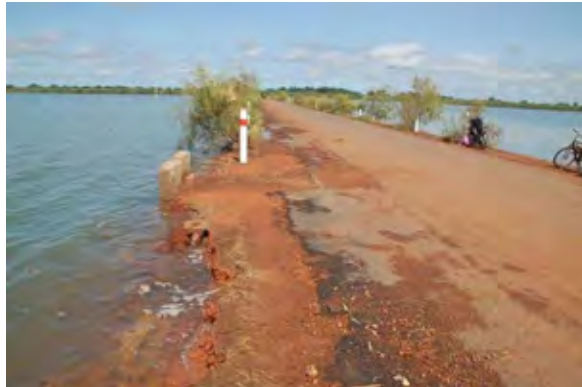
Before height of embankment 16 th Sep. 2010
