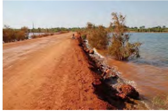
After height of embankment 26 th Nov. 2010
