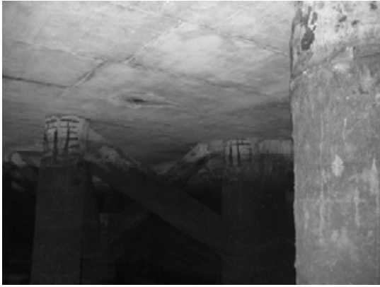
Pile 12D ~ Pile 12E-1
