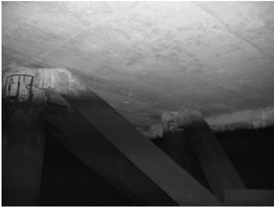
Pile 25D ~ Pile 25D
