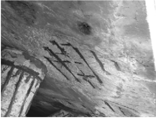
Slab nearby Pile 1B
