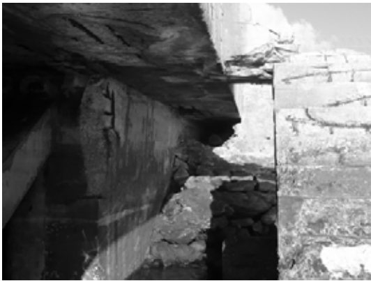
Wall and Slab nearby Pile 1C
