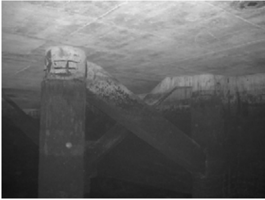
Pile 8D ~ Pile E
