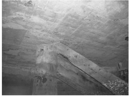
Block 3 Pile 62F
