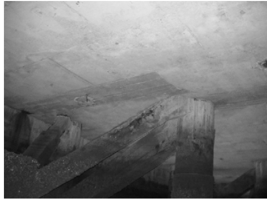
Block 3 Pile 49F
