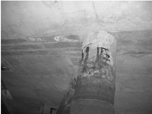
Block 3 Pile 50E-1
