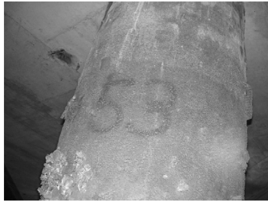
Block 3 Pile 53D
