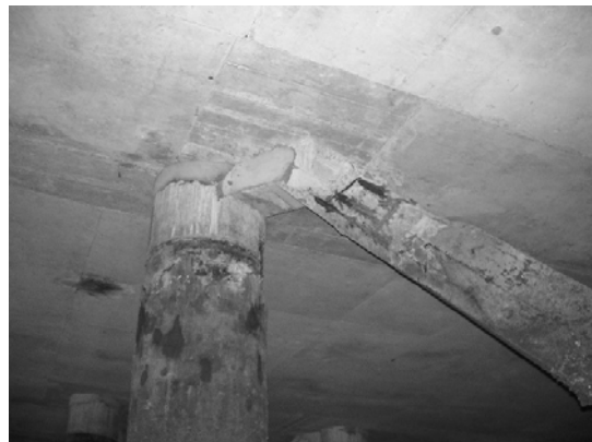
Block 3 Pile 57E-2
