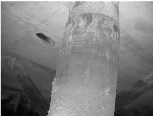
Block 3 Pile 47D-1
