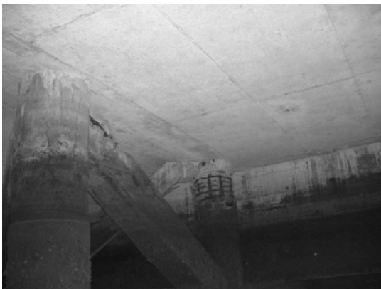
Block 3 Pile 47F ~ 47G
