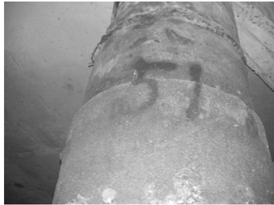
Block 3 Pile 51E-2
