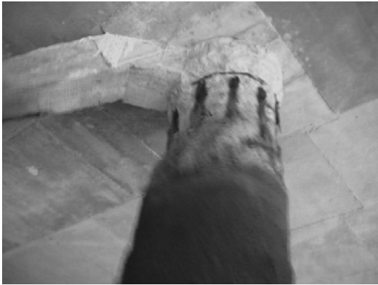
Block 3 Pile 42E-1
