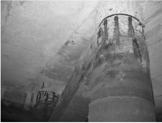
Block 3 Pile 46F ~ 46G-1
