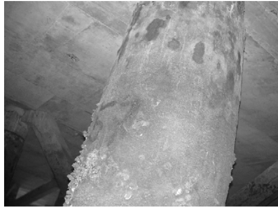
Block 3 Pile 57D
