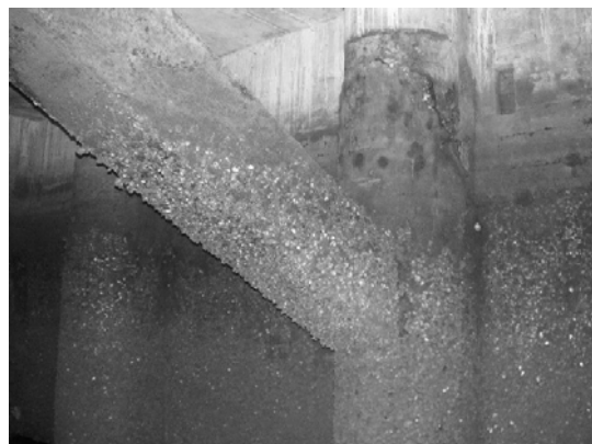
Block 3 Pile 54A
