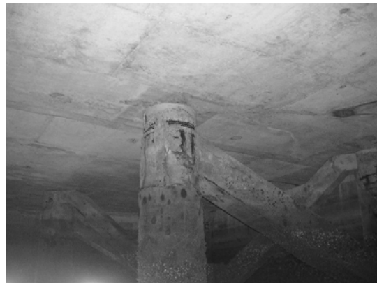
Block 3 Pile 61F
