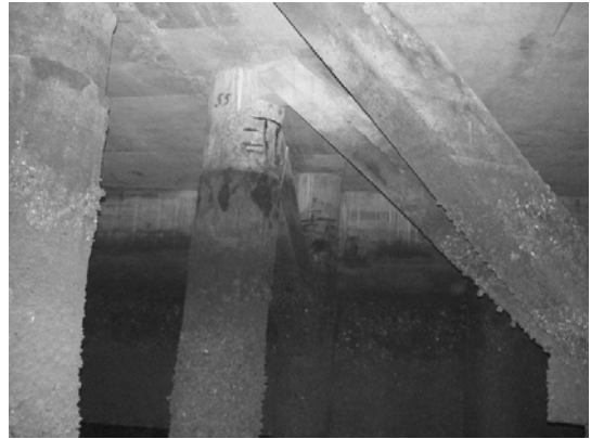
Block 3 Pile 49B
