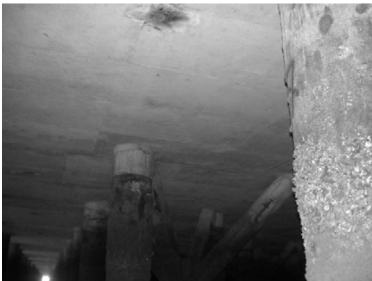
Block 3 Pile 56E-2
