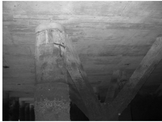
Block 3 Pile 54E-2
