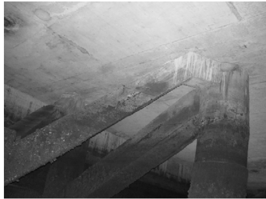
Block 3 Pile 47F
