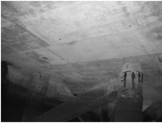
Block 3 Pile 44F
