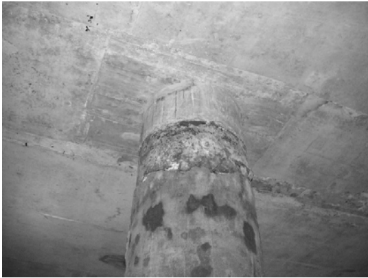
Block 3 Pile 58E-1
