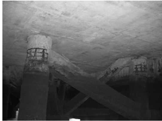
Block 3 Brace bet. Pile 41F & 41G-1
