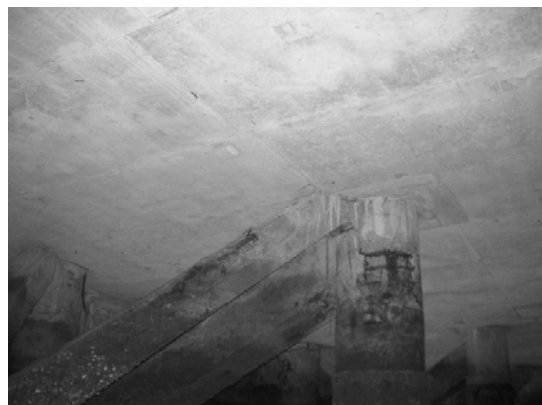
Block 3 Pile 51F-4
