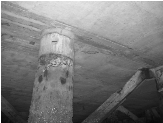
Block 3 Pile 61E-1
