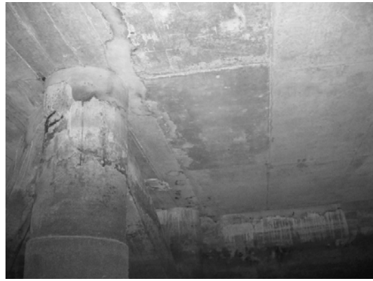
Block 3 Pile 55F
