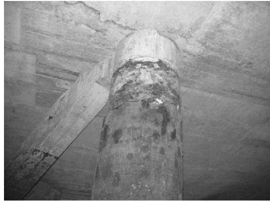
Block 3 Pile 58E-2
