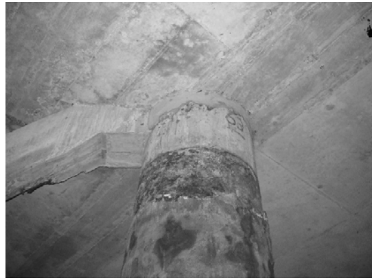
Block 3 Pile 58C
