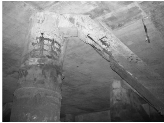
Block 3 Pile 43C-2
