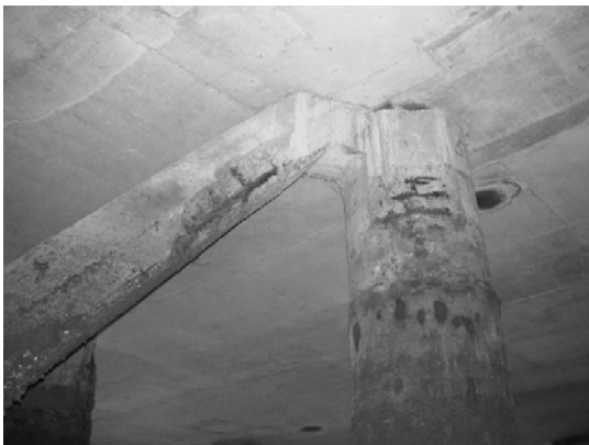
Block 3 Pile 51D-1
