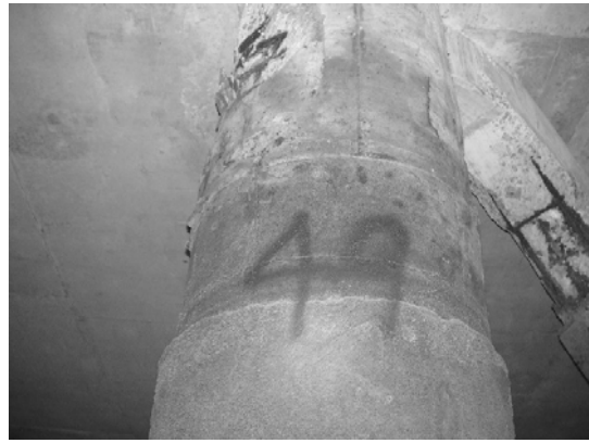
Block 3 Pile 49E-2
