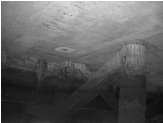
Block 3 Pile 54F ~ 53G
