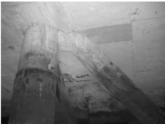
Block 3 Pile 50F
