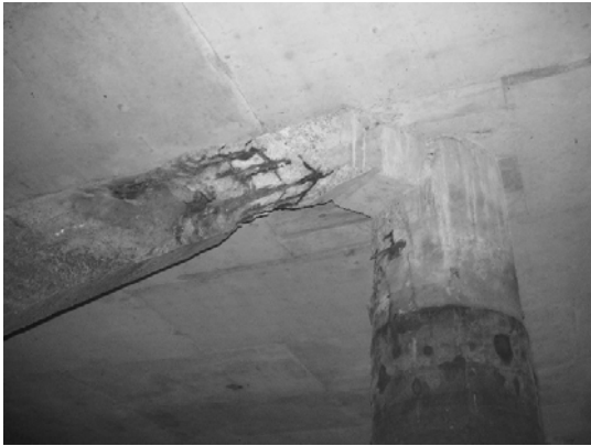
Block 3 Pile 49E-3
