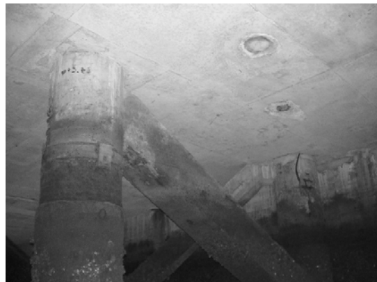
Block 3 Pile 51F-2
