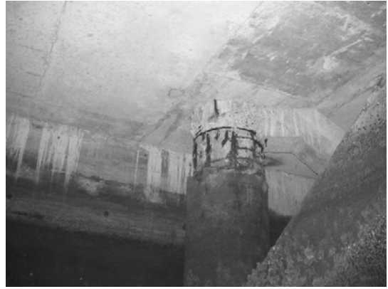
Block 3 Pile 48G
