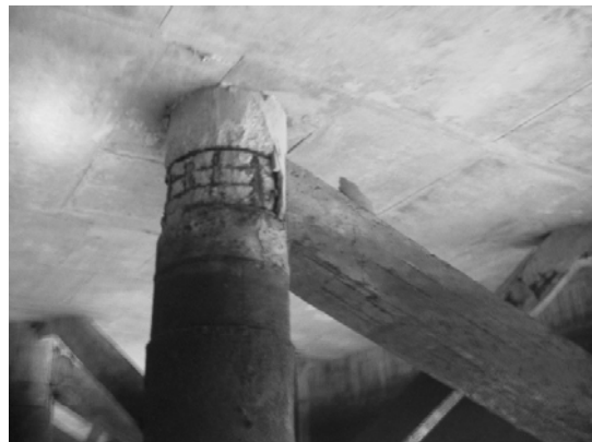
Block 3 Pile 43F
