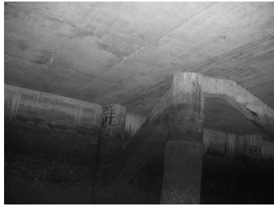
Block 3 Pile 45A ~ 45B
