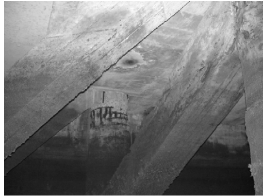
Block 3 Pile 45G
