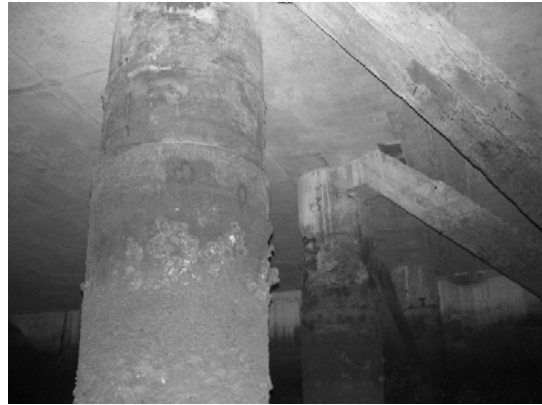
Block 3 Pile 47B
