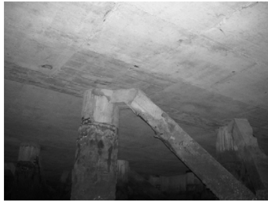
Block 3 Pile 57C-1
