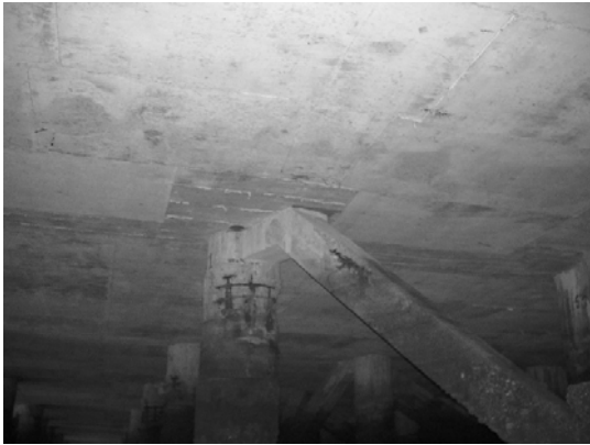
Block 3 Pile 45C-1
