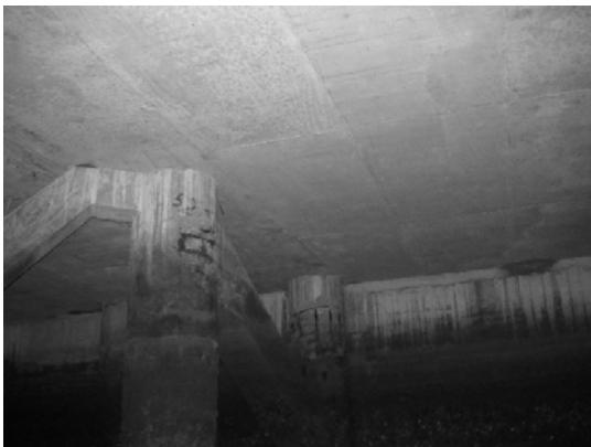
Block 3 Pile 46A ~ 46B
