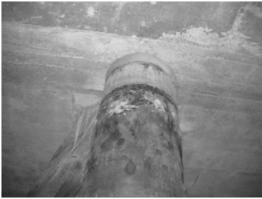
Block 3 Pile 54E-1
