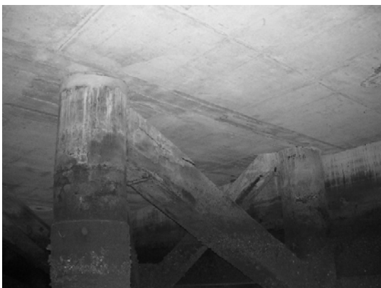
Block 3 Pile 53F ~ 53G
