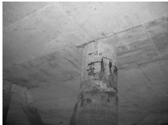
Block 3 Pile 47D-2
