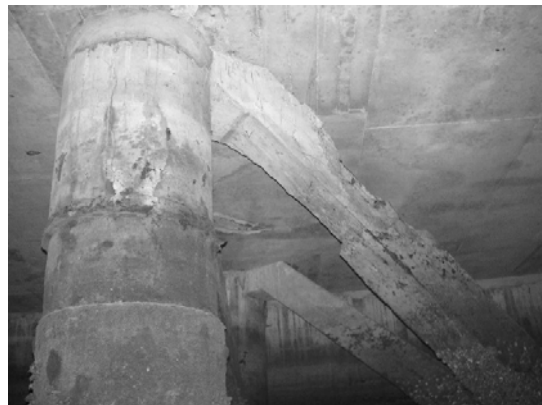
Block 3 Pile 60F
