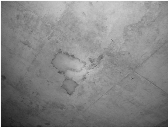
Block 3 Slab bet. Pile 60E & 61E-2
