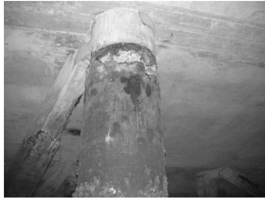
Block 3 Pile 56E-1
