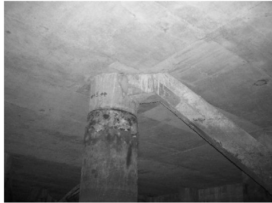
Block 3 Pile 51C-3
