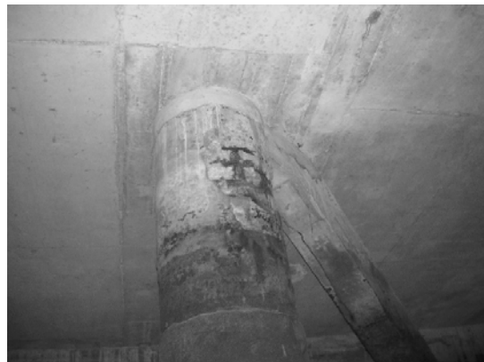
Block 3 Pile 56F
