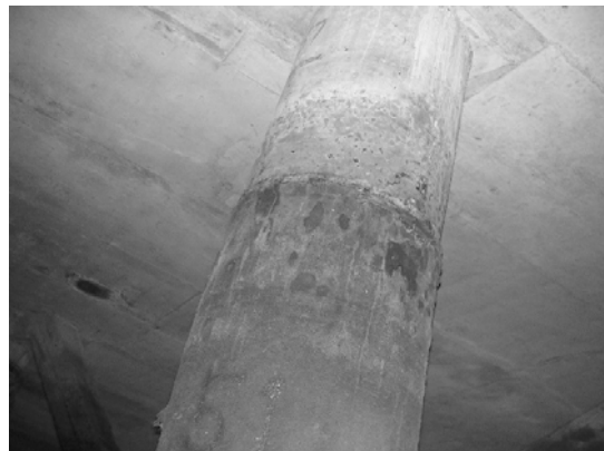
Block 3 Pile 51D-2
