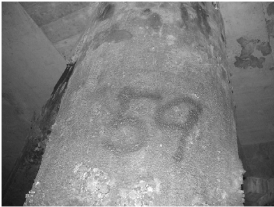
Block 3 Pile 59D
