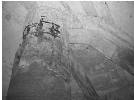
Block 3 Pile 46F
