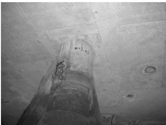
Block 3 Pile 51F-3
