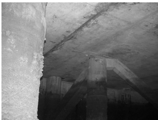
Block 3 Pile 41A ~ 41B
