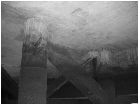
Block 3 Pile 51F-1
