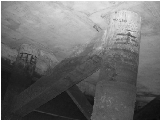
Block 3 Pile 42F
