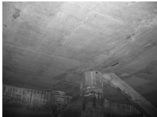
Block 3 Pile 59C
