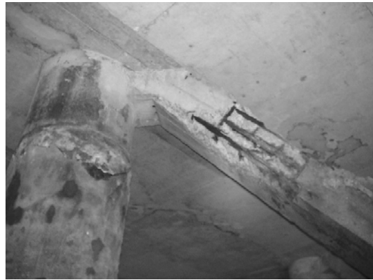
Block 3 Pile 61E-2
