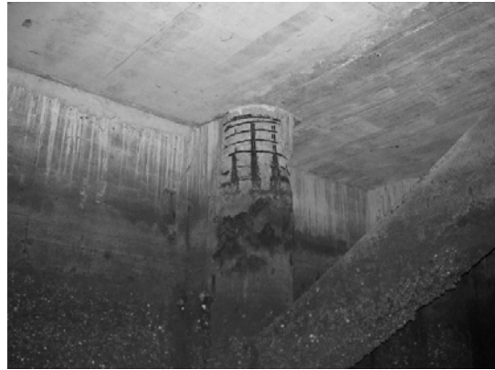
Block 3 Pile 55A
