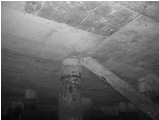
Block 3 Pile 53C
