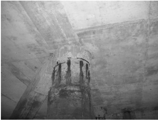
Block 3 Pile 45F-3
