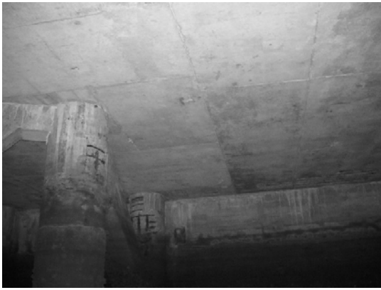
Block 3 Pile 42A ~ 42B-2
