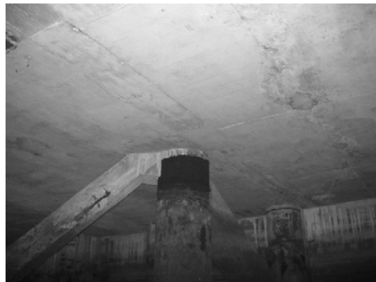
Block 3 Pile 60B
