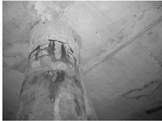
Block 3 Pile 61E-4
