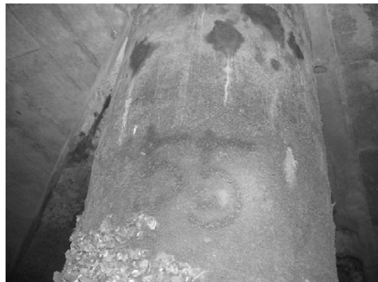
Block 3 Pile 55D-2
