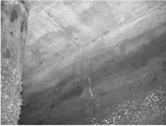
Block 3 Slab nearby Pile 62E
