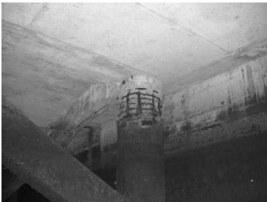
Block 3 Pile 49G
