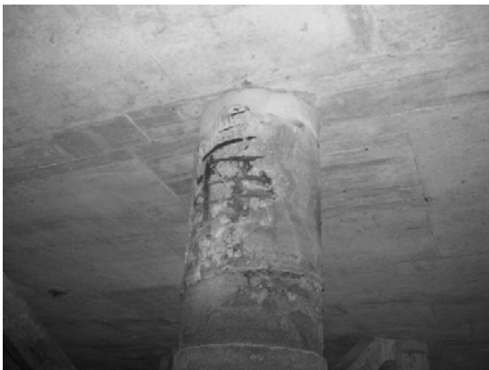
Block 3 Pile 53E-1
