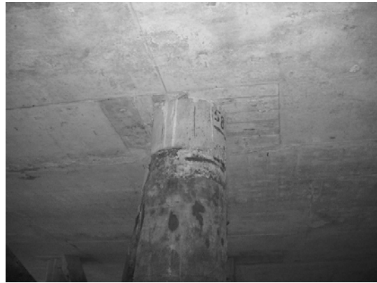
Block 3 Pile 52D
