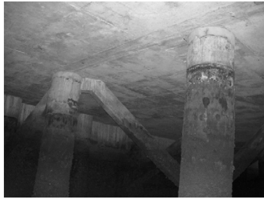
Block 3 Pile 51C-1
