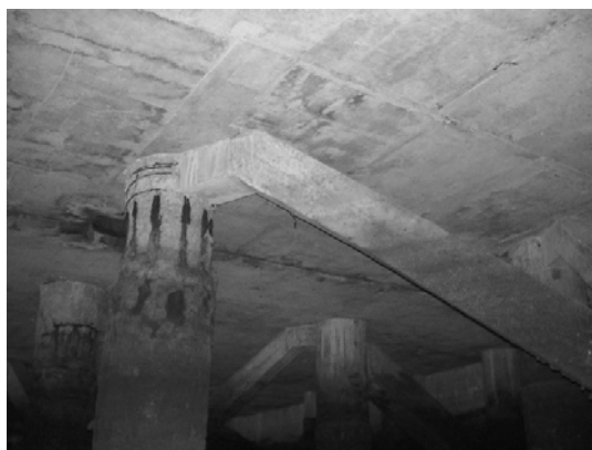
Block 3 Pile 41C
