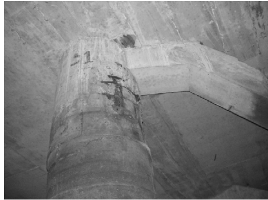
Block 3 Pile 45C-2
