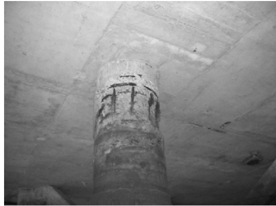
Block 3 Pile 42E-2
