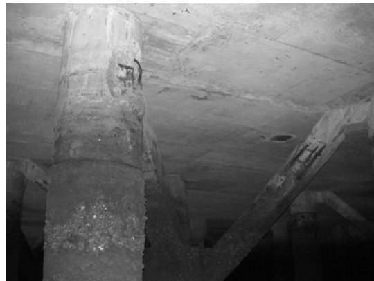
Block 3 Pile 53E-2
