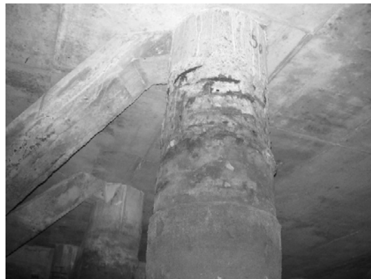
Block 3 Pile 44C
