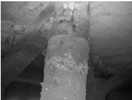
Block 3 Pile 58F
