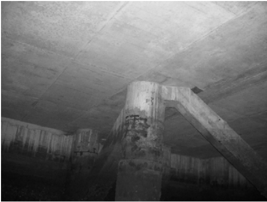
Block 3 Pile 47A ~ 47B
