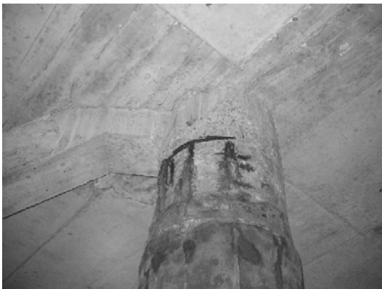
Block 3 Pile 45D-1
