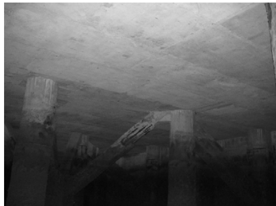
Block 3 Pile 50A ~ 50C
