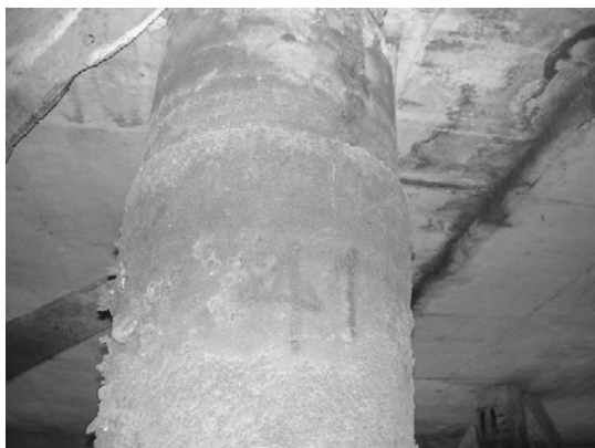
Block 3 Pile 41D-3
