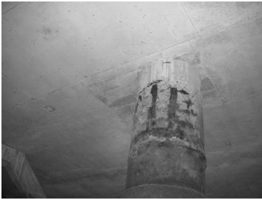
Block 3 Pile 51E-1
