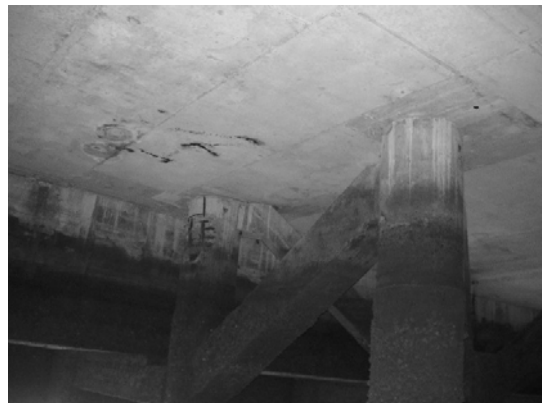
Block 3 Pile 50F ~ 50G
