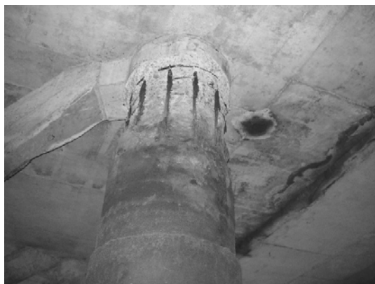
Block 3 Pile 41D-2
