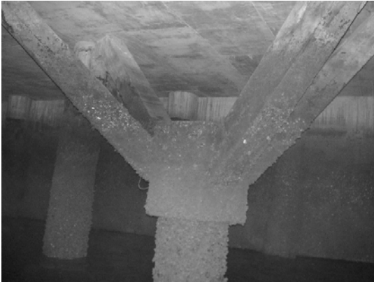
Block 3 Pile 126a
