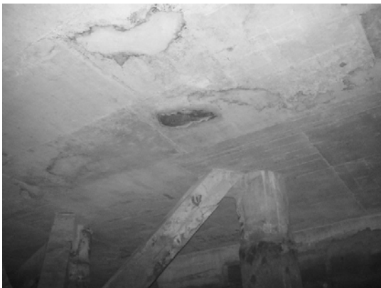
Block 3 Slab nearby Pile 61F
