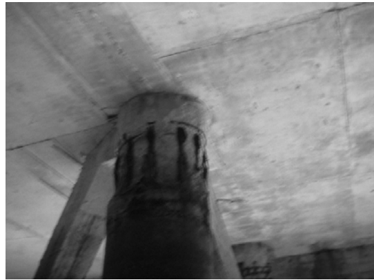
Block 3 Pile 45F-2
