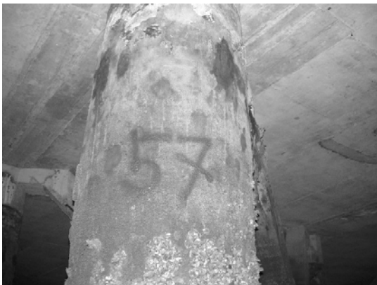
Block 3 Pile 57E-1
