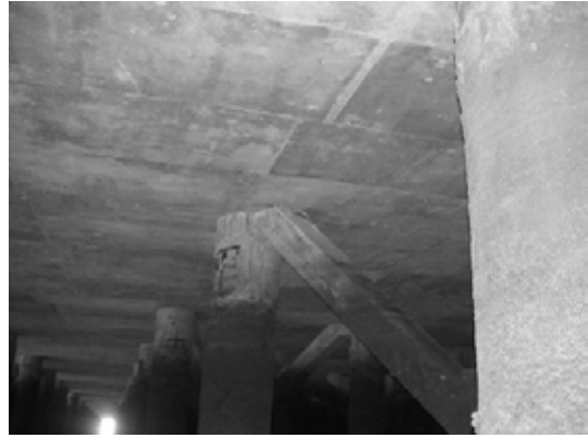
Block 2 Pile 37C
