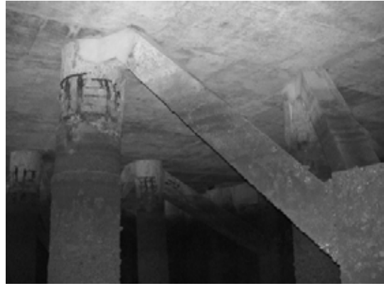
Block 2 Pile 39C
