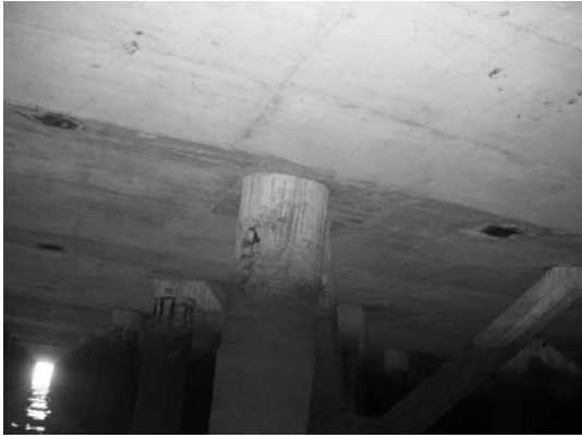
Block 2 Pile 30E-1
