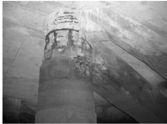
Block 2 Pile 34F-2
