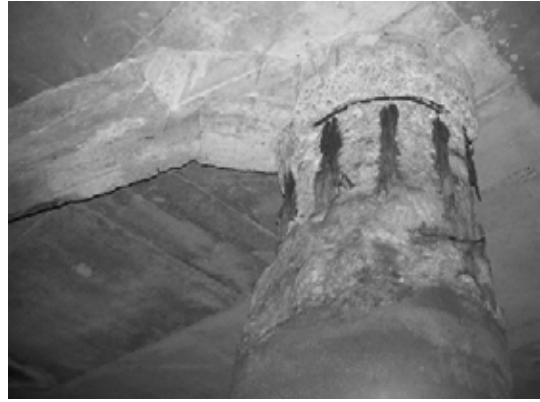
Block 2 Pile 38E-2
