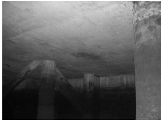
Block 2 Pile 34A ~ 34C
