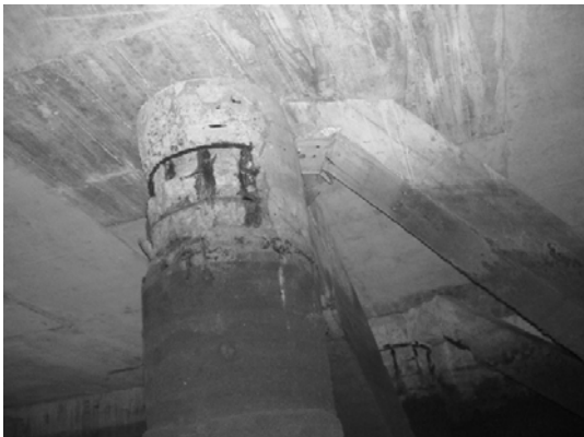
Block 2 Pile 26F
