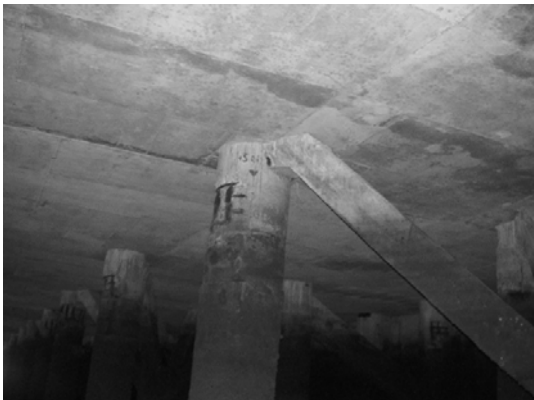
Block 2 Pile 35C-1
