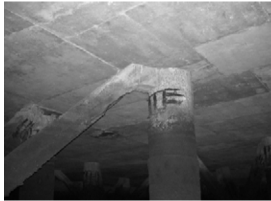
Block 2 Pile 36E-2
