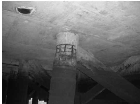
Block 2 Pile 39F
