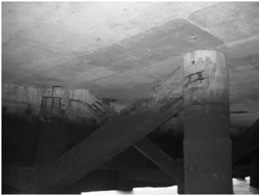
Block 2 Pile 34F-1
