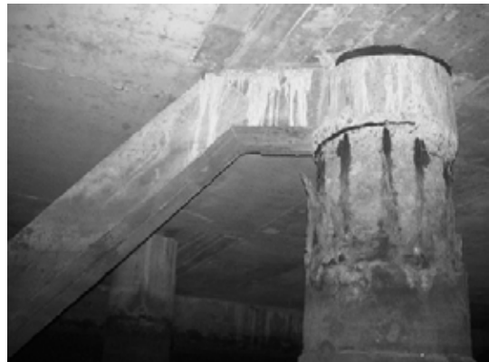
Block 2 Pile 22C
