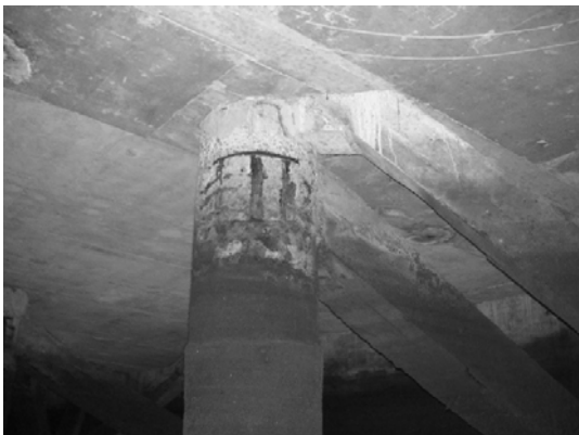
Block 2 Pile 38F-3
