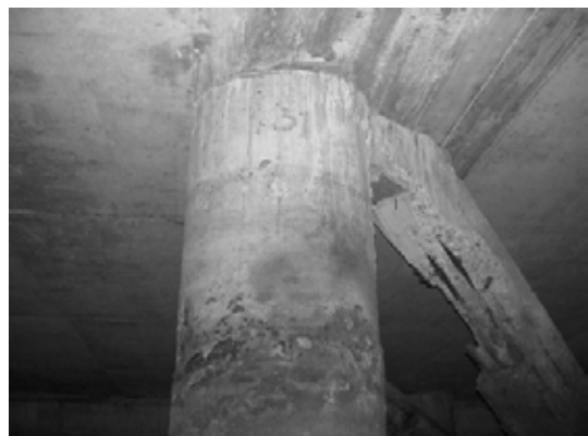
Block 2 Pile 25C-1
