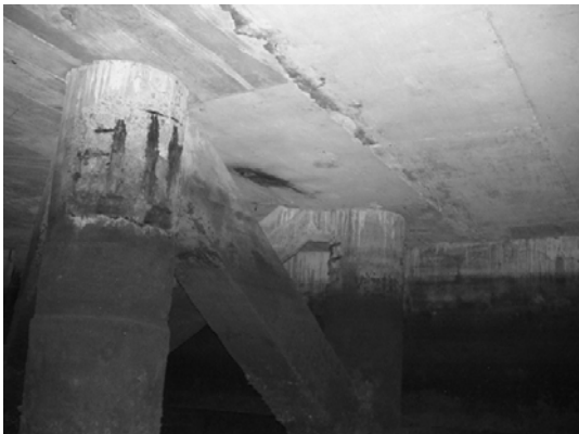
Block 2 Pile 23F ~ 23G
