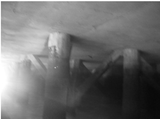
Block 2 Pile 34C
