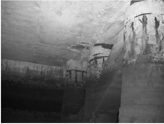
Block 2 Pile 20F
