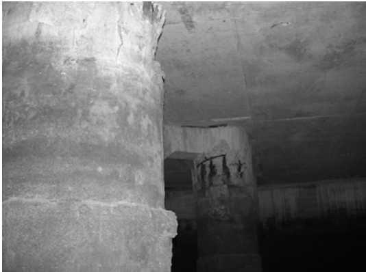
Block 2 Pile 30B
