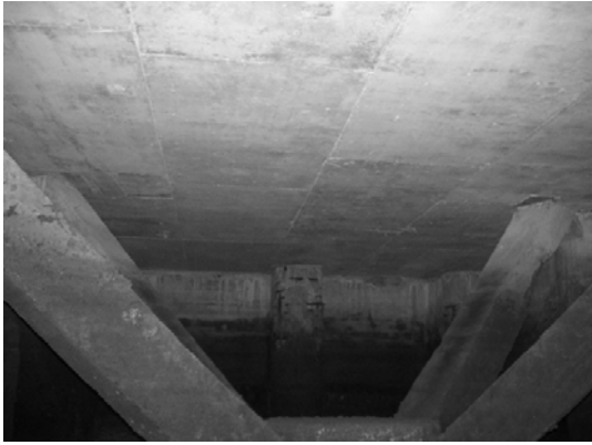
Block 2 Pile 111a
