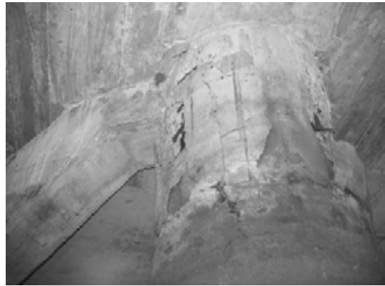
Block 2 Pile 26E
