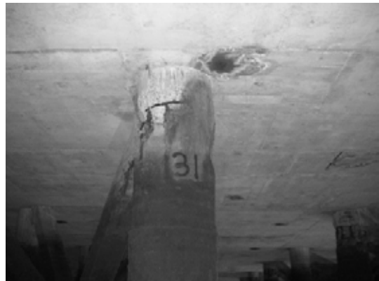
Block 2 Pile 31E-2
