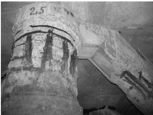
Block 2 Pile 19C
