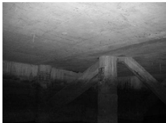
Block 2 Pile 27F ~ 27B
