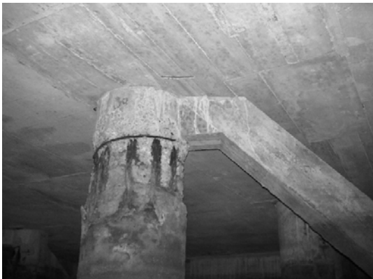
Block 2 Pile 33C-2
