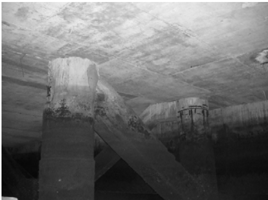
Block 2 Pile 21F ~ 21G
