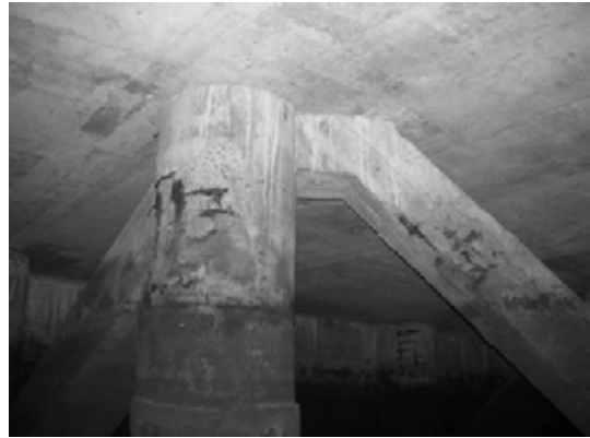
Block 2 Pile 21B
