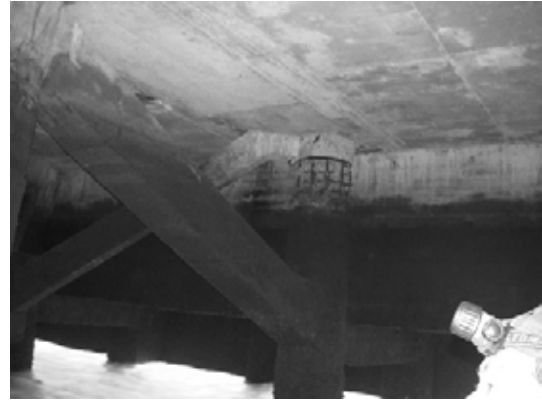
Block 2 Pile 39G
