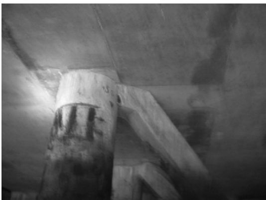
Block 2 Pile 35C-3
