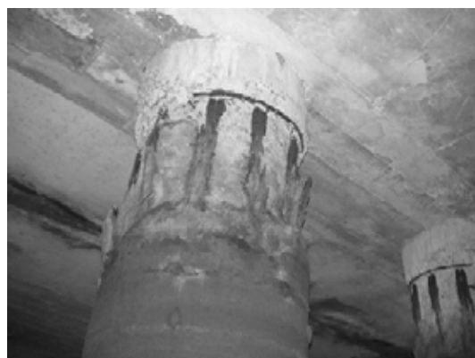
Block 2 Pile 18E-2
