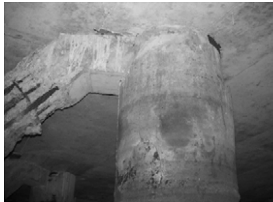
Block 2 Pile 20C-2
