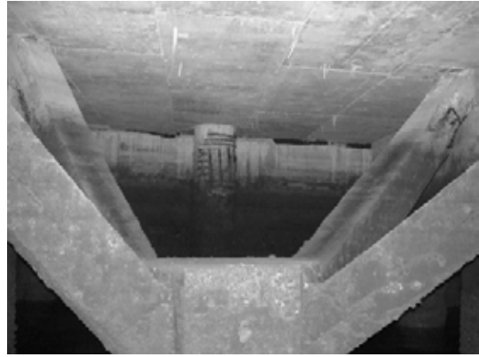
Block 2 Pile 113a
