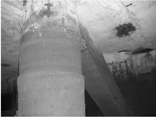
Block 2 Brace bet. Pile 29F & 29G
