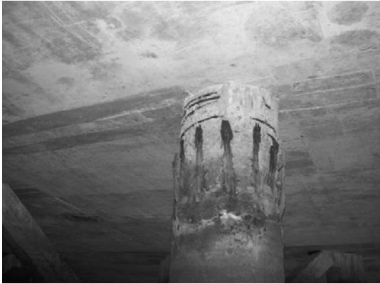
Block 2 Pile 21E-1
