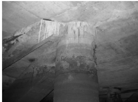
Block 2 Pile 19F-2
