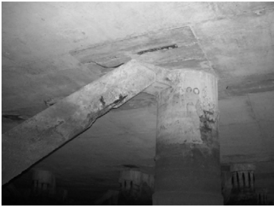
Block 2 Pile 28E-1
