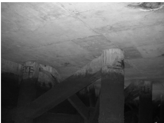
Block 2 Pile 36F ~ 36G-2
