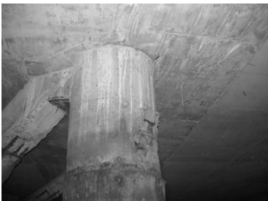
Block 2 Pile 27C-4
