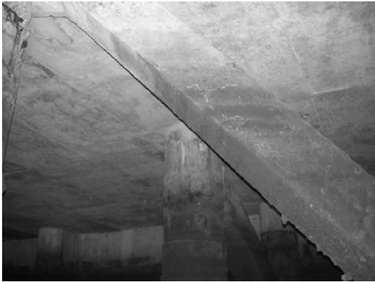
Block 2 Pile 38B
