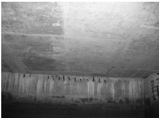
Block 2 Wall bet. Pile 18A & 19A
