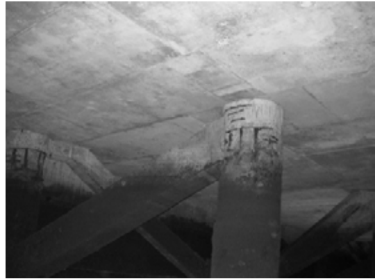
Block 2 Pile 38F-2
