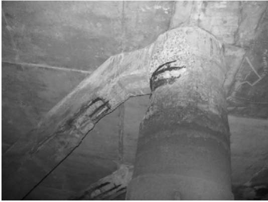
Block 2 Pile 38E-1
