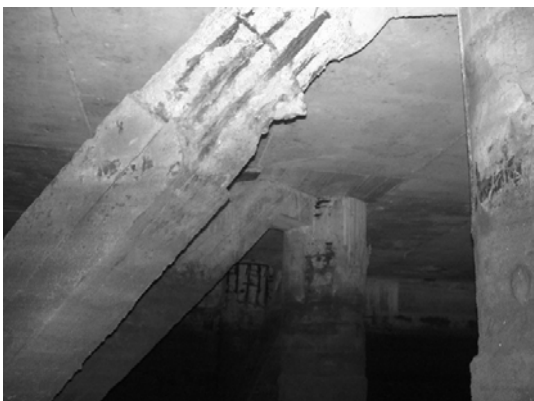
Block 2 Beam bet. Pile 20C & 109a
