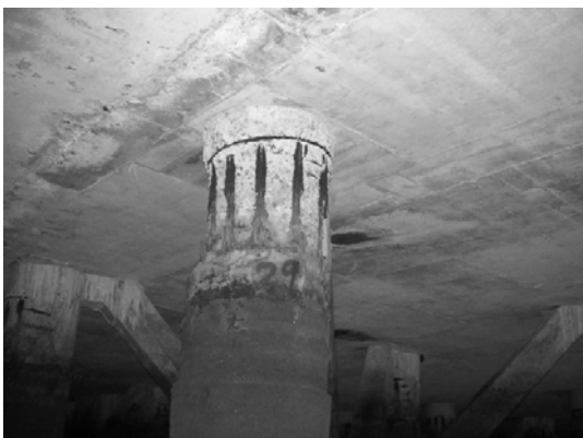
Block 2 Pile 29E-2
