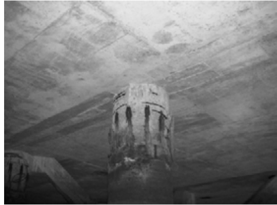
Block 2 Pile 21E-2
