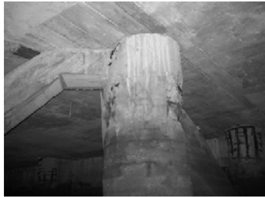
Block 2 Pile 20B
