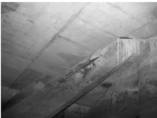
Block 2 Beam bet. Pile 19F & 109c
