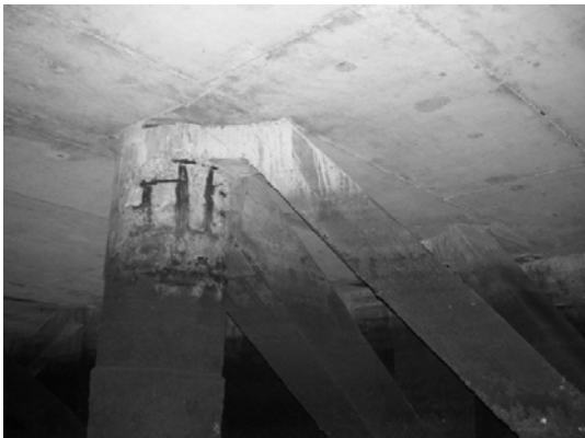
Block 2 Pile 22F
