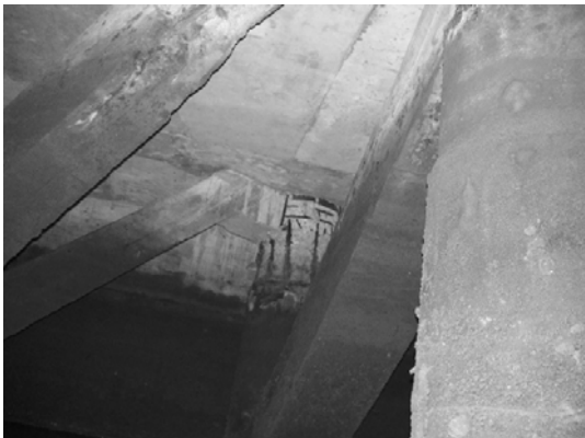
Block 2 Pile 35F-4
