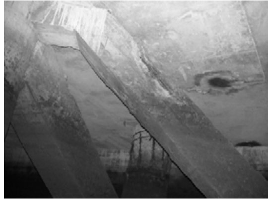
Block 2 Beam bet. Pile 20F & 109c
