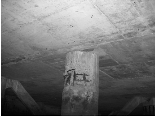
Block 2 Pile 23C-2
