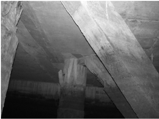
Block 2 Pile 27B
