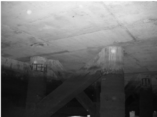
Block 2 Pile 24F ~ 24G
