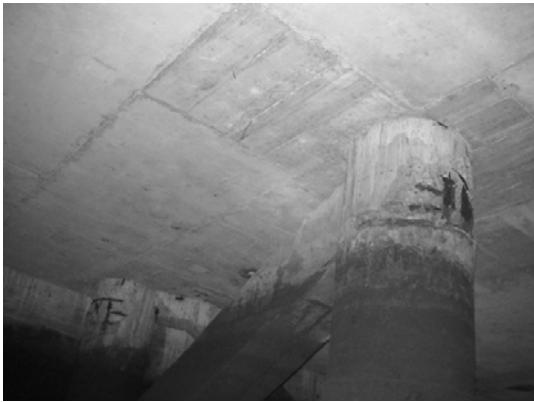
Block 2 Pile 35F-2
