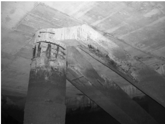
Block 2 Pile 36F
