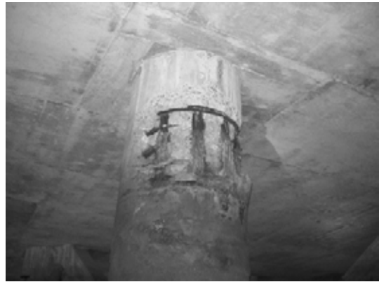
Block 2 Pile 24E-2
