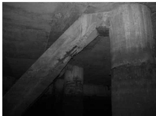
Block 2 Pile 26C
