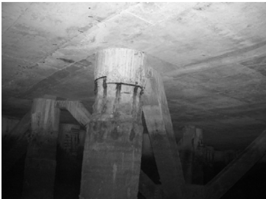
Block 2 Pile 27C-2
