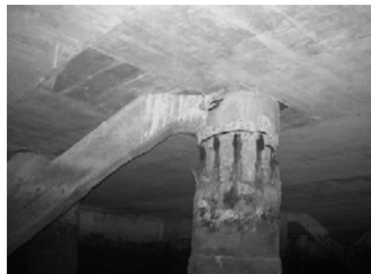
Block 2 Pile 24C
