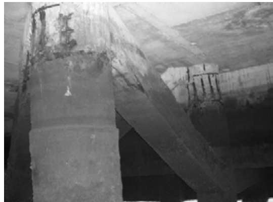
Block 2 Pile 25F ~ 25G
