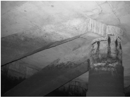
Block 2 Pile 33F-2
