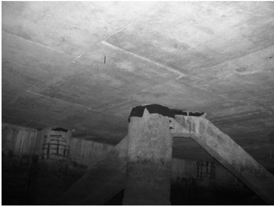
Block 2 Pile 19B-1
