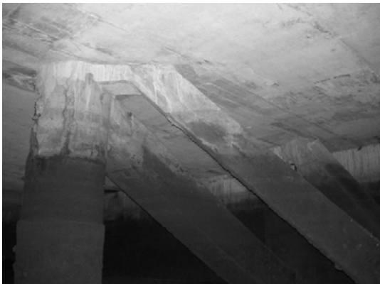
Block 2 Pile 28F
