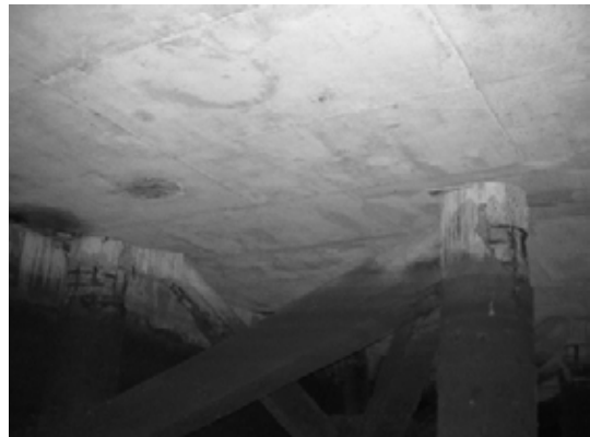
Block 2 Pile 36F ~ 36G-1
