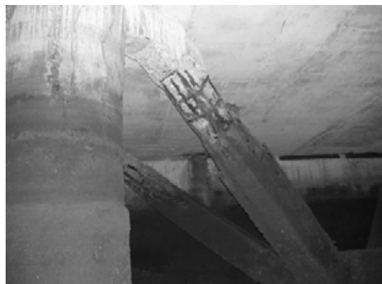
Block 2 Beam bet. Pile 32F & 115c
