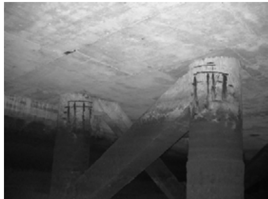
Block 2 Pile 22F ~ 22G
