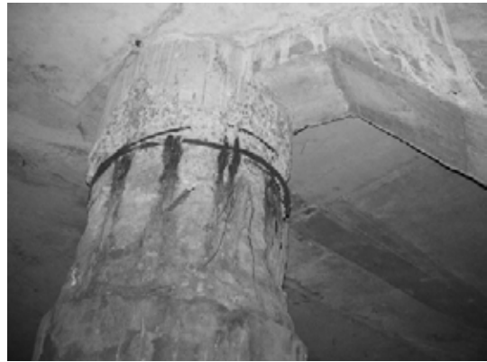
Block 2 Pile 27C-1
