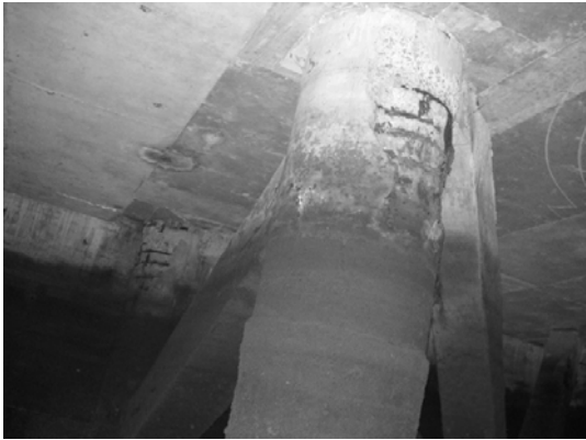
Block 2 Pile 40B
