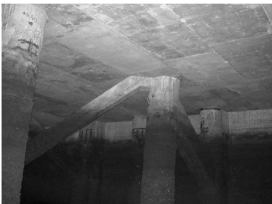
Block 2 Pile 36A ~ 36C
