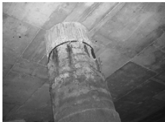
Block 2 Pile 36C
