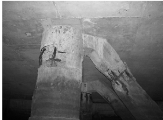
Block 2 Pile 30C
