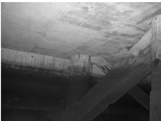
Block 2 Pile 26F ~ 26G-2
