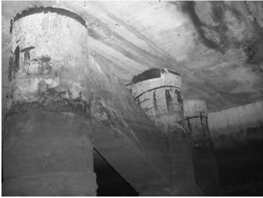
Block 2 Pile 18F ~ 18d
