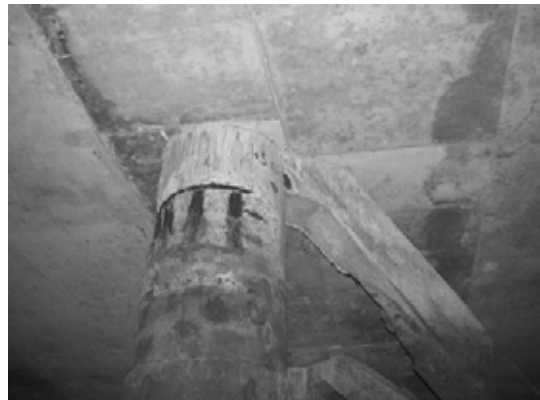
Block 2 Pile 35C-2
