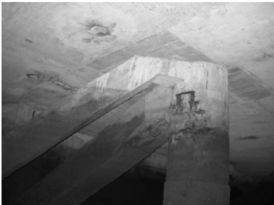
Block 2 Pile 27F
