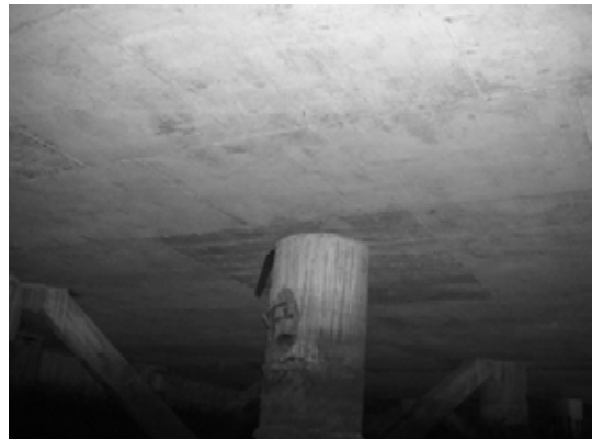
Block 2 Pile 27C-3
