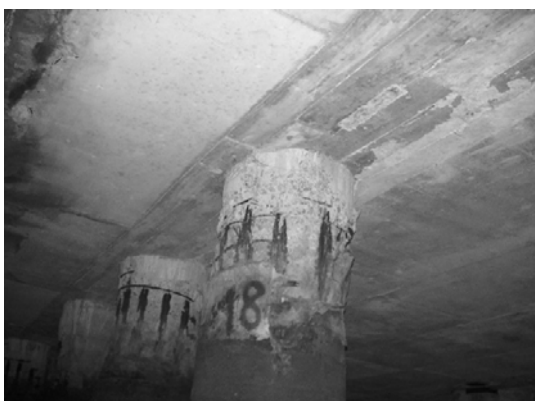
Block 2 Pile 18E-1
