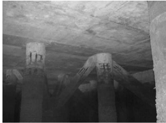
Block 2 Pile 38B ~ 38C
