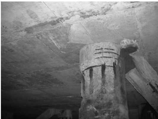
Block 2 Pile 21C
