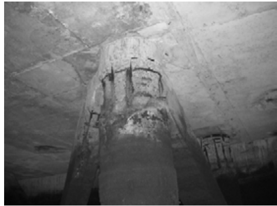
Block 2 Pile 35F-3
