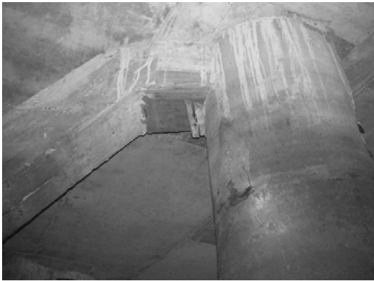
Block 2 Pile 24E-1
