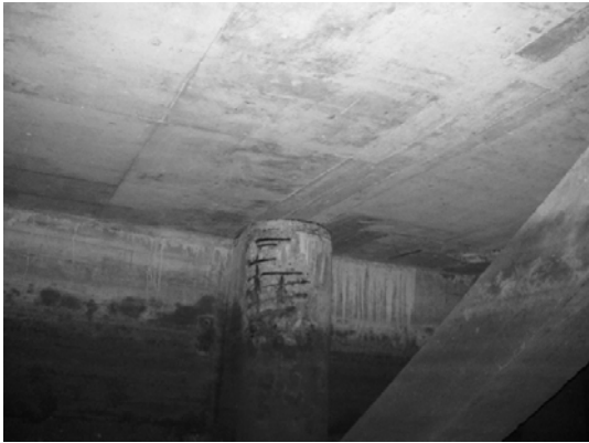
Block 2 Pile 21A
