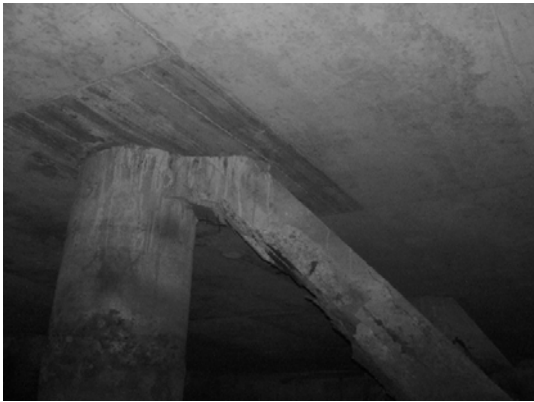
Block 2 Pile 25C-2
