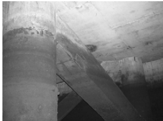
Block 2 Pile 35F ~ 35G
