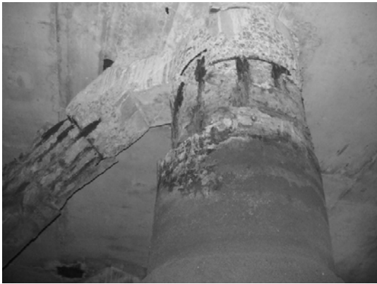
Block 2 Pile 36E-1
