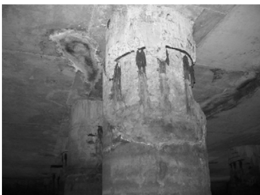
Block 2 Pile 18A
