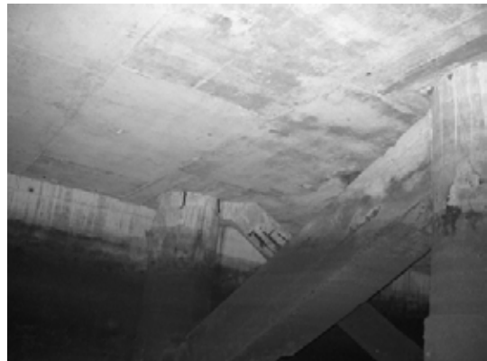
Block 2 Pile 26F ~ 26G-1
