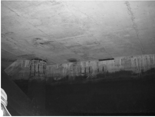
Block 2 Pile 37G-2
