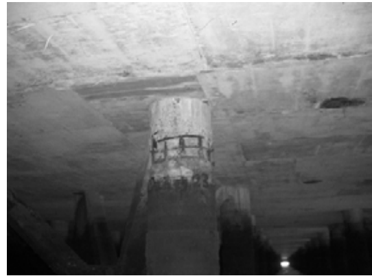
Block 2 Pile 23E-4
