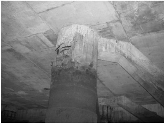
Block 2 Pile 38F-1
