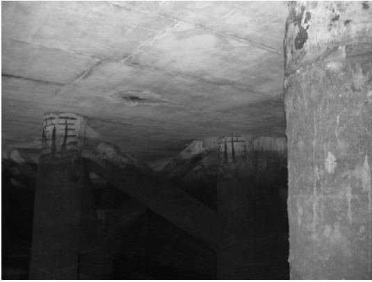
Pile 12D ~ Pile 12E-1
