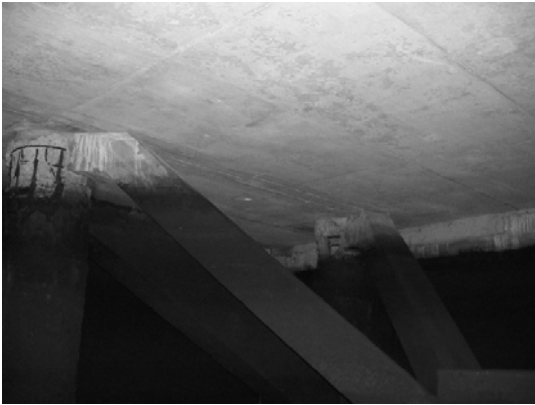
Pile 25D ~ Pile 25D
