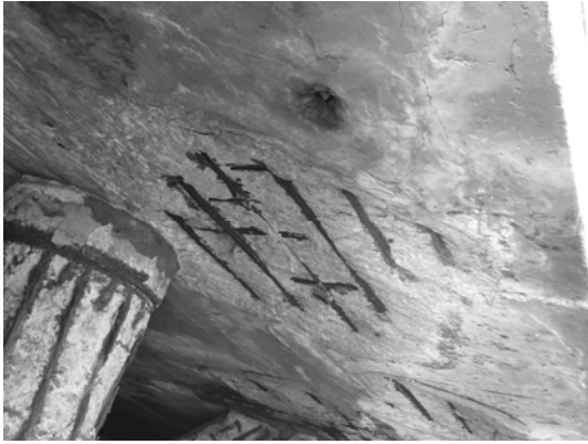
Slab nearby Pile 1B
