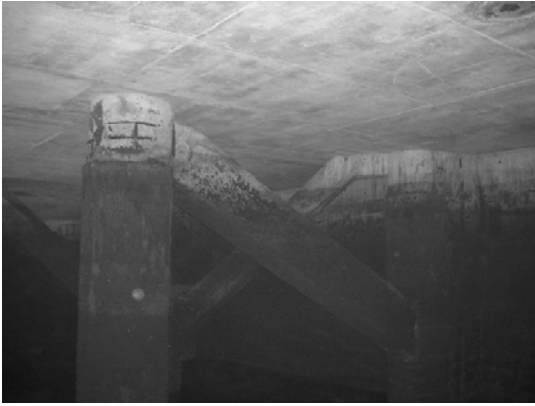
Pile 8D ~ Pile E
