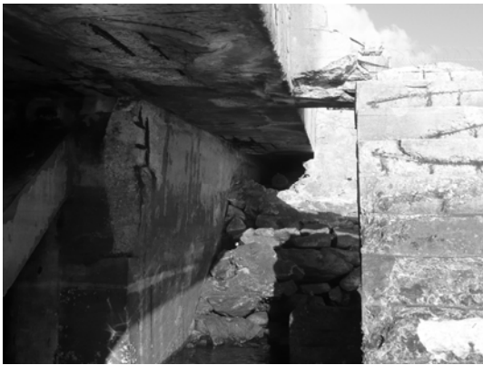
Wall and Slab nearby Pile 1C
