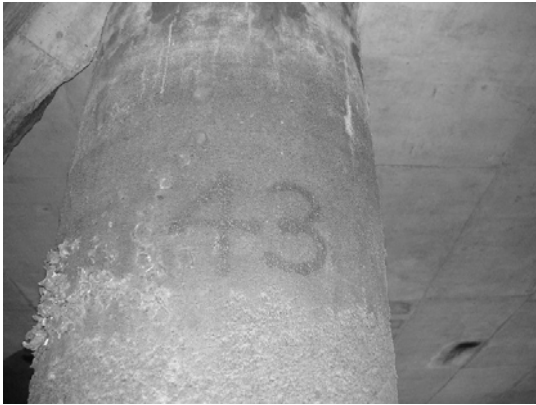
Block 3 Pile 43D-1
