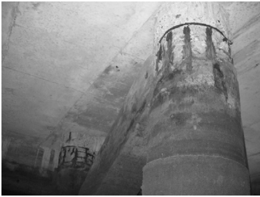
Block 3 Pile 46F ~ 46G-1
