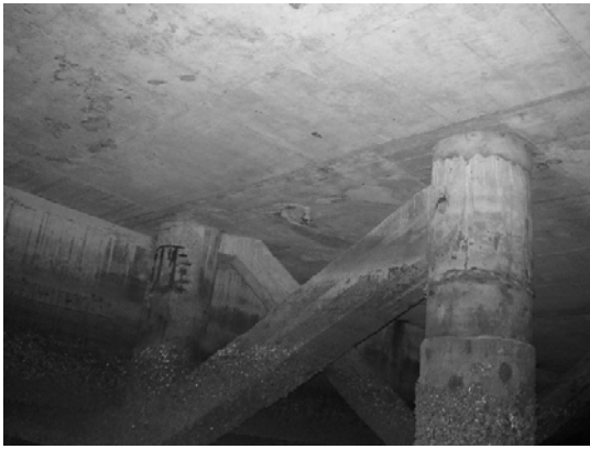
Block 3 Pile 60F ~ 60G-1
