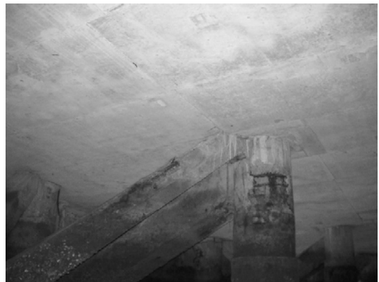
Block 3 Pile 51F-4
