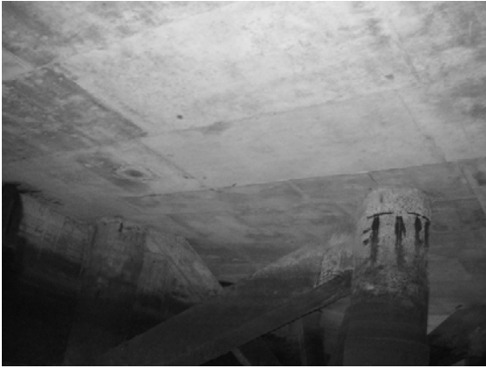
Block 3 Pile 44F
