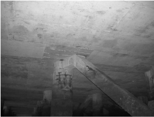
Block 3 Pile 45C-1
