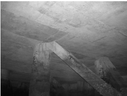
Block 3 Pile 49C
