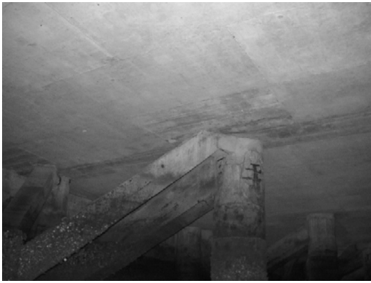
Block 3 Pile 57F
