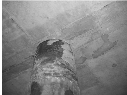
Block 3 Pile 61C
