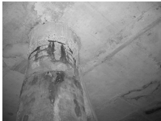
Block 3 Pile 61E-4
