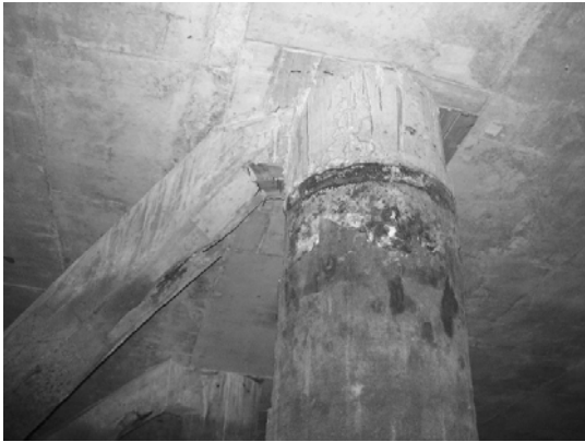
Block 3 Pile 51C-2
