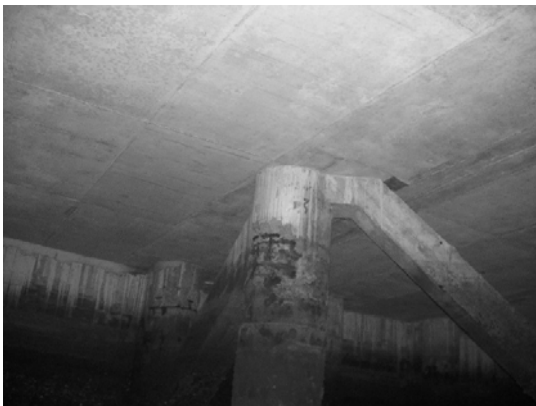
Block 3 Pile 47A ~ 47B
