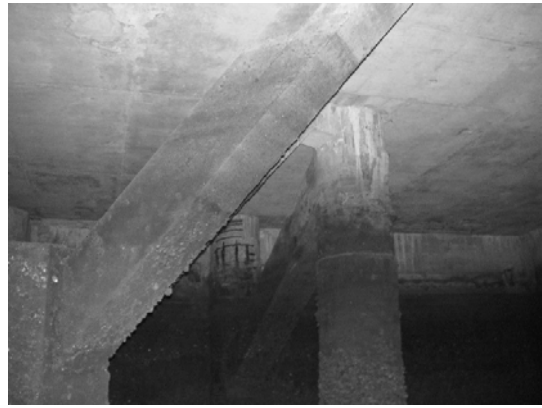
Block 3 Pile 42A ~ 42B-3
