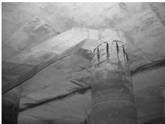
Block 3 Pile 41D-1
