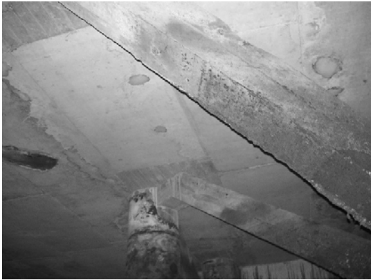
Block 3 Pile 61B
