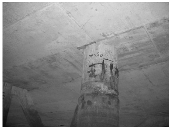
Block 3 Pile 47D-2
