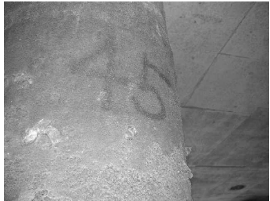
Block 3 Pile 45D-2
