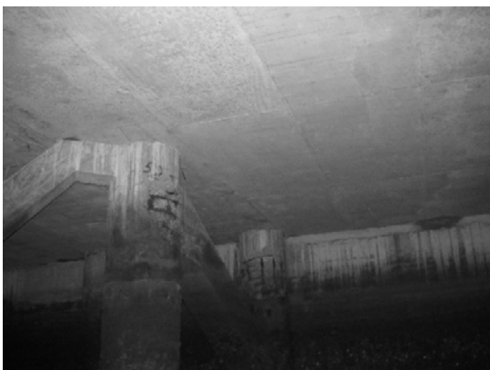
Block 3 Pile 46A ~ 46B
