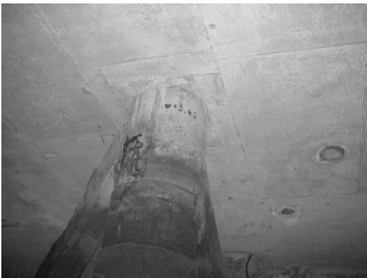
Block 3 Pile 51F-3
