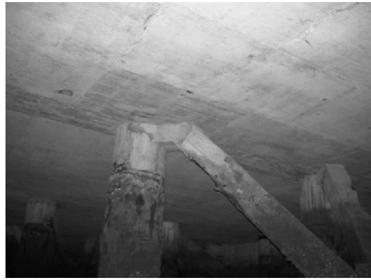
Block 3 Pile 57C-1
