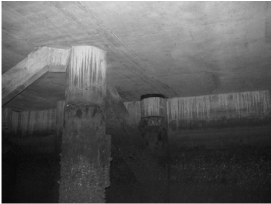
Block 3 Pile 56B
