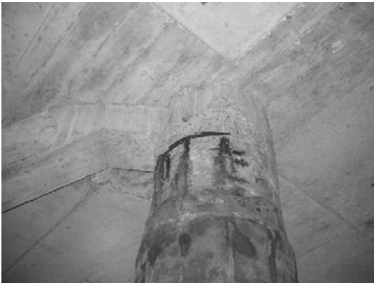
Block 3 Pile 45D-1
