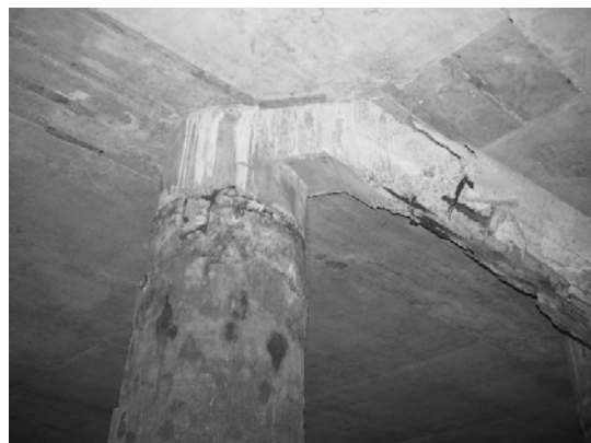
Block 3 Pile 60D
