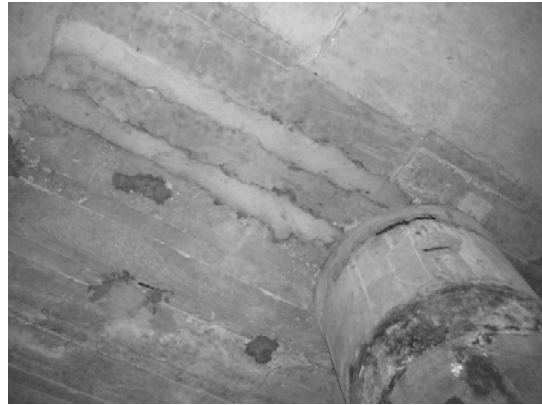
Block 3 Slab bet. Pile 60E & 61E-3
