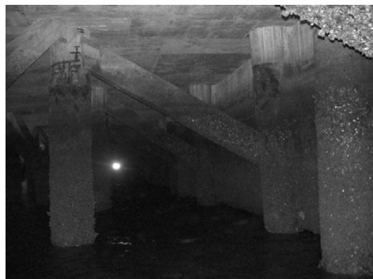
Block 3 Pile 53A ~ 53B
