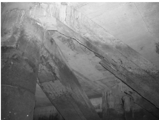
Block 3 Pile 52F
