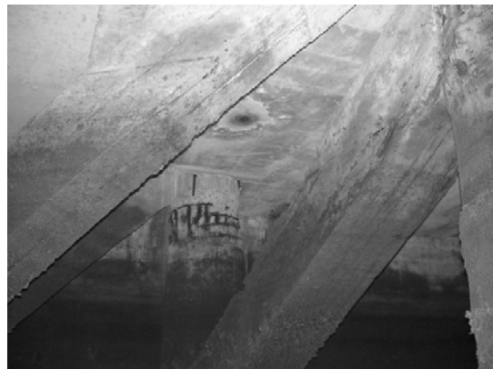
Block 3 Pile 45G
