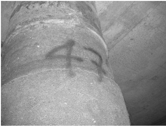
Block 3 Pile 47D-3
