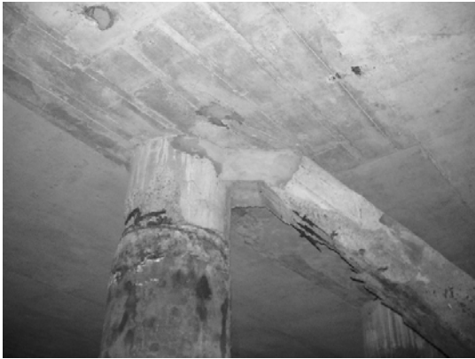
Block 3 Pile 57C-2
