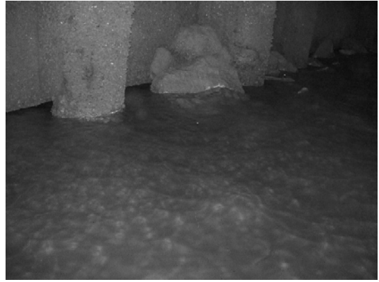
Block 3 Pile 127A
