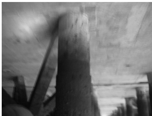
Block 3 Pile 41E-1
