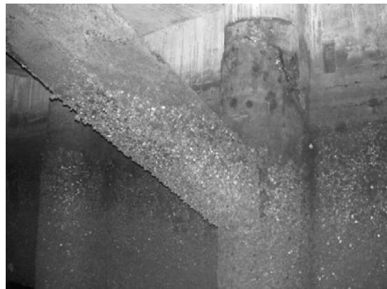
Block 3 Pile 54A
