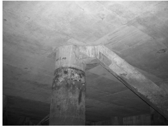
Block 3 Pile 51C-3
