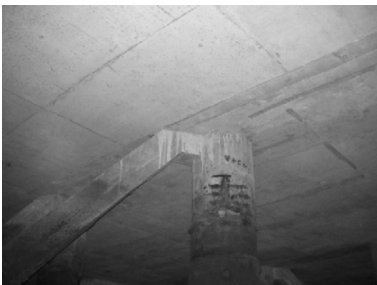
Block 3 Pile 48C-2
