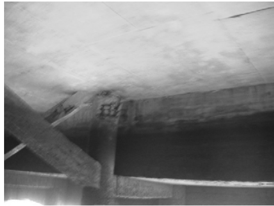
Block 3 Pile 43G
