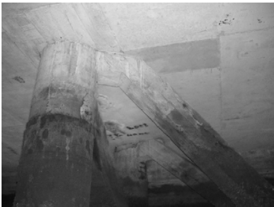
Block 3 Pile 50F
