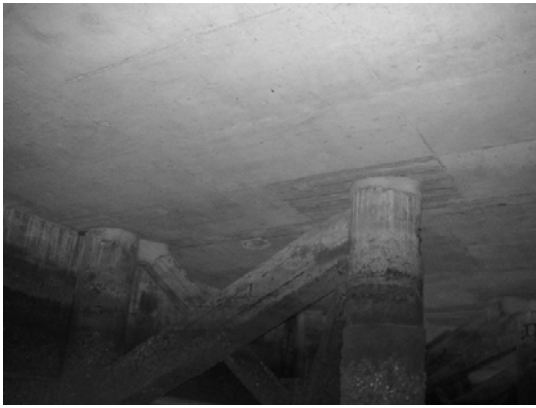
Block 3 Pile 56F ~ 53G
