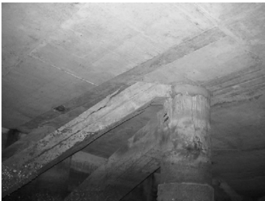
Block 3 Pile 59F
