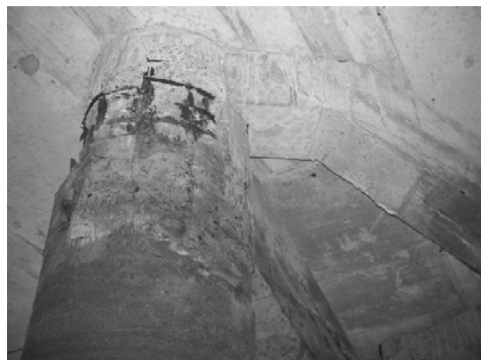
Block 3 Pile 46F
