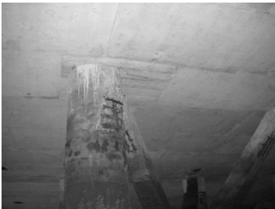
Block 3 Pile 52E-1
