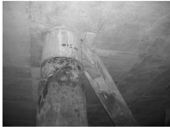
Block 3 Pile 50C
