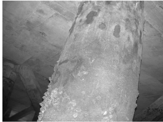
Block 3 Pile 57D
