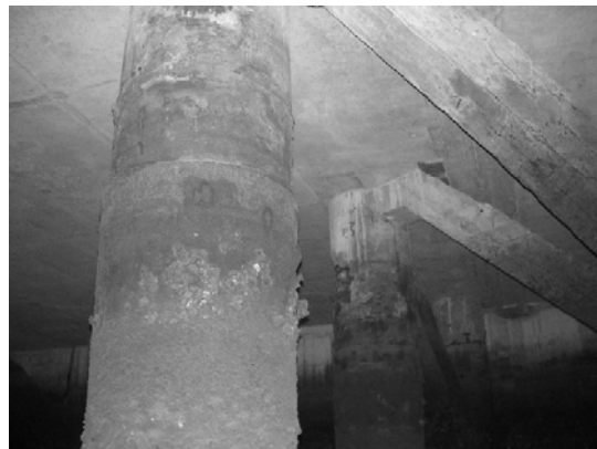
Block 3 Pile 47B
