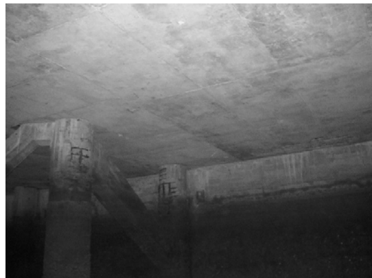
Block 3 Pile 42A ~ 42B-1
