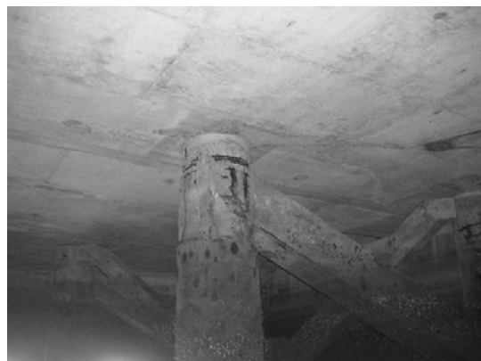
Block 3 Pile 61F
