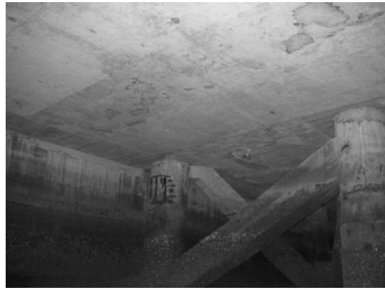
Block 3 Pile 60F ~ 60G-2
