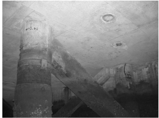
Block 3 Pile 51F-2
