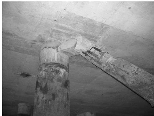
Block 3 Pile 57E-2
