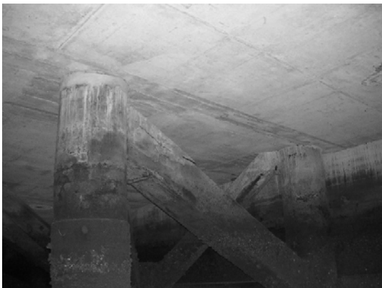
Block 3 Pile 53F ~ 53G
