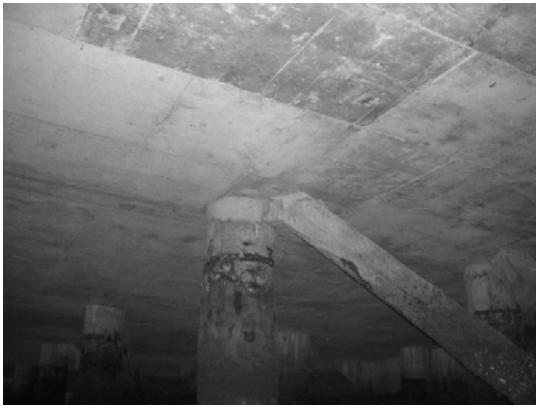
Block 3 Pile 53C
