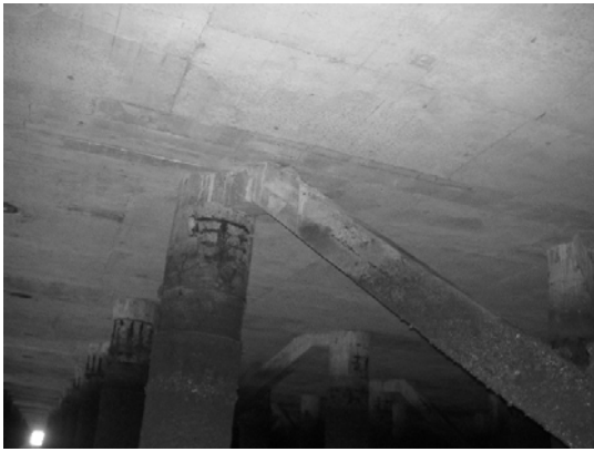
Block 3 Pile 49E-1
