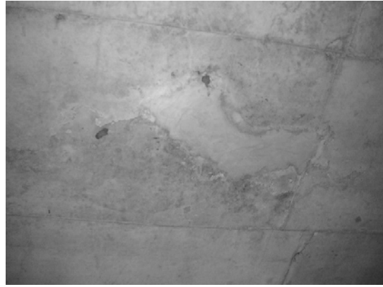
Block 3 Slab bet. Pile 60E & 61E-1
