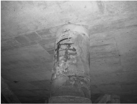
Block 3 Pile 53E-1
