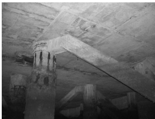
Block 3 Pile 41C
