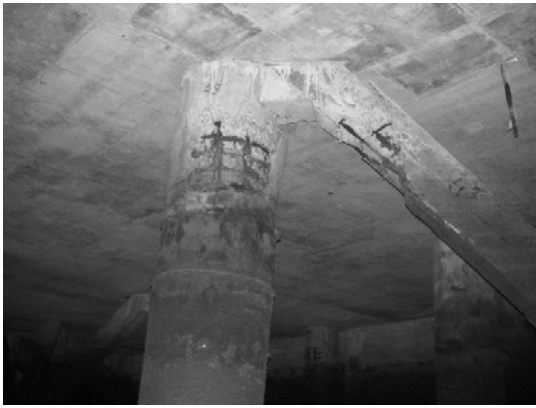
Block 3 Pile 43C-1
