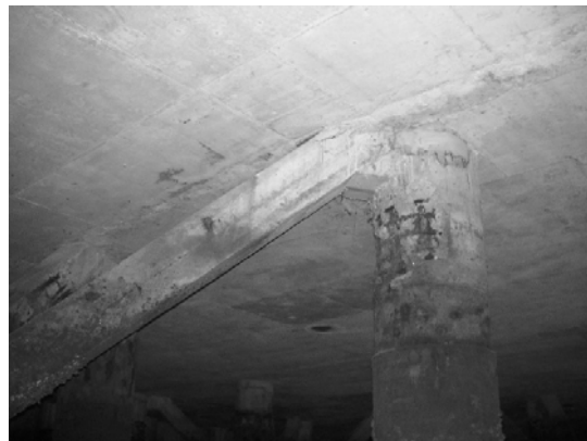
Block 3 Pile 52E-2
