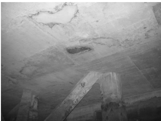
Block 3 Slab nearby Pile 61F
