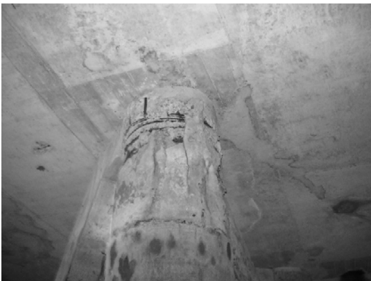
Block 3 Slab bet. Pile 60E & 61E-4
