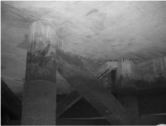
Block 3 Pile 51F-1
