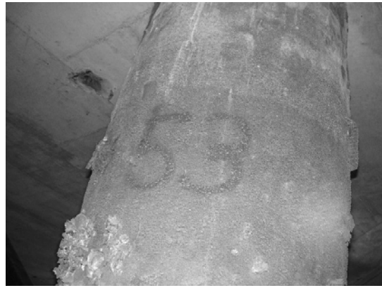
Block 3 Pile 53D
