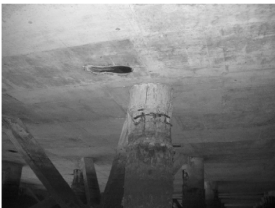
Block 3 Pile 44D
