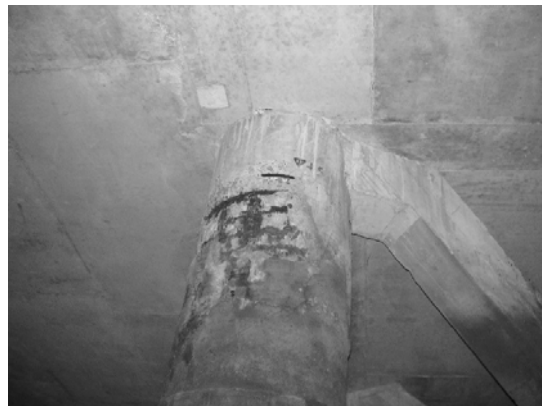
Block 3 Pile 48C-1
