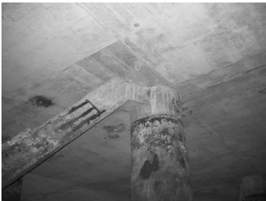
Block 3 Pile 61D-1
