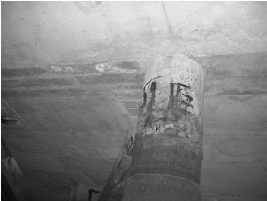
Block 3 Pile 50E-1
