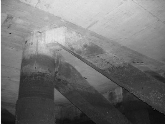
Block 3 Pile 48F
