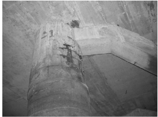
Block 3 Pile 45C-2
