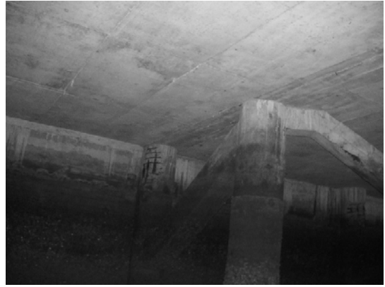
Block 3 Pile 45A ~ 45B
