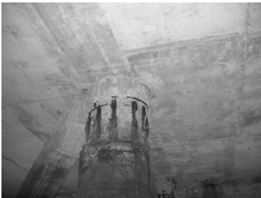
Block 3 Pile 45F-3
