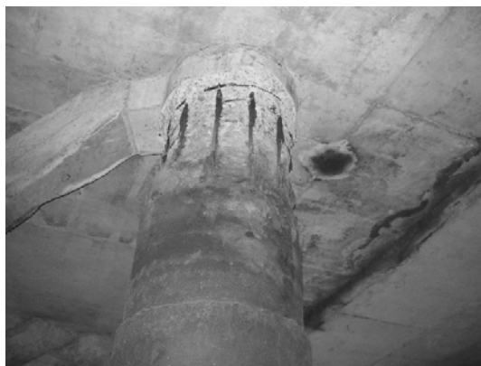
Block 3 Pile 41D-2
