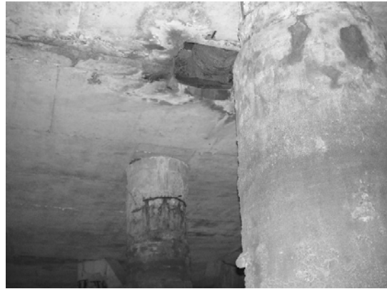
Block 3 Pile 43D-2
