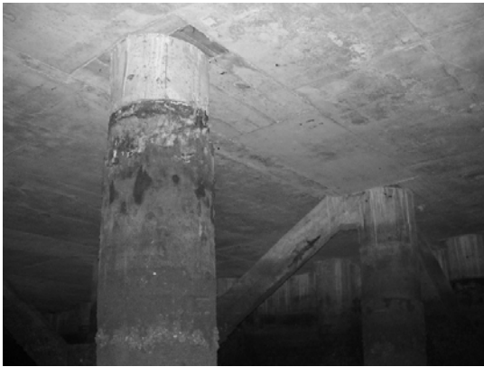
Block 3 Pile 52C
