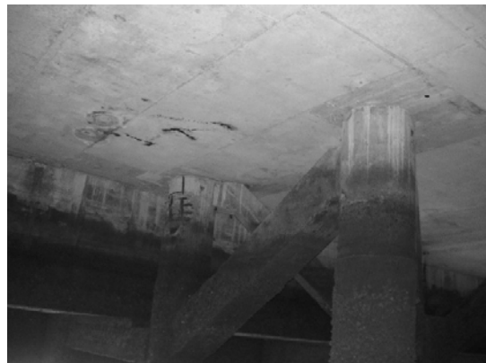
Block 3 Pile 50F ~ 50G
