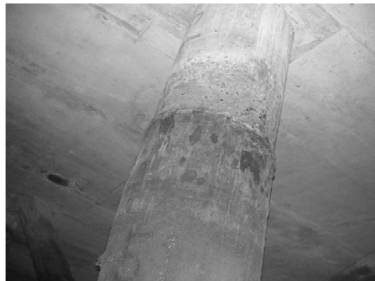
Block 3 Pile 51D-2
