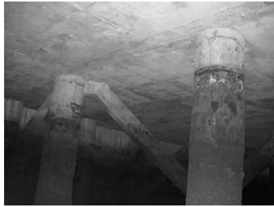
Block 3 Pile 51C-1
