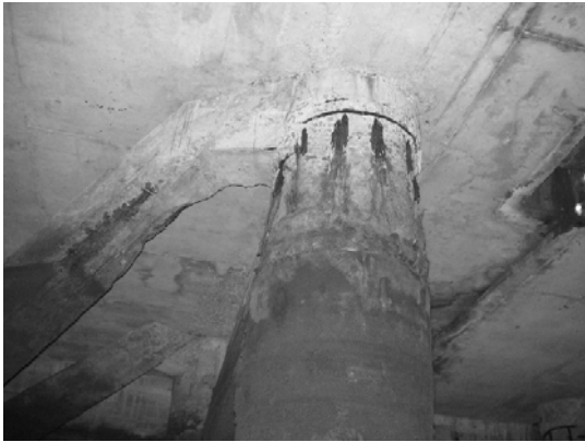
Block 3 Pile 41F
