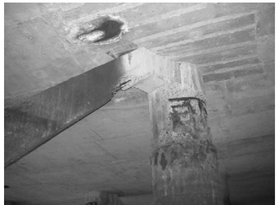
Block 3 Pile 49D
