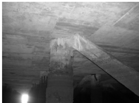
Block 2 Pile 23E-2
