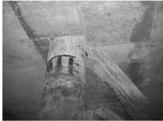
Block 2 Pile 35C-2
