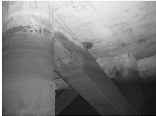
Block 2 Pile 35F ~ 35G
