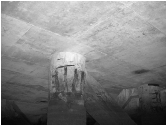
Block 2 Pile 19F-1
