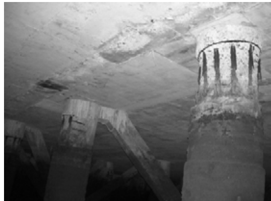
Block 2 Pile 29E-1
