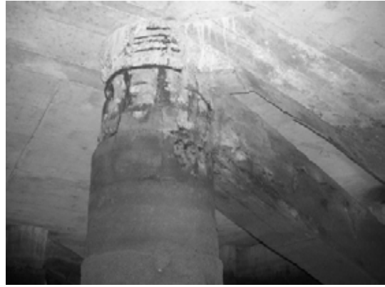
Block 2 Pile 34F-2
