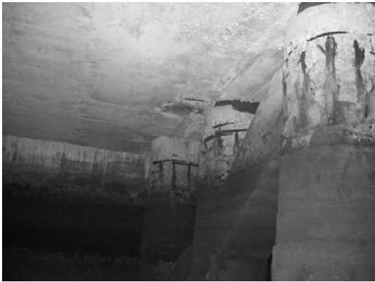
Block 2 Pile 20F
