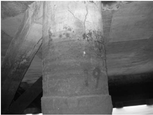
Block 2 Pile 19D-2
