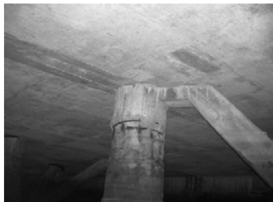
Block 2 Pile 22D-2
