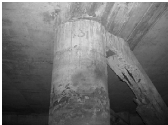
Block 2 Pile 25C-1
