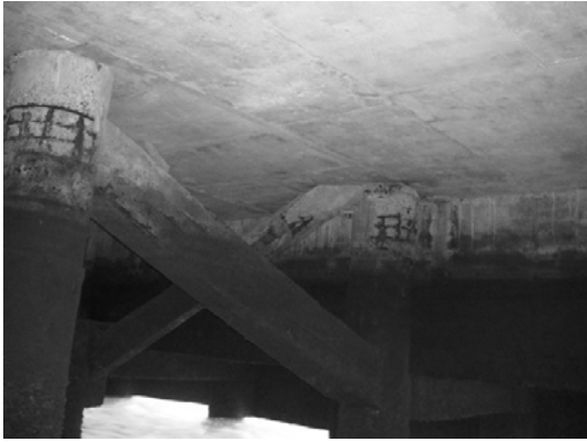
Block 2 Brace bet. Pile 39F & 39G
