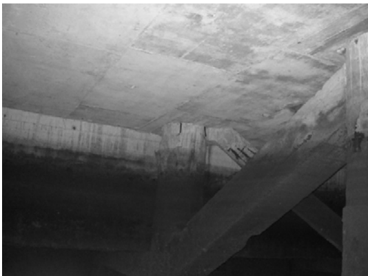
Block 2 Pile 26F ~ 26G-2
