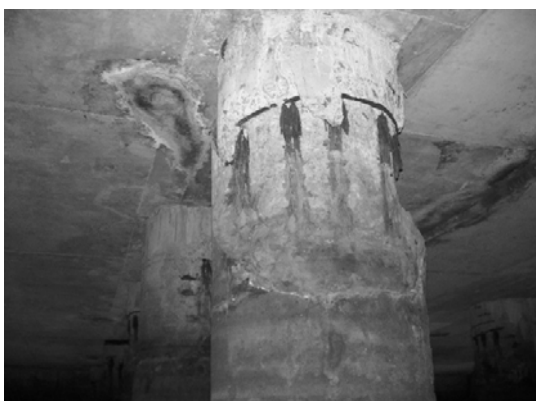
Block 2 Pile 18A
