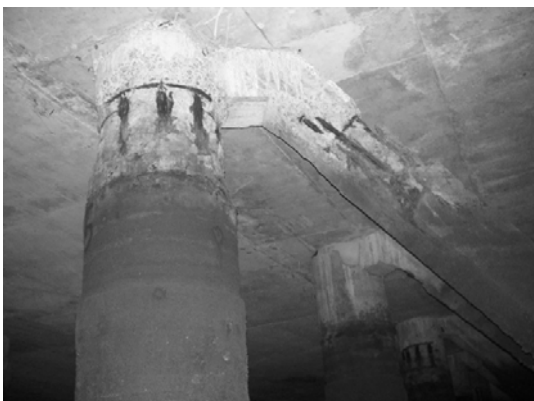
Block 2 Pile 35E-3
