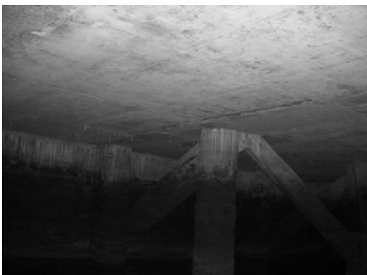
Block 2 Pile 23A ~ 23B
