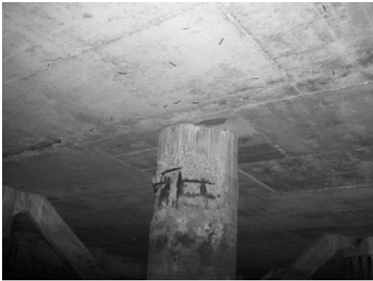
Block 2 Pile 23C-2
