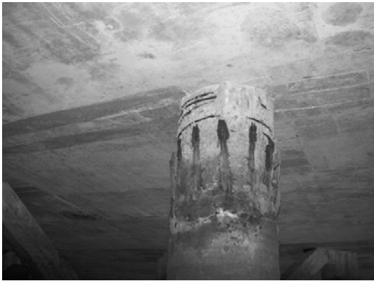
Block 2 Pile 21E-1
