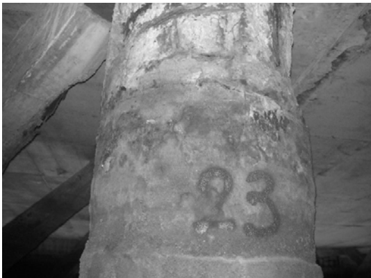
Block 2 Pile 23D-2
