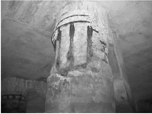
Block 2 Pile 26D
