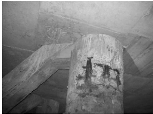
Block 2 Pile 33C-1
