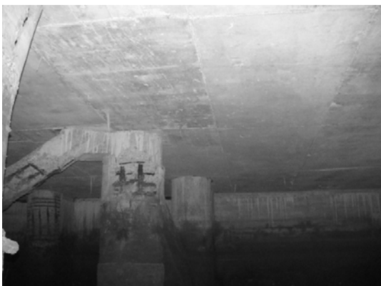
Block 2 Pile 28A ~ 28B
