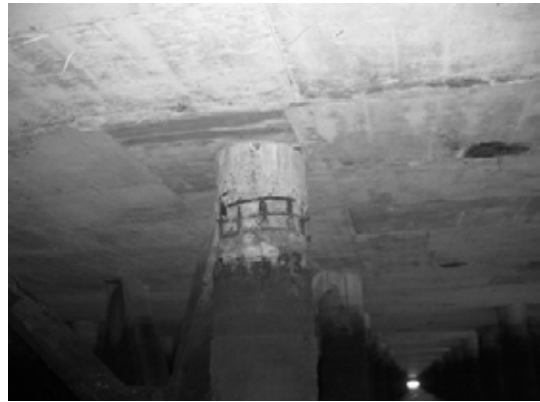
Block 2 Pile 23E-4
