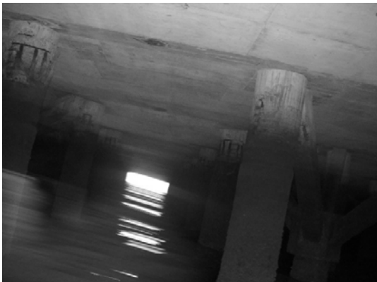
Block 2 Pile 30E-3
