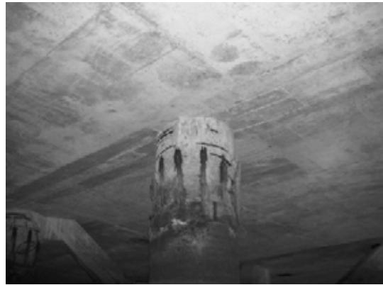
Block 2 Pile 21E-2
