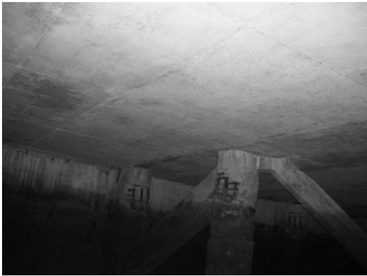
Block 2 Pile 33A ~ 33B
