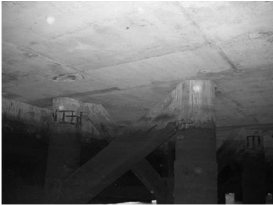
Block 2 Pile 24F ~ 24G
