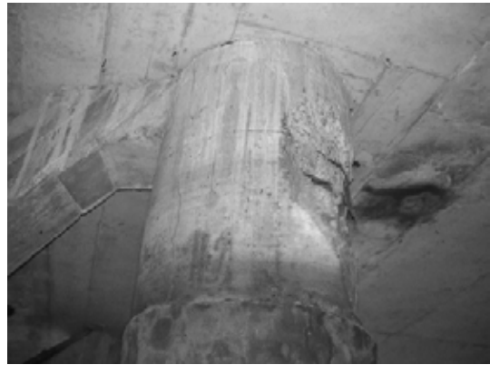
Block 2 Pile 29D-1
