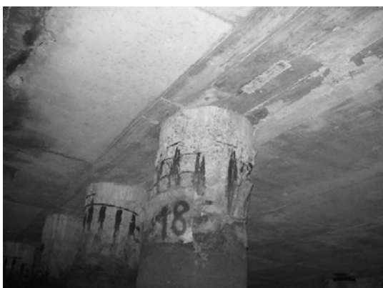
Block 2 Pile 18E-1
