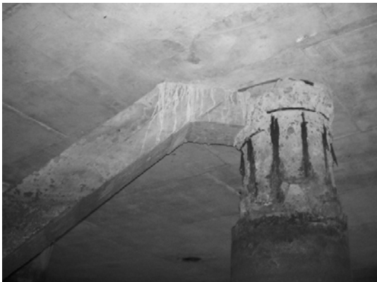
Block 2 Pile 31E-1
