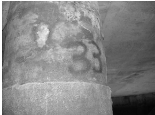
Block 2 Pile 33D
