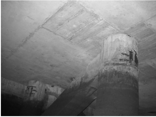
Block 2 Pile 35F-2
