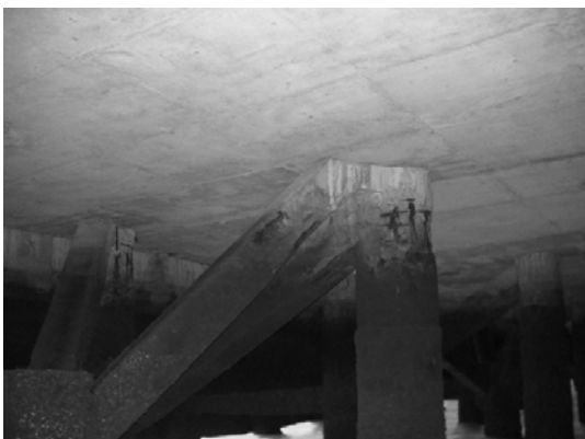
Block 2 Beam bet. Pile 25F & 112c
