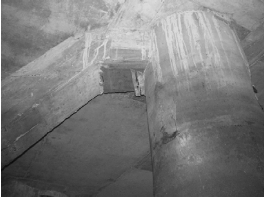
Block 2 Pile 24E-1
