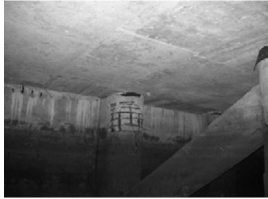
Block 2 Pile 19A
