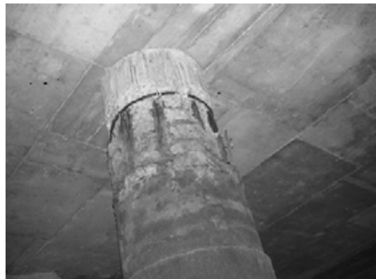
Block 2 Pile 36C
