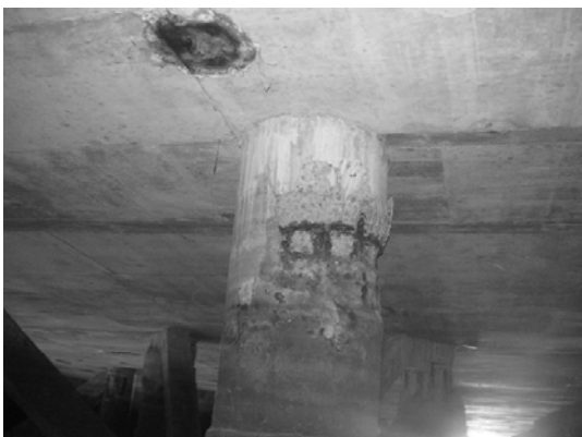
Block 2 Pile 22D-1
