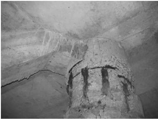
Block 2 Pile 31D-2
