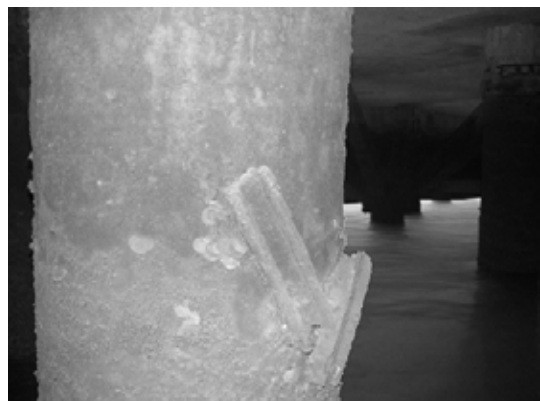
Block 2 Pile 27D-1
