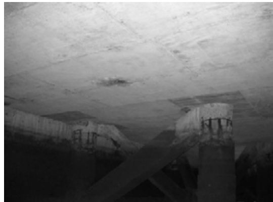
Block 2 Brace bet. Pile 28F & 28G
