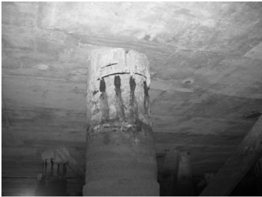
Block 2 Pile 22E-1
