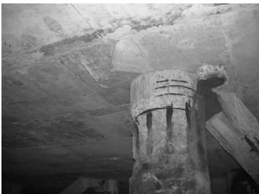
Block 2 Pile 21C
