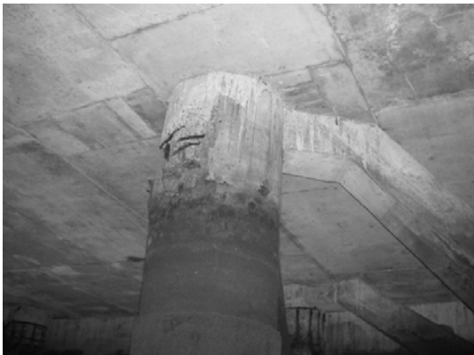
Block 2 Pile 38F-1
