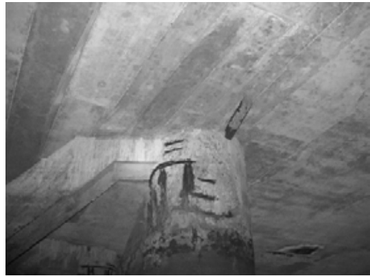
Block 2 Pile 22E-2
