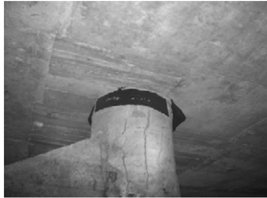
Block 2 Pile 19B-2
