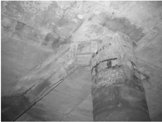
Block 2 Pile 39D-1
