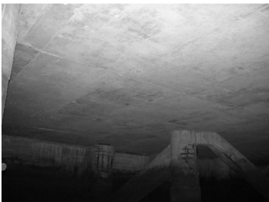
Block 2 Pile 29A ~ 29B
