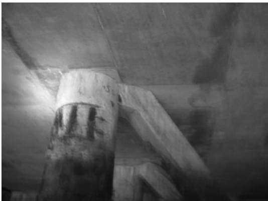
Block 2 Pile 35C-3
