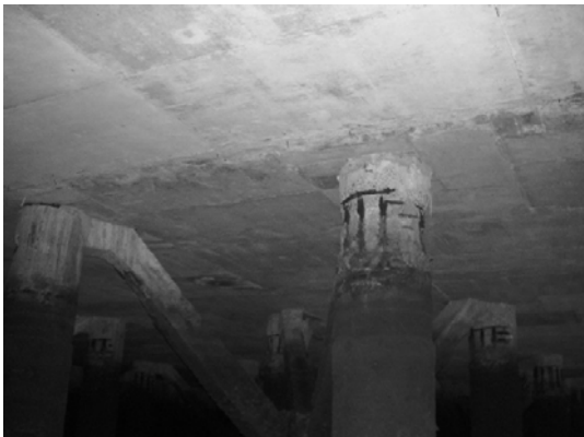
Block 2 Pile 35E-1
