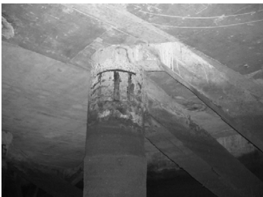
Block 2 Pile 38F-3
