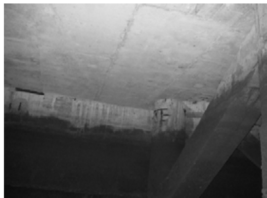
Block 2 Pile 36G
