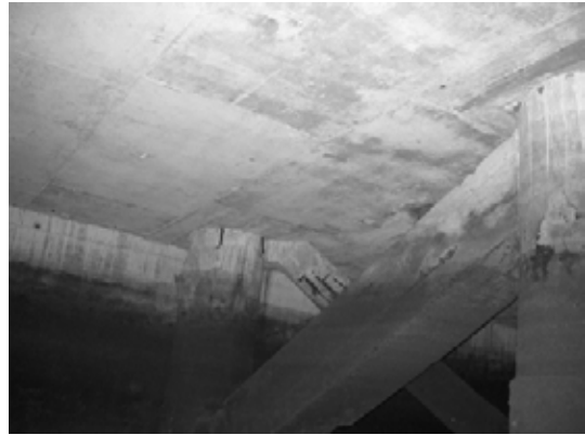
Block 2 Pile 26F ~ 26G-1
