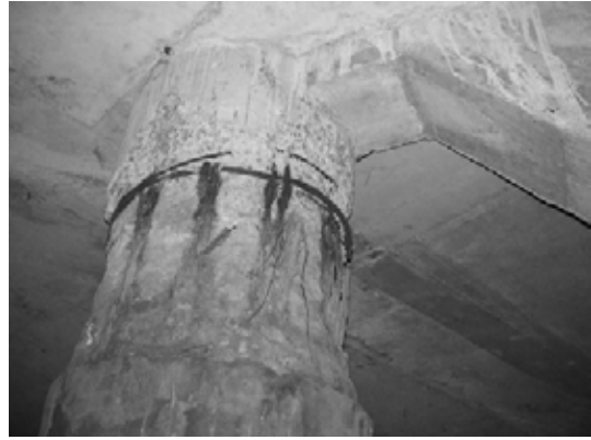
Block 2 Pile 27C-1
