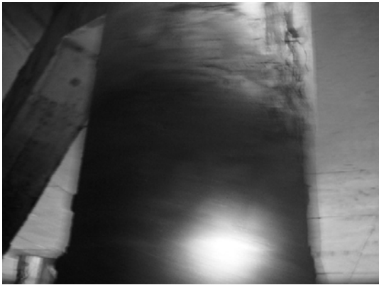
Block 2 Pile 27D-2
