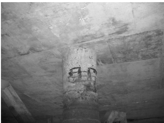
Block 2 Pile 38D-1
