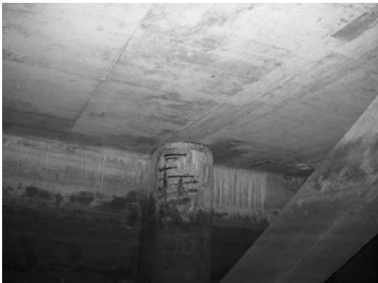
Block 2 Pile 21A
