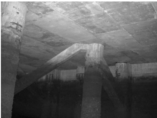
Block 2 Pile 36A ~ 36C
