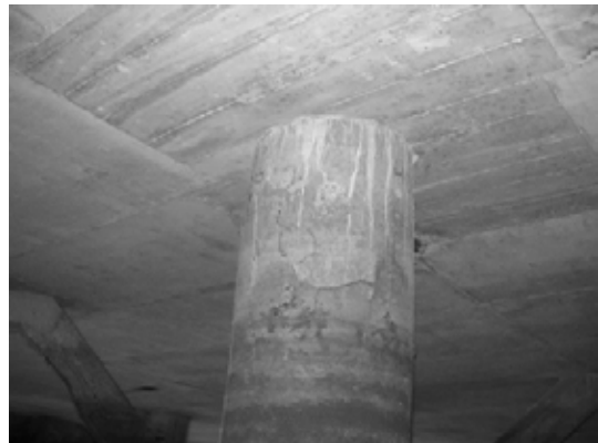
Block 2 Pile 34D
