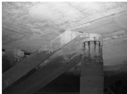
Block 2 Pile 31F
