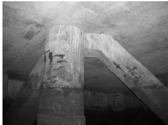
Block 2 Pile 21B
