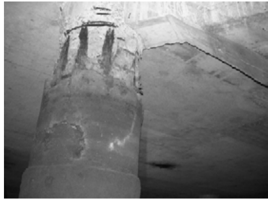
Block 2 Pile 28E-2
