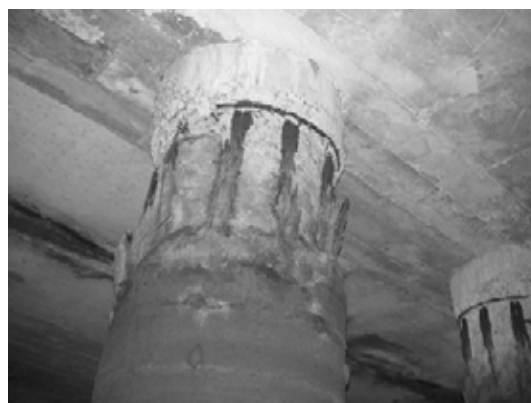
Block 2 Pile 18E-2
