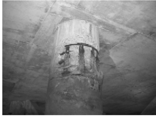
Block 2 Pile 24E-2
