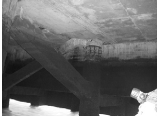
Block 2 Pile 39G
