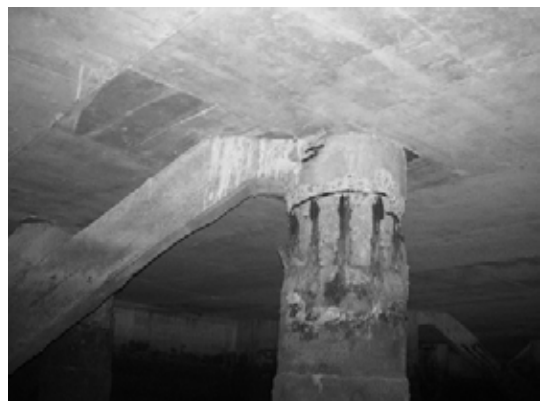
Block 2 Pile 24C
