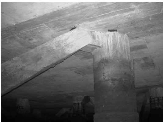
Block 2 Pile 23E-1
