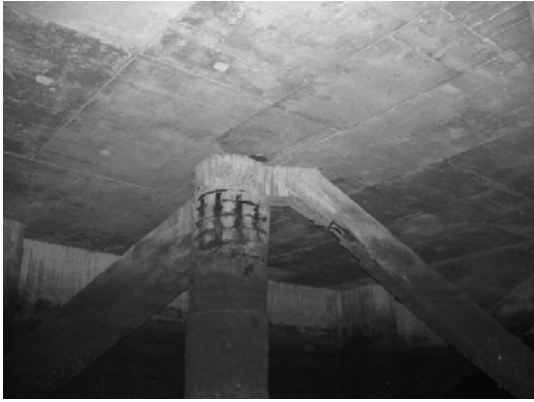
Block 2 Pile 37B
