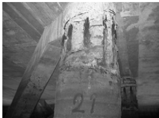
Block 2 Pile 21D
