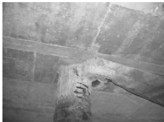
Block 2 Pile 38D-2
