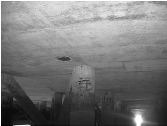
Block 2 Pile 32D-1
