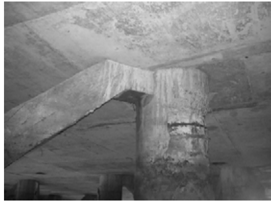
Block 2 Pile 23D-1
