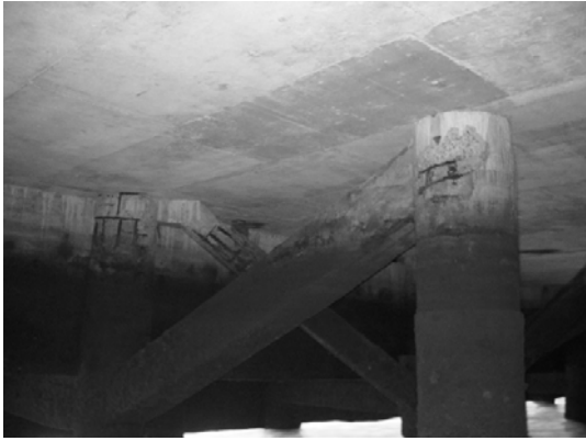
Block 2 Pile 34F-1
