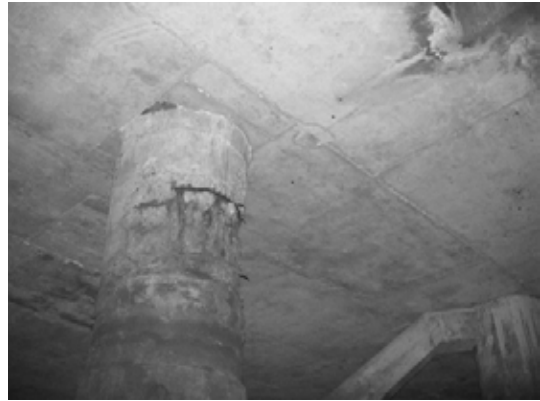
Block 2 Pile 40D-1
