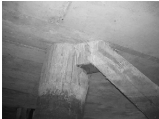
Block 2 Pile 32D-2
