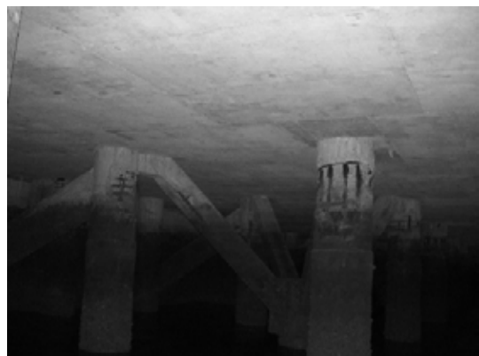
Block 2 Pile 29B ~ 29C
