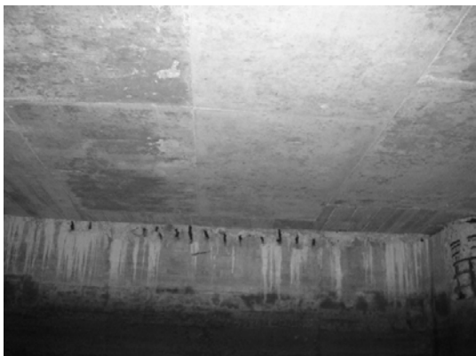
Block 2 Wall bet. Pile 18A & 19A
