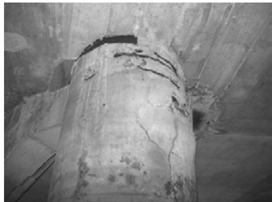
Block 2 Pile 19D-1
