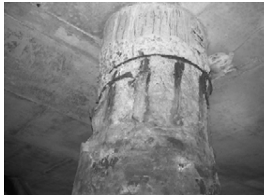
Block 2 Pile 23D-3
