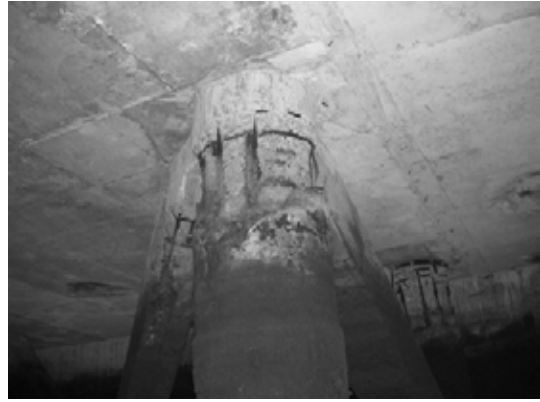
Block 2 Pile 35F-3
