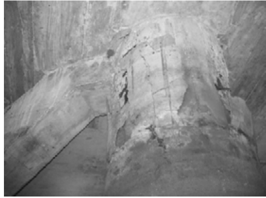
Block 2 Pile 26E
