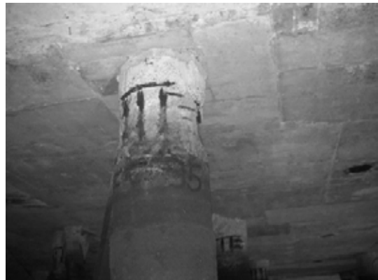
Block 2 Pile 35E-2
