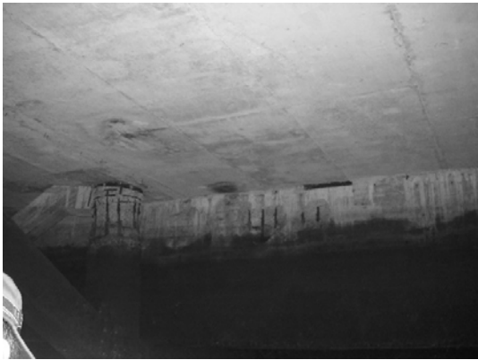
Block 2 Pile 37G-2
