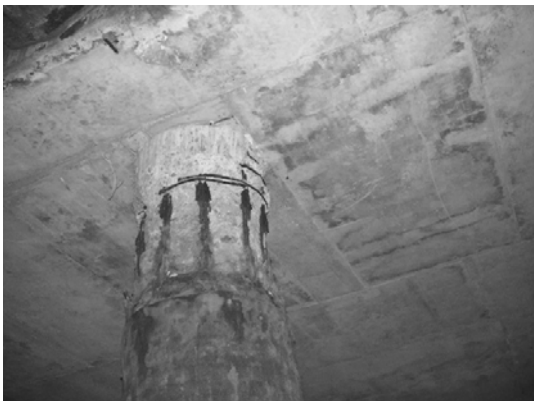
Block 2 Pile 40D-2
