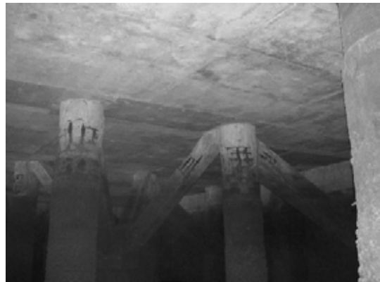
Block 2 Pile 38B ~ 38C
