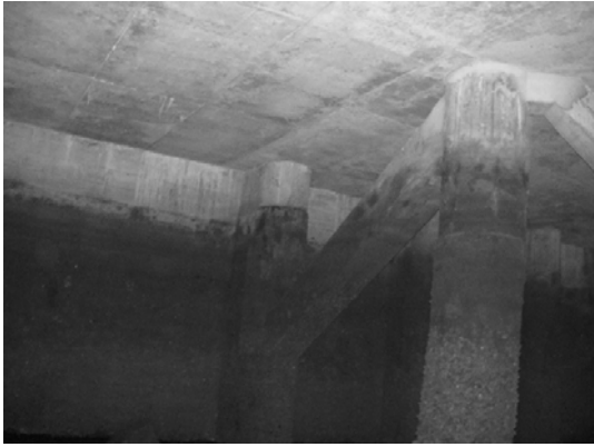
Block 2 Pile 39A ~ 39B
