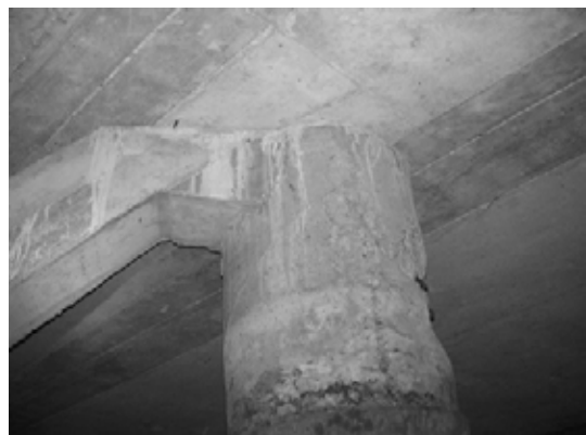
Block 2 Pile 28C
