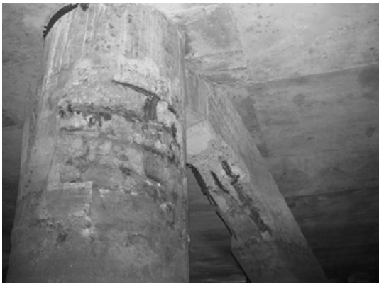
Block 2 Pile 20C-1
