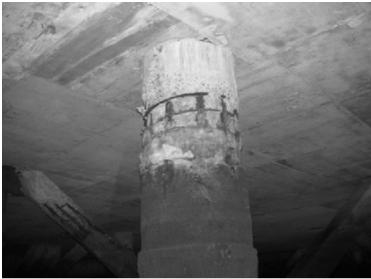
Block 2 Pile 23E-3
