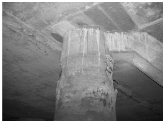
Block 2 Pile 23C-1
