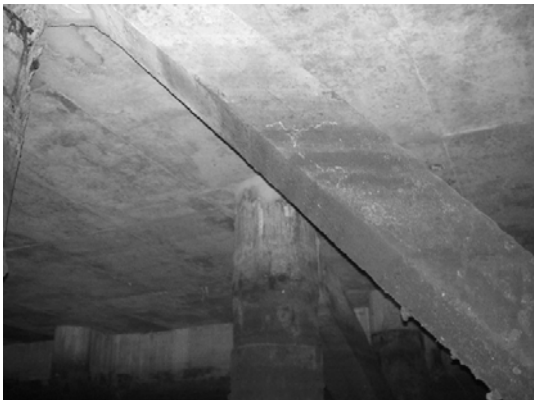
Block 2 Pile 38B
