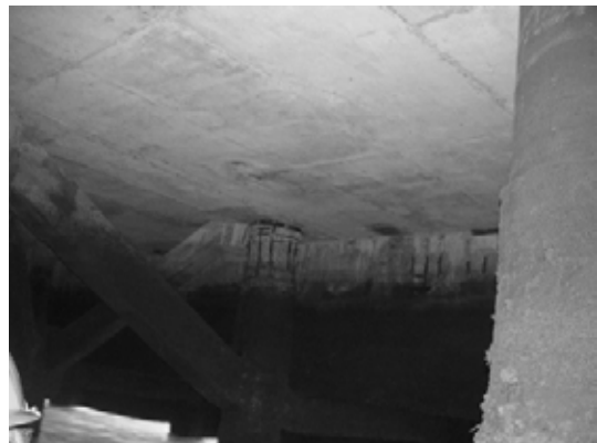
Block 2 Pile 37G-1
