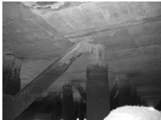
Block 2 Pile 35D-1
