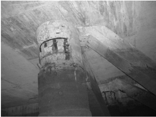
Block 2 Pile 26F
