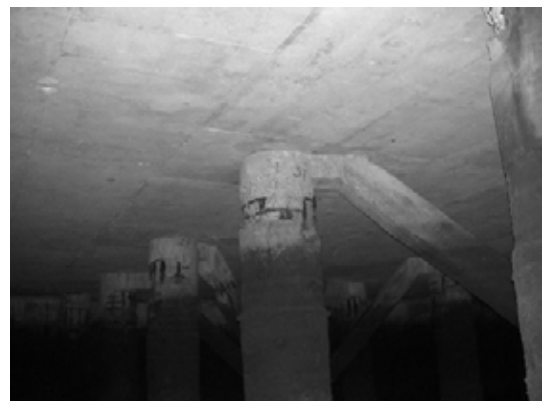
Block 2 Pile 31D-1
