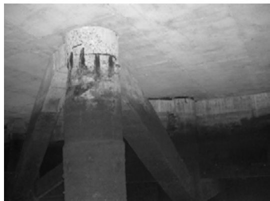
Block 2 Pile 33F-1
