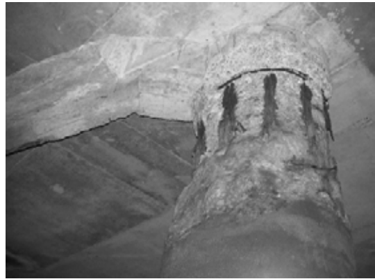
Block 2 Pile 38E-2
