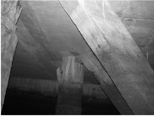
Block 2 Pile 27B
