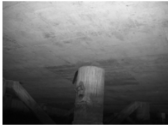
Block 2 Pile 27C-3
