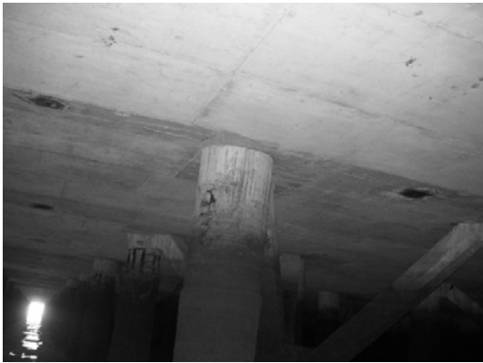
Block 2 Pile 30E-1
