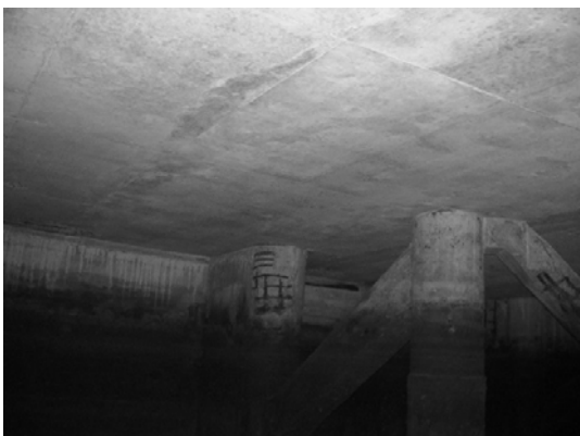
Block 2 Pile 31A ~ 31B
