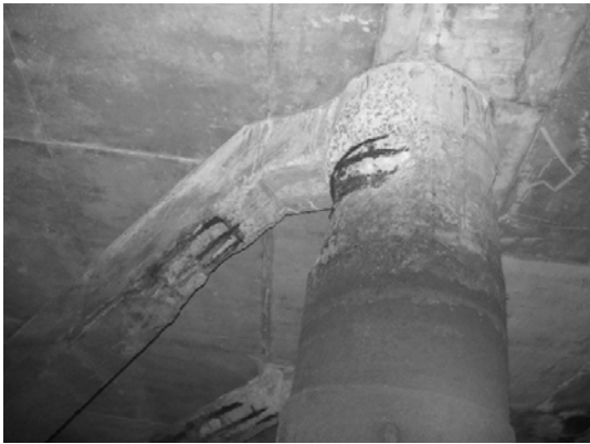
Block 2 Pile 38E-1
