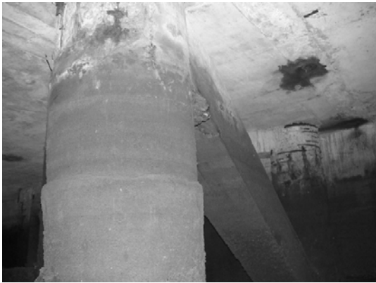
Block 2 Brace bet. Pile 29F & 29G
