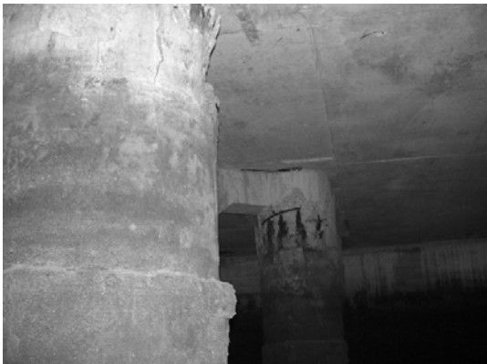
Block 2 Pile 30B
