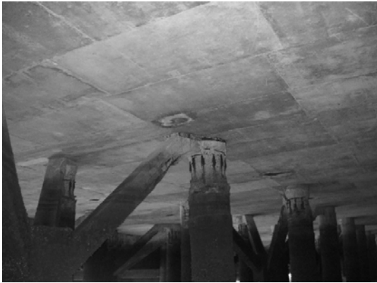
Block 2 Pile 37D-1
