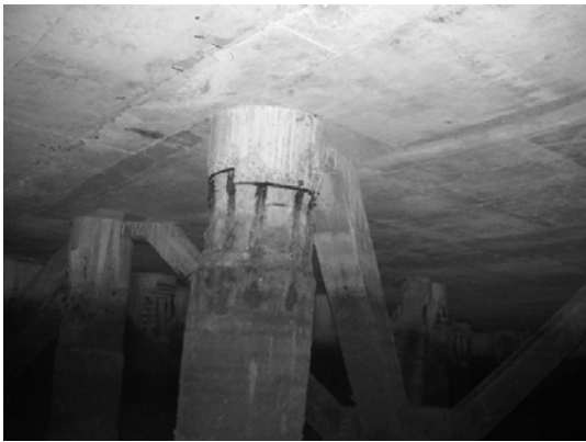
Block 2 Pile 27C-2
