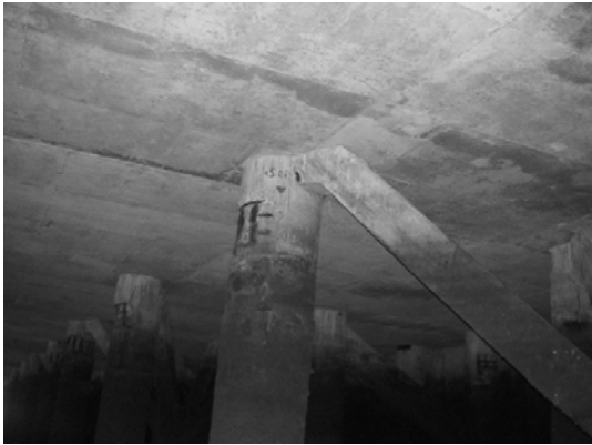
Block 2 Pile 35C-1
