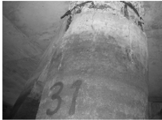
Block 2 Pile 31D-3
