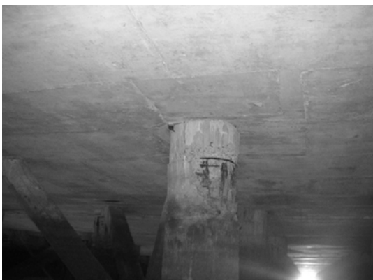
Block 2 Pile 30D
