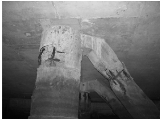
Block 2 Pile 30C
