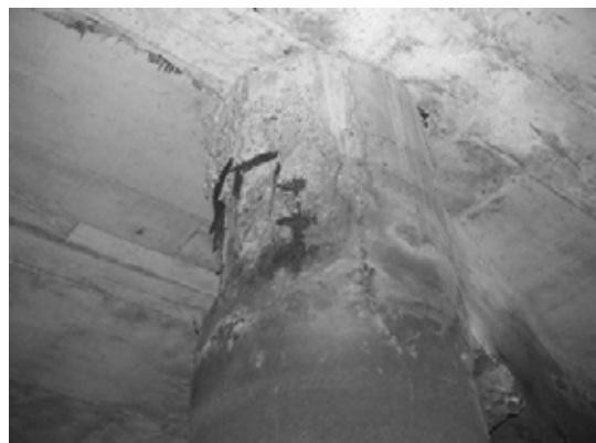
Block 2 Pile 29E-3
