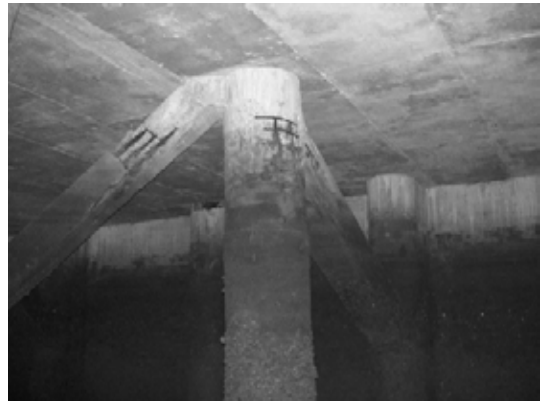
Block 2 Pile 38A ~ 38B
