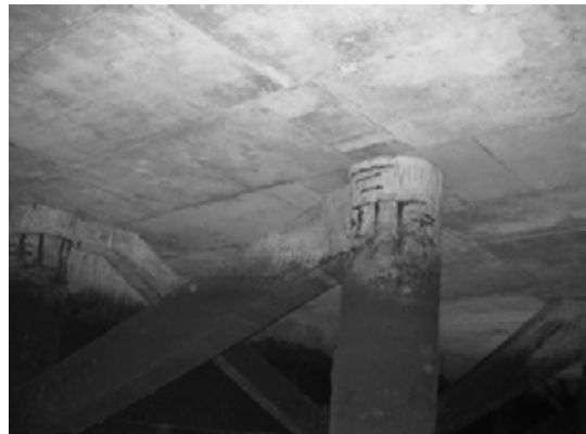
Block 2 Pile 38F-2
