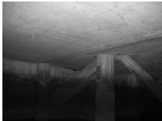
Block 2 Pile 27F ~ 27B
