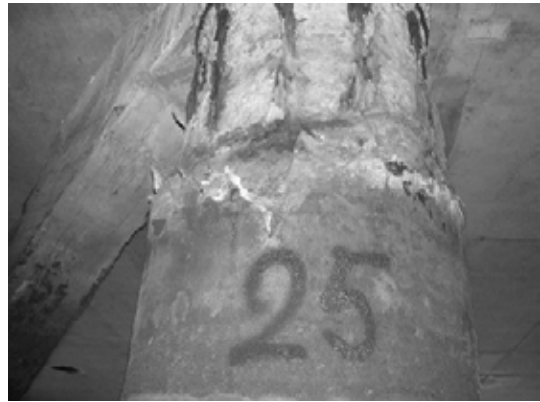
Block 2 Pile 25D
