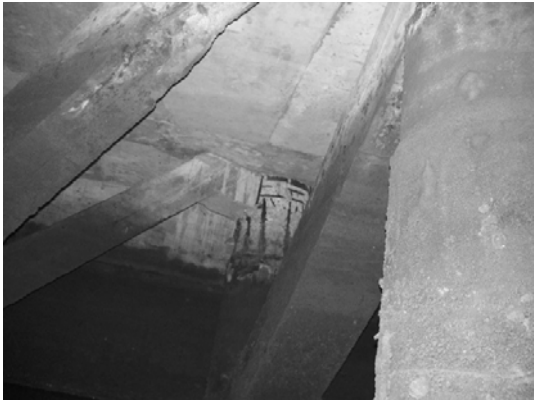
Block 2 Pile 35F-4
