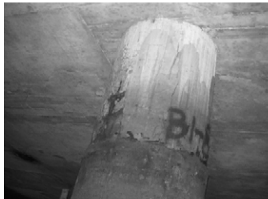
Block 1 Pile 8E-3
