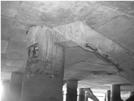
Block 1 Pile 4E-2
