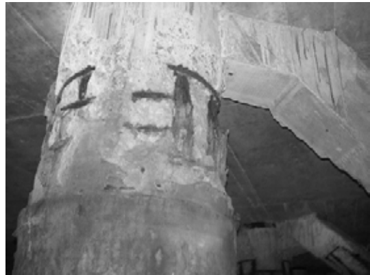
Block 1 Pile 10C
