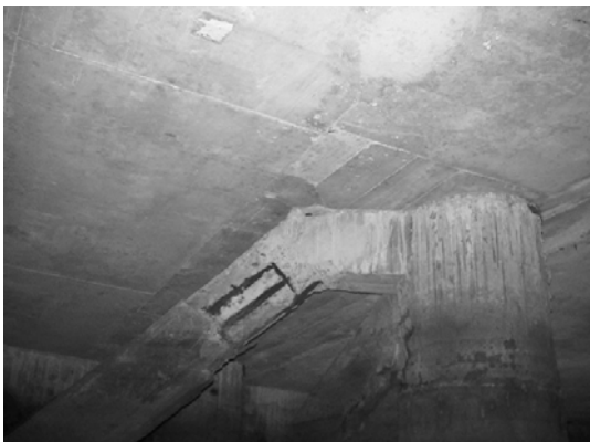
Block 1 Beam bet. Pile 12F & 106c-1
