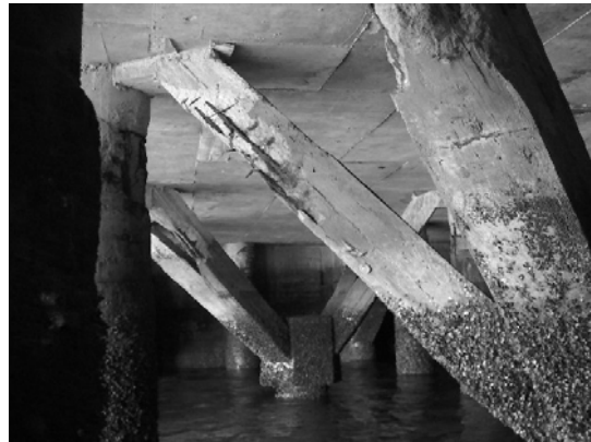
Block 1 Pile 101b-4
