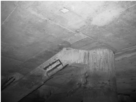
Block 1 Beam bet. Pile 12F & 106c-3
