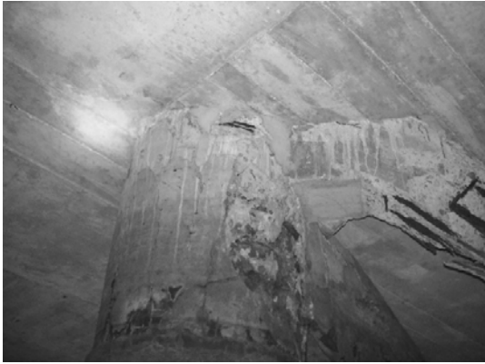
Block 1 Pile 13F
