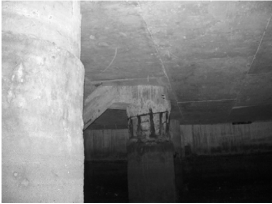
Block 1 Pile 11B-3
