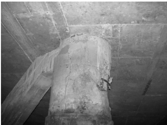
Block 1 Pile 17C-2
