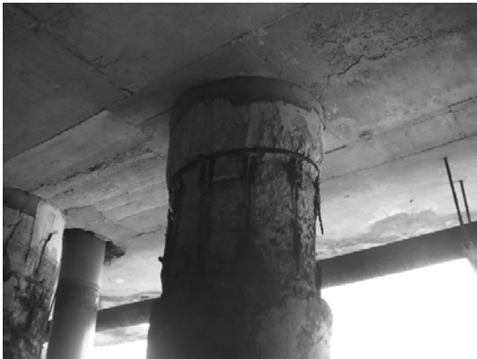
Block 1 Pile 1B-1
