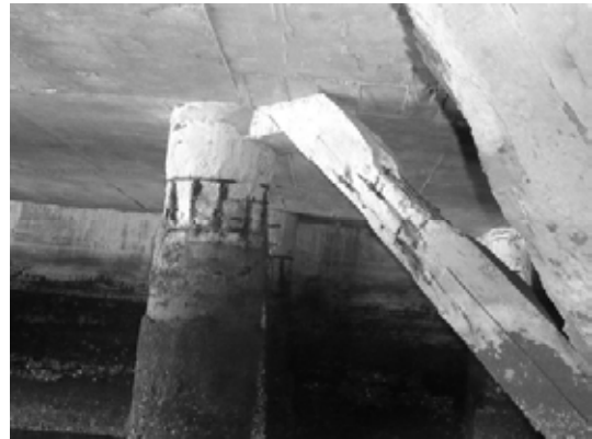
Block 1 Pile 4B
