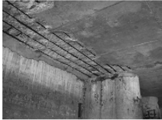
Block 1 Slab bet. Pile 1A& 2A-2
