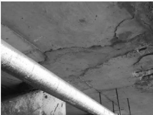
Block 1 Slab nearby Pile 1B-1
