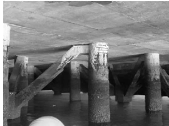
Block 1 Pile 4E-3
