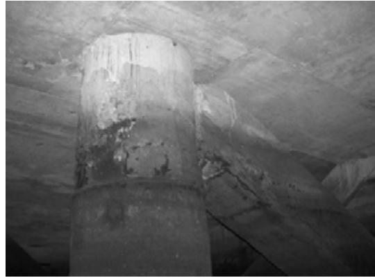
Block 1 Pile 8F-1
