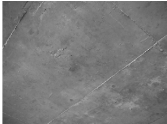
Block 1 Slab bet. Pile 1B & 2B
