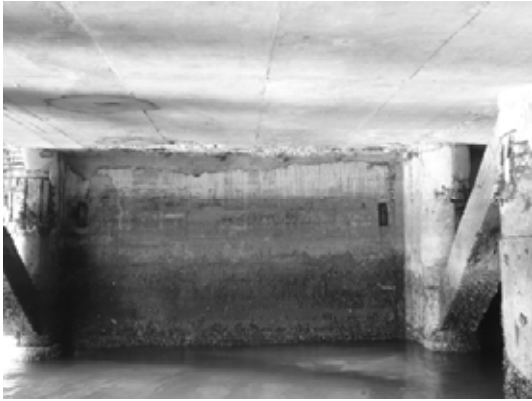
Block 1 Wall bet. Pile 1A & 2A-1
