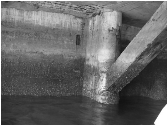
Block 1 Pile 2A
