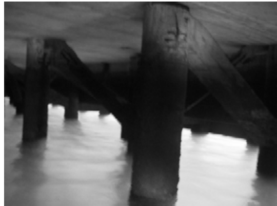
Block 1 Pile 12F-3
