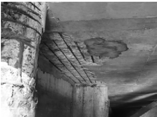
Block 1 Slab bet. Pile 1A& 2A-5
