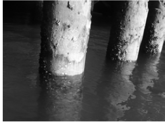
Block 1 Pile 1B ~ 1C
