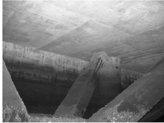
Block 1 Pile 106c
