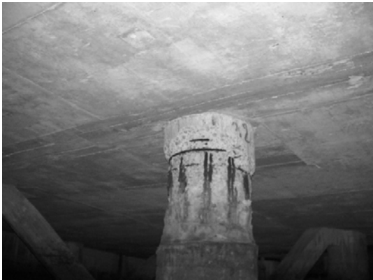
Block 1 Pile 14C-1
