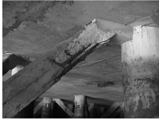
Block 1 Pile 101b-2
