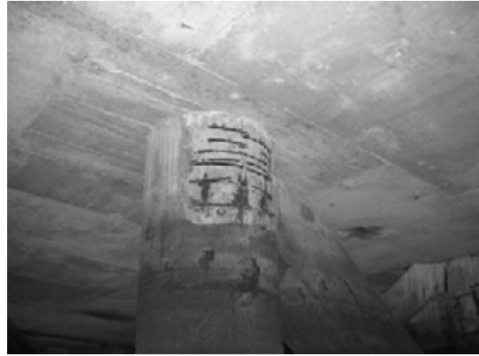
Block 1 Pile 16F-1
