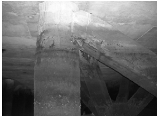
Block 1 Pile 8F-3
