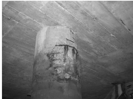
Block 1 Pile 17E-3
