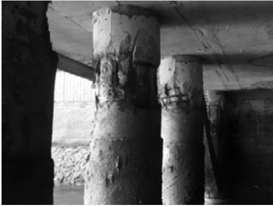
Block 1 Pile 1B & 1a
