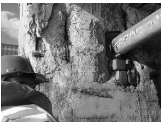
Block 1 Wall nearby Pile 1A
