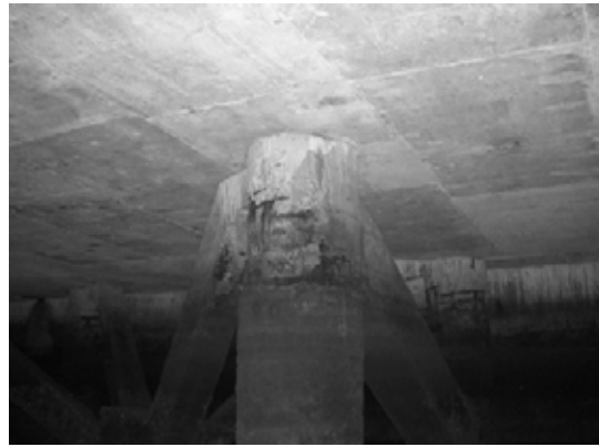
Block 1 Pile 14F-2
