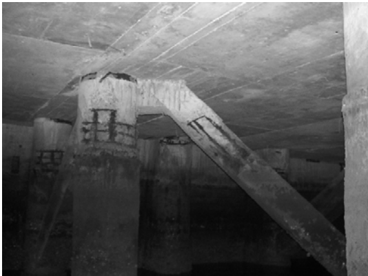
Block 1 Pile 10B
