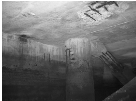
Block 1 Pile 5G-2
