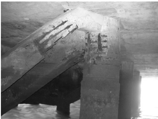
Block 1 Pile 6F
