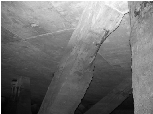
Block 1 Pile 16E-1
