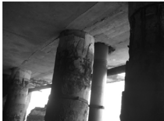
Block 1 Pile 1C
