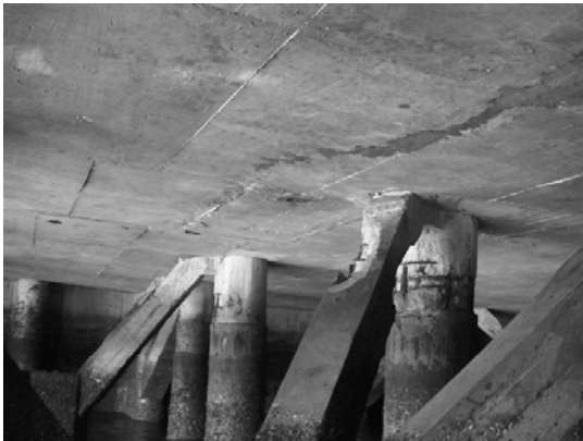
Block 1 Pile 101b-3
