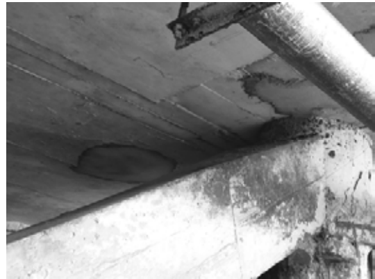
Block 1 Pile 1B-2
