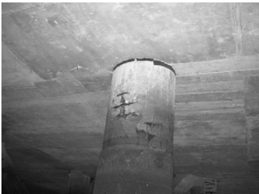
Block 1 Pile 10E-1
