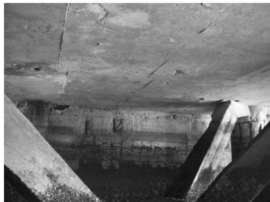
Block 1 Pile 101c-2
