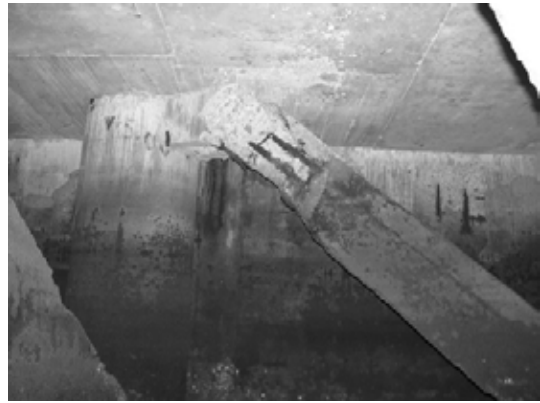
Block 1 Pile 7G
