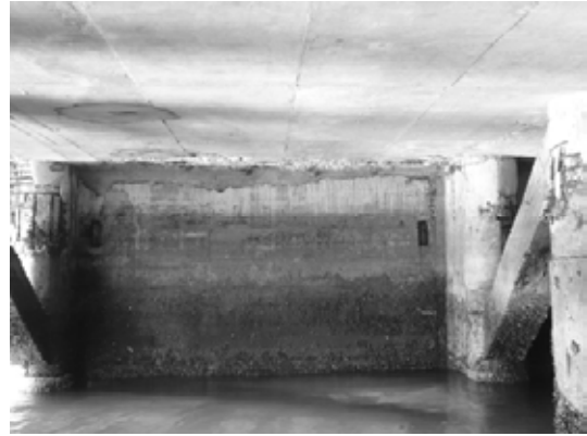
Block 1 Wall bet. Pile 1A & 2A-2
