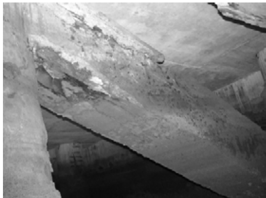
Block 1 Brace bet. Pile 7F & 7G
