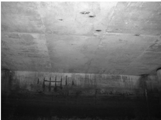
Block 1 Wall bet. Pile 11G & 12G-1
