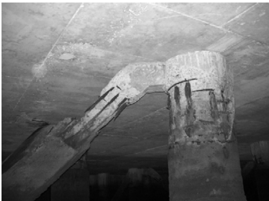
Block 1 Pile 7E-2
