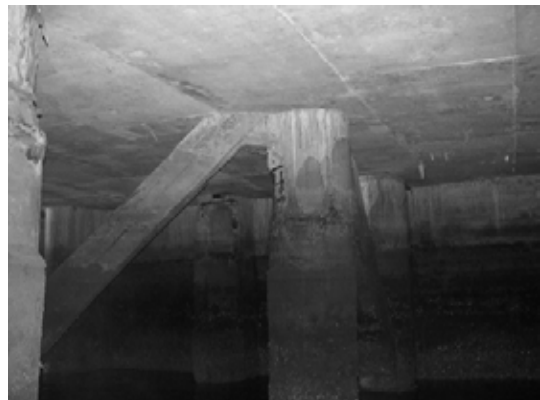
Block 1 Pile 9B
