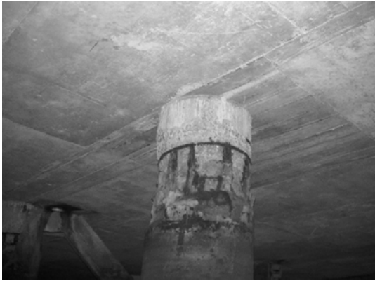
Block 1 Pile 16E-3
