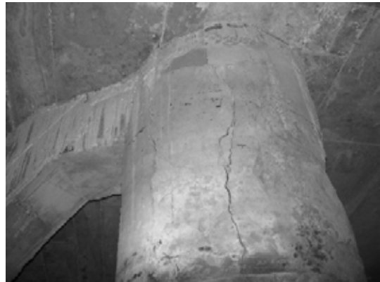
Block 1 Pile 17C-1
