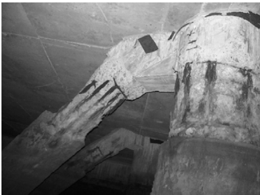
Block 1 Pile 13C
