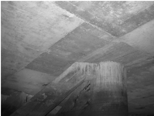
Block 1 Pile 16F-2
