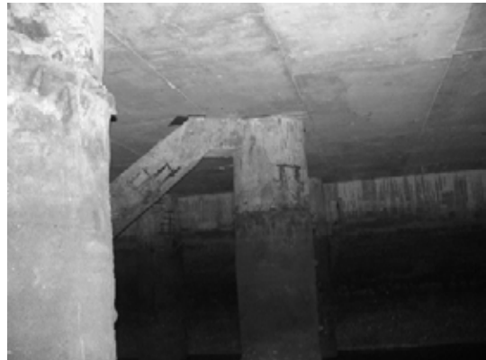
Block 1 Pile 13B
