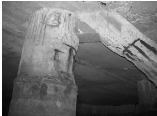
Block 1 Pile 12C-2
