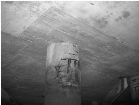
Block 1 Pile 17E-2
