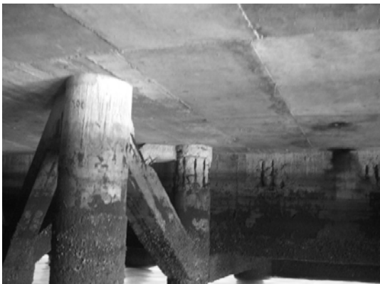
Block 1 Pile 4F ~ 4G
