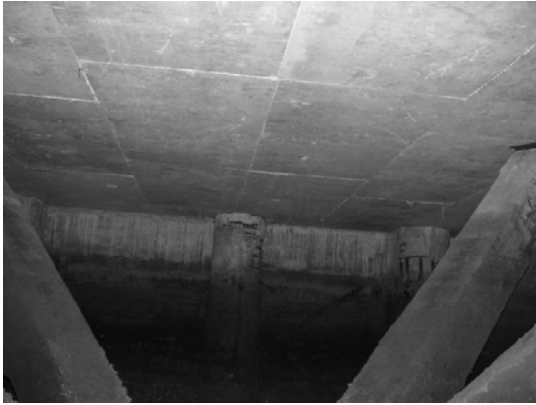
Block 1 Pile 106a
