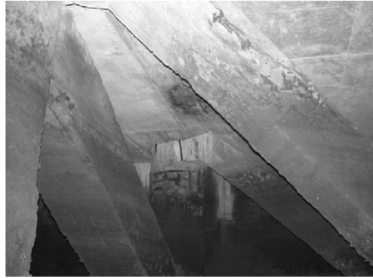
Block 1 Pile 17G-1
