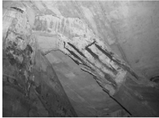
Block 1 Beam bet. Pile 13F & 106c
