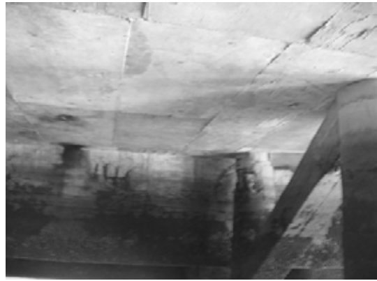
Block 1 Pile 3G
