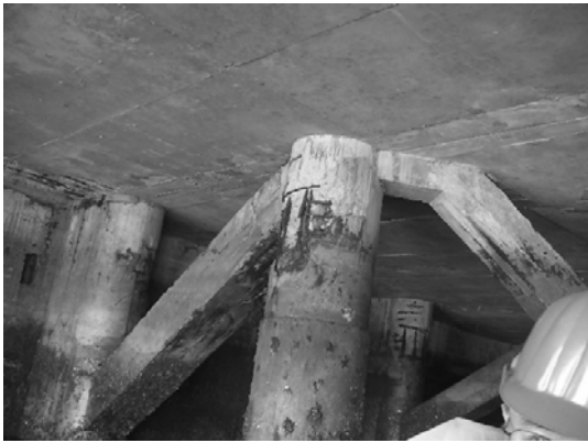
Block 1 Pile 2B-2
