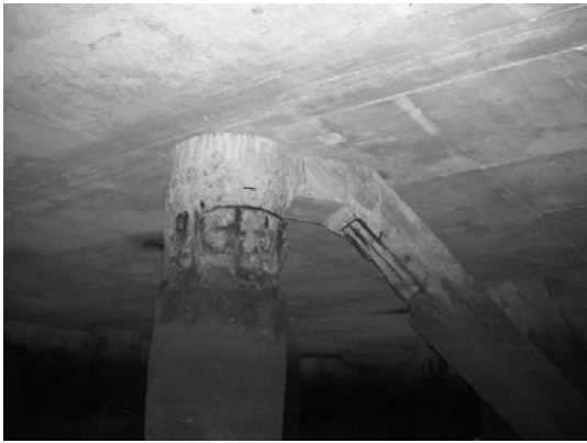
Block 1 Pile 14F-1
