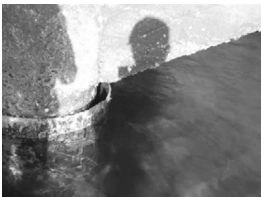
Block 1 Pile 1A
