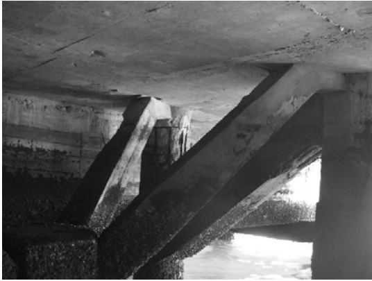
Block 1 Pile 101c-3
