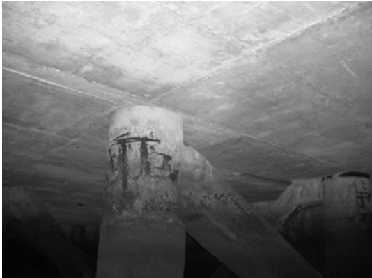
Block 1 Pile 10F-2
