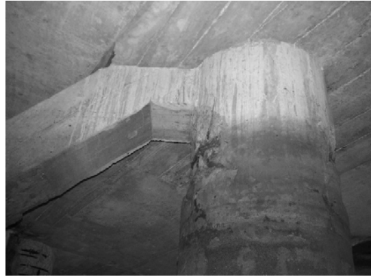
Block 1 Pile 17E-1
