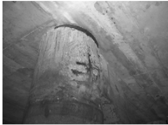
Block 1 Pile 12F-1
