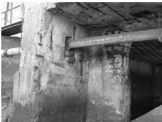
Block 1 Pile 1A and Wall
