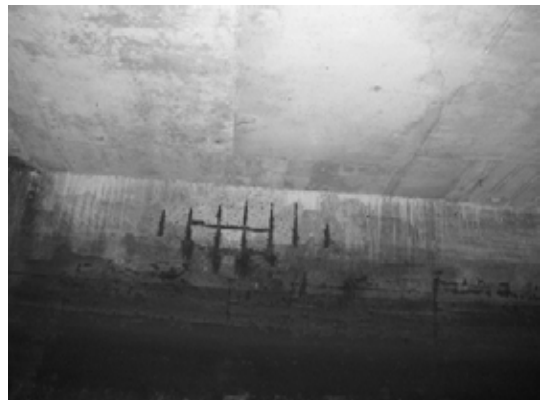
Block 1 Wall bet. Pile 11G & 12G-2
