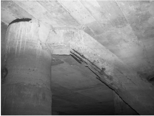
Block 1 Beam bet. Pile 10E & 105b
