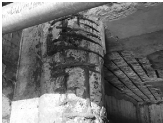
Block 1 Pile 1A and Slab
