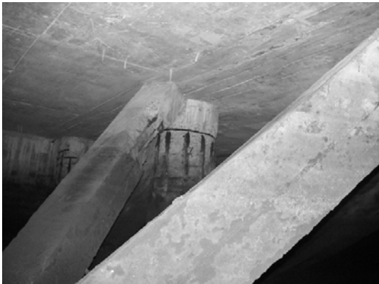
Block 1 Pile 15B
