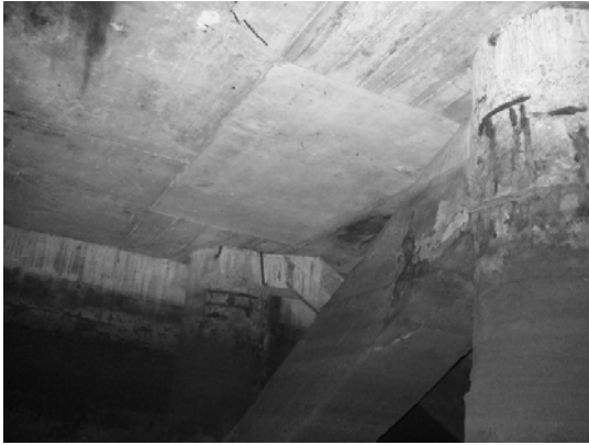
Block 1 Pile 17G-2
