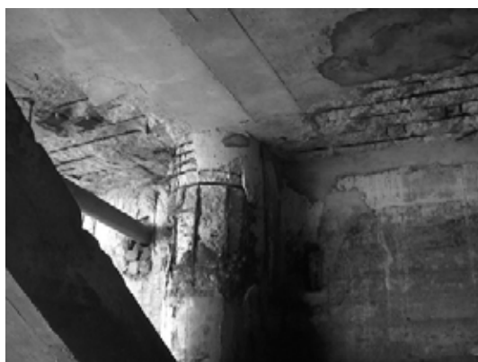
Block 1 Pile 1A
