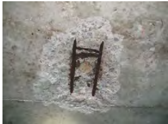
Block 1 Slab bet. Pile 4F & 5F
