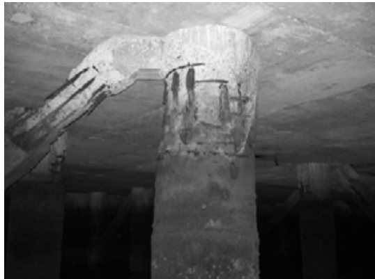
Block 1 Pile 7E-1
