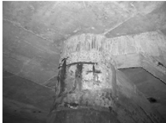
Block 1 Pile 11F
