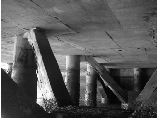
Block 1 Pile 101b-1
