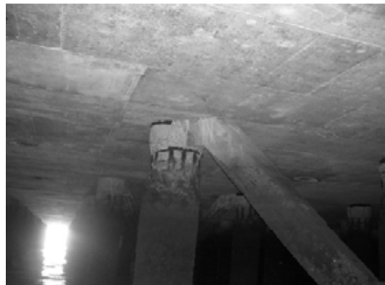
Block 1 Pile 16E-2
