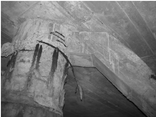
Block 1 Pile 16C
