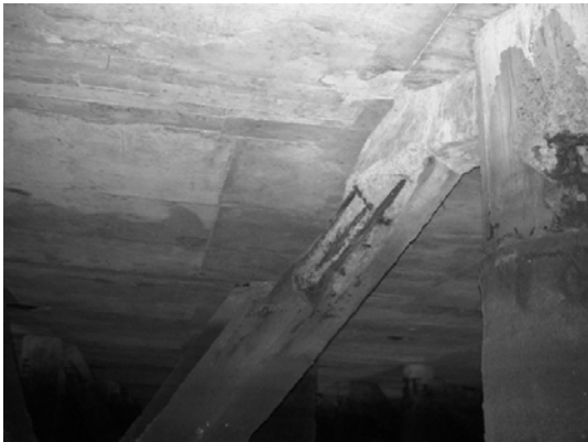
Block 1 Pile 8F-2
