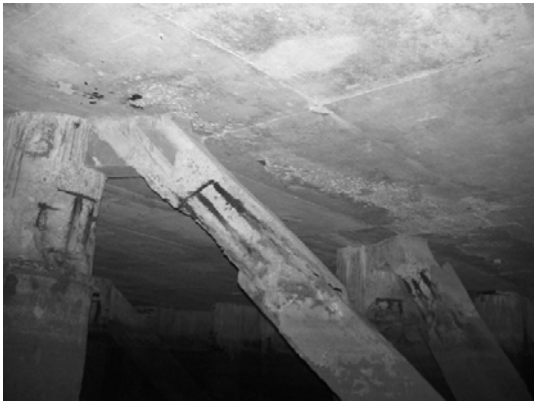
Block 1 Pile 12C-1
