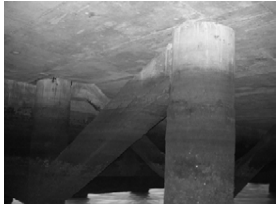
Block 1 Pile 9F
