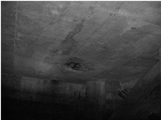
Block 1 Pile 5G-1
