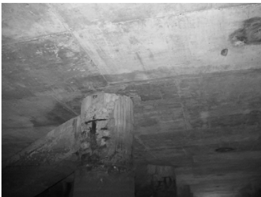
Block 1 Pile 17F-1
