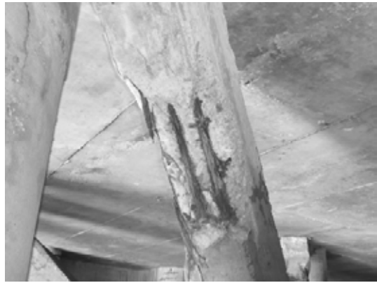
Block 1 Beam bet. Pile 2C & 101a
