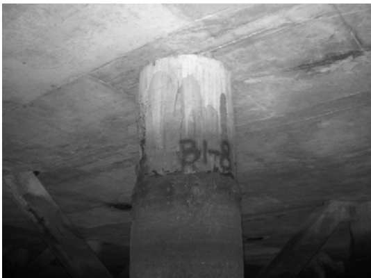
Block 1 Pile 8E-2
