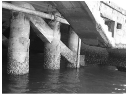
Block 1 Pile 1F ~ 1d
