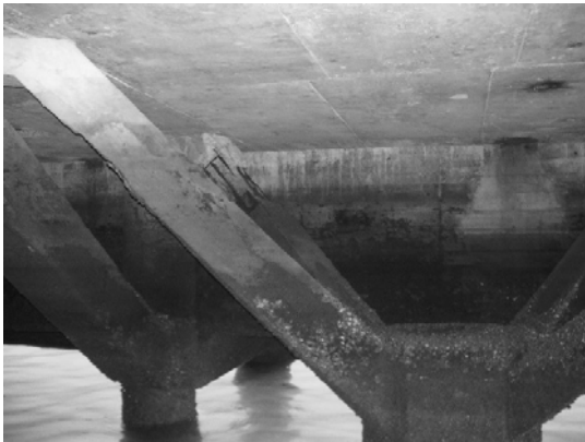
Block 1 Pile 102c
