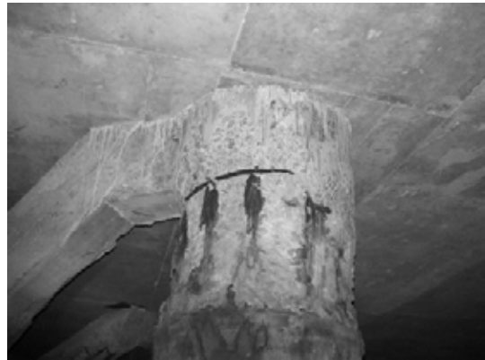
Block 1 Pile 14C-2
