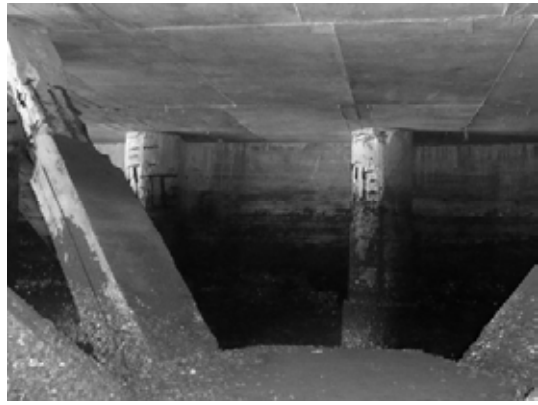
Block 1 Pile 102a
