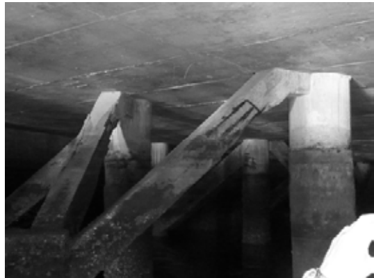
Block 1 Pile 7C
