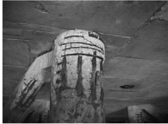
Block 1 Pile 4E-1
