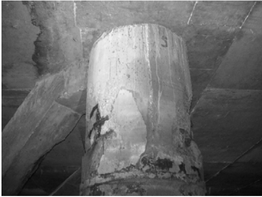
Block 1 Pile 9C-1
