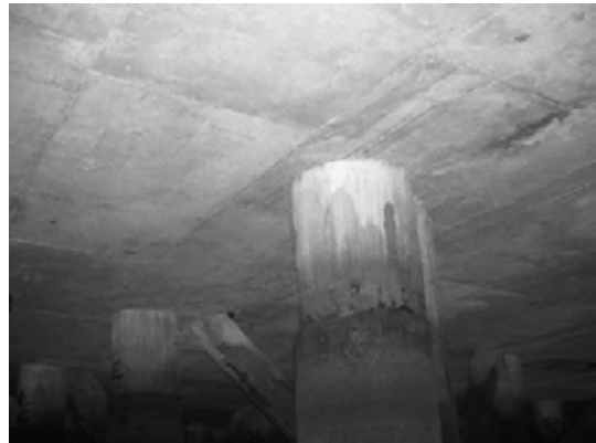
Block 1 Pile 8E-1
