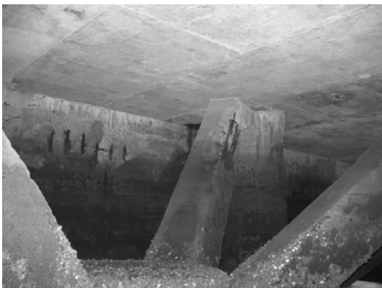
Block 1 Pile 103c
