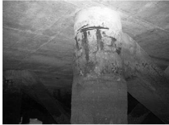
Block 1 Pile 10F-1
