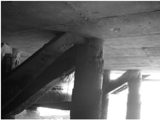
Block 1 Pile 2F
