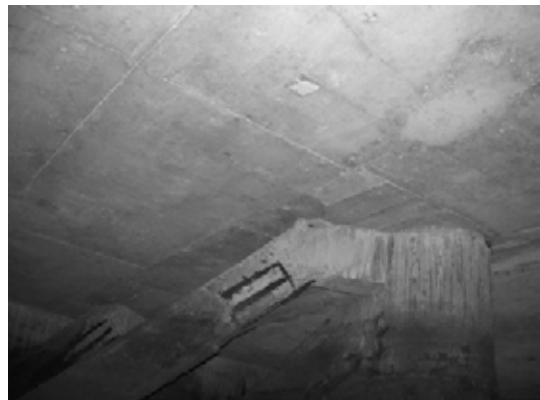
Block 1 Beam bet. Pile 12F & 106c-2
