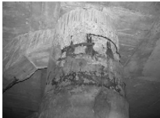
Block 1 Pile 15E-1
