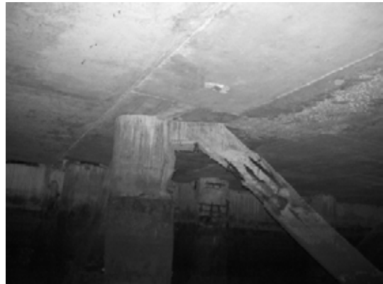
Block 1 Pile 12B
