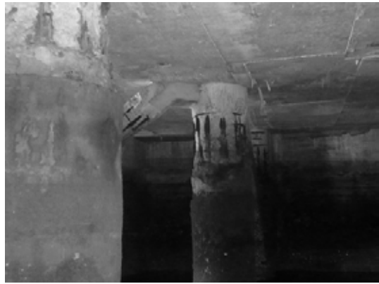
Block 1 Pile 5B
