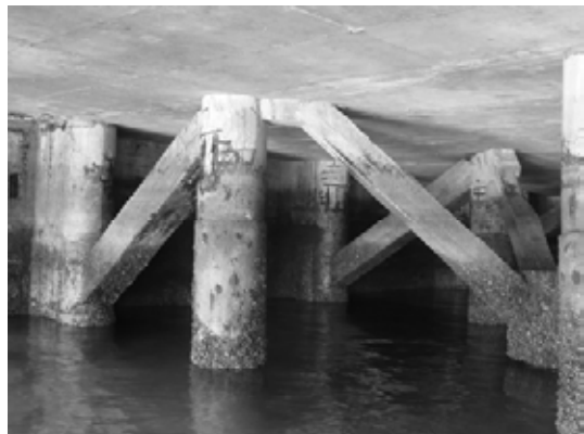
Block 1 Pile 2B-1
