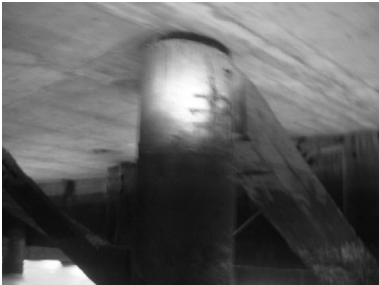
Block 1 Pile 12F-2
