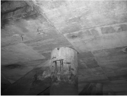
Block 1 Pile 17F-3
