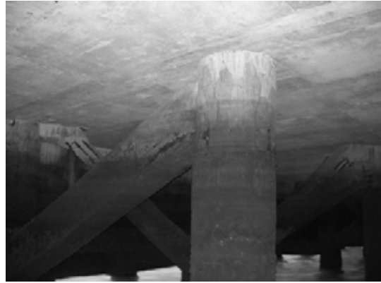
Block 1 Pile 15F
