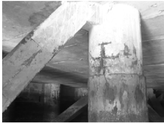
Block 1 Pile 3C
