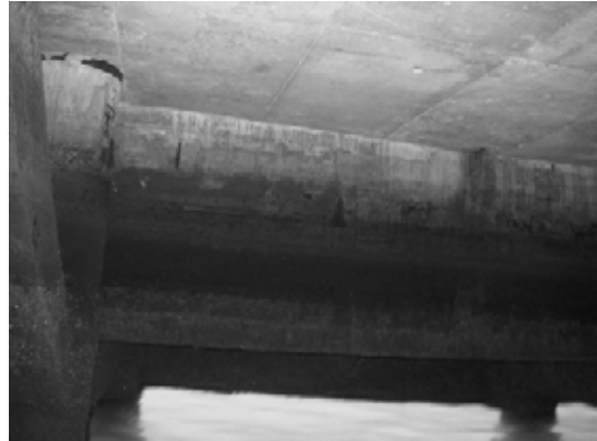
Block 1 Pile 10G
