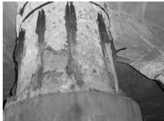
Block 1 Pile 6C
