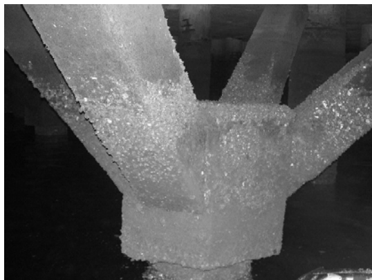
Block 1 Pile 104b
