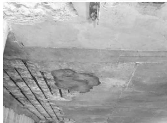
Block 1 Slab bet. Pile 1A& 2A-6
