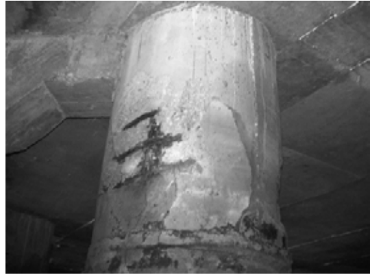
Block 1 Pile 9C-2
