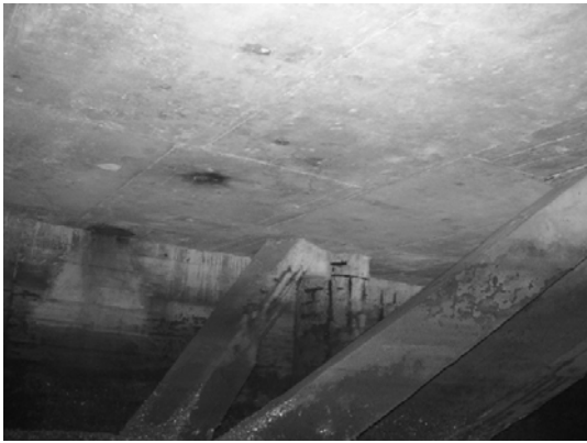
Block 1 Pile 4G
