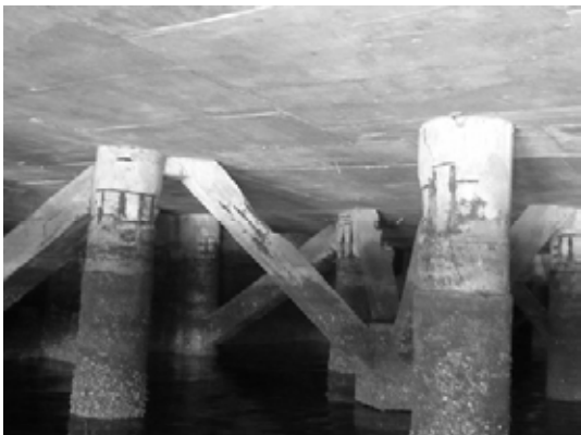
Block 1 Pile 4C
