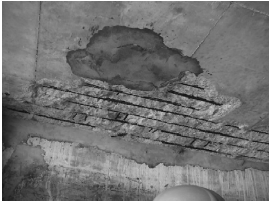
Block 1 Slab bet. Pile 1A& 2A-1
