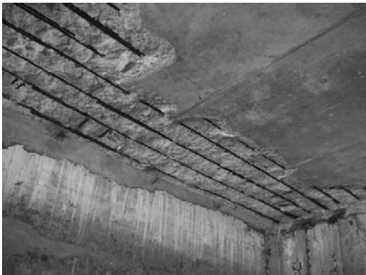
Block 1 Slab bet. Pile 1A& 2A-3
