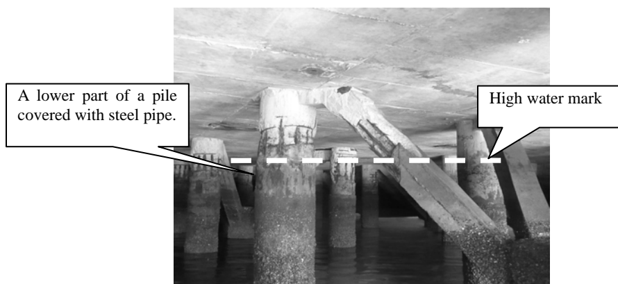
Figure 4.1-9 Overall view of damaged piles and props under the deck concrete
