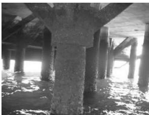
Figure 4.1-10 Supporting pile with head and props
