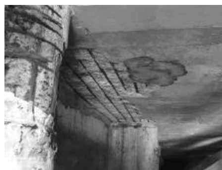
Figure 4.1-12 Stripping from deck concrete from 1 st to 2 nd columns
