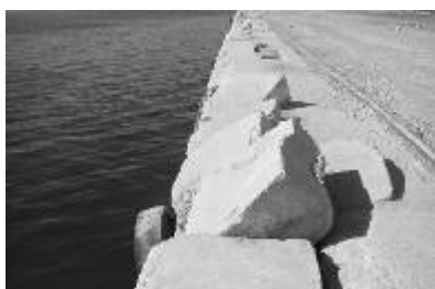
Figure 4.1-24 Deteriorated cap concrete of the general cargo terminal
