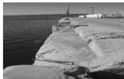
Figure 4.1-24 Deteriorated cap concrete of the general cargo terminal
