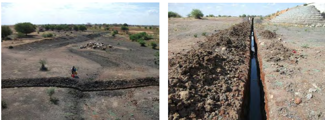
Figure 1.2.6 Upper Stream of Manonga River and Trench at River Floor at Location No. 11
