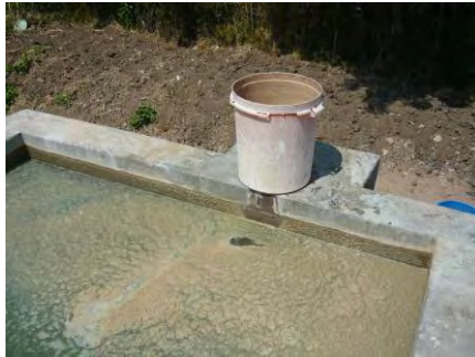
The present point of injection of coagulant
