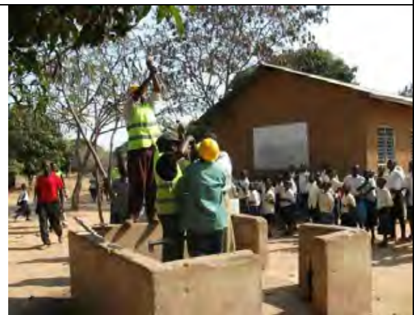
22: Repairing of a hand pump (Nata village, Nzega District)
