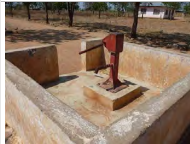
23: A malfunctioned hand pump (Isanga village, Nzega Distrit)
