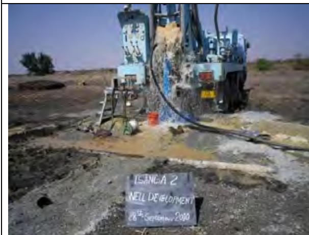
21: Test well drilling (development work)
