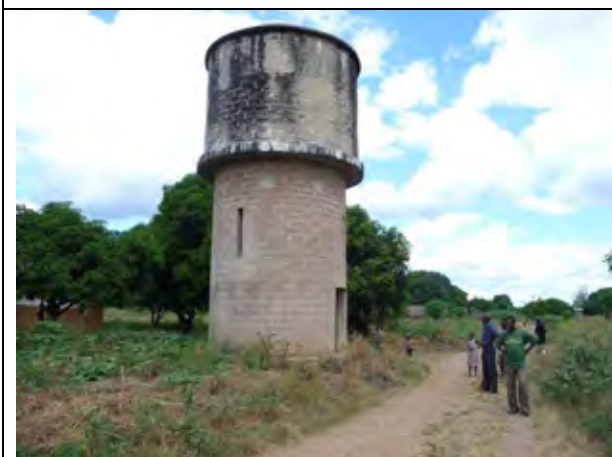
11: An abandoned distribution tank (Sikonge District)
