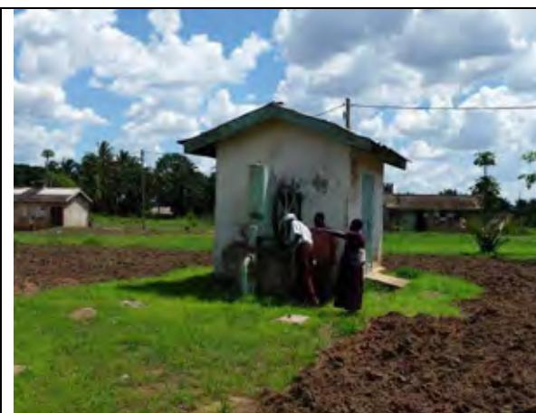
14: A malfunctioned piped water supply scheme (Urambo District)
