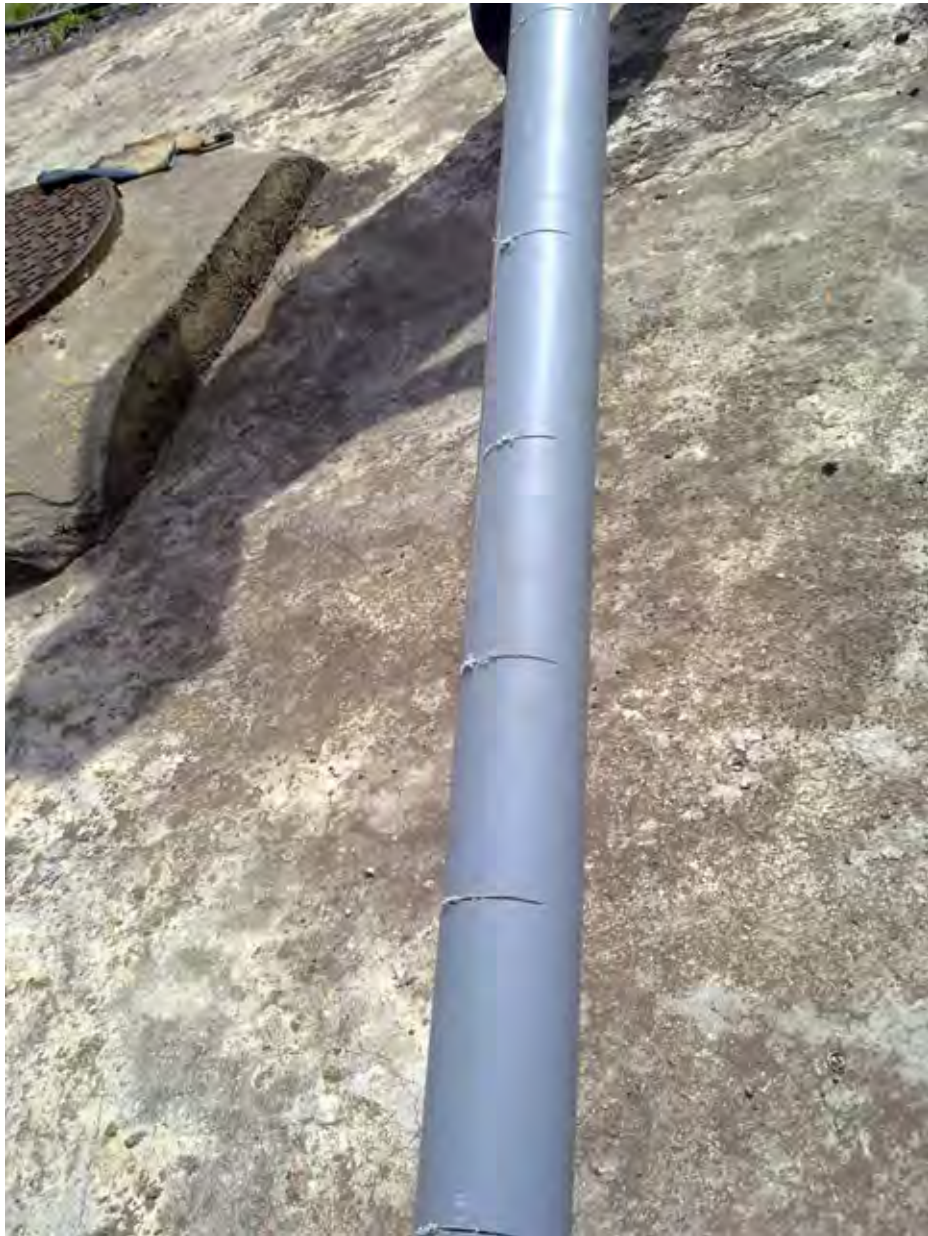
Figure B-3 Slotted tube for standpipe
