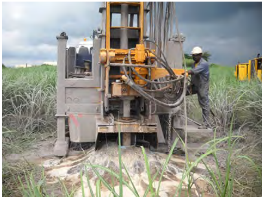
B.1 Drilling of BH 1
