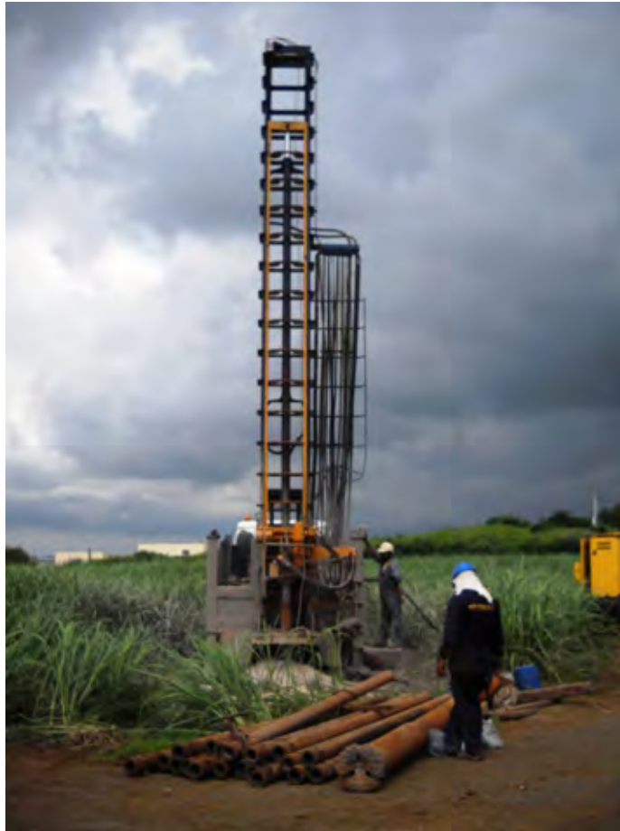
B.1 View of the Site – BH 1
