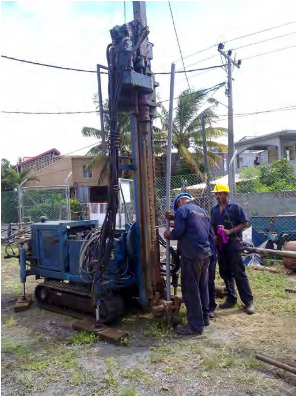
Figure B-2 Installation of standpipe
