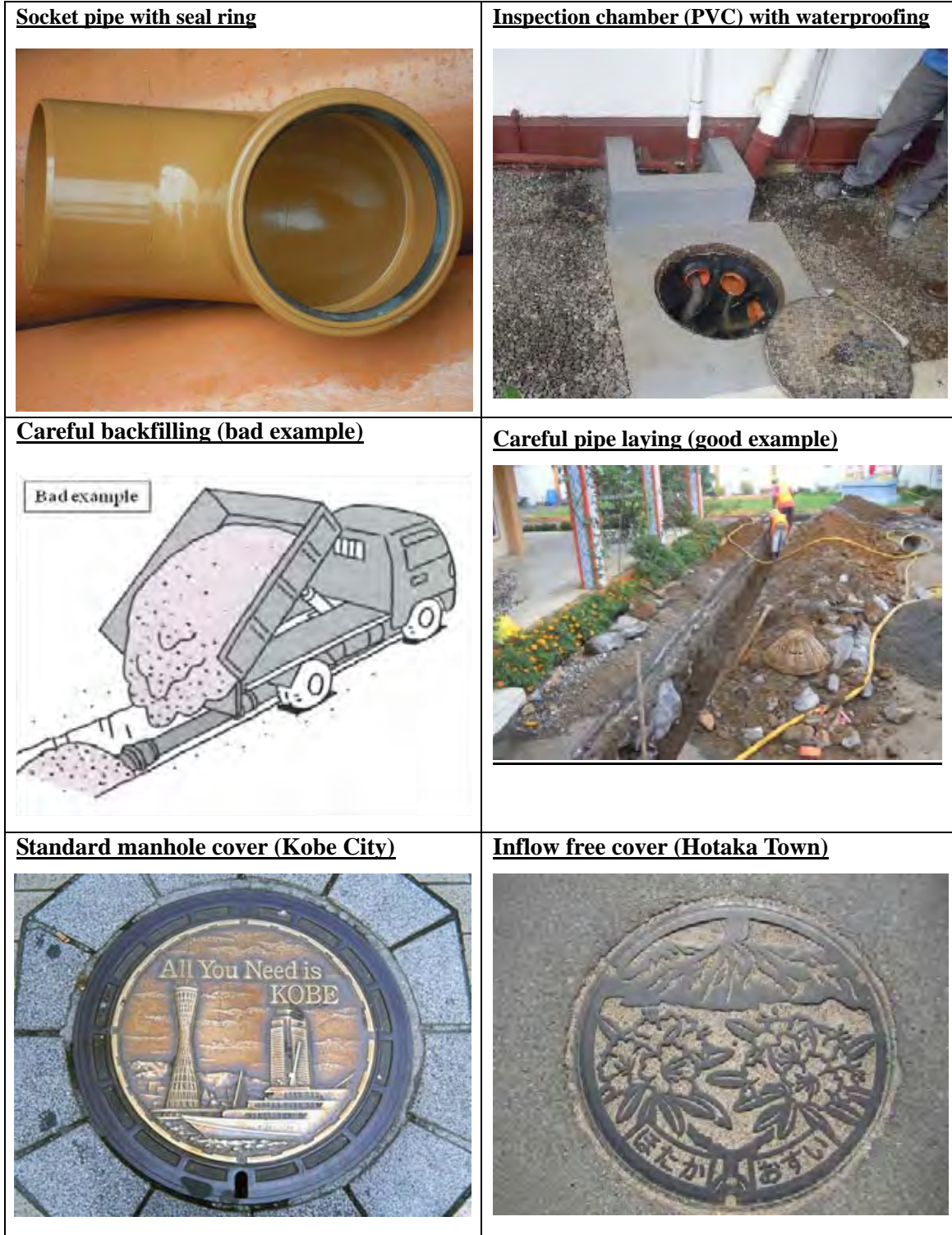
Figure 5.3-4 I/I Mitigation during the Construction Stage (2/2)
