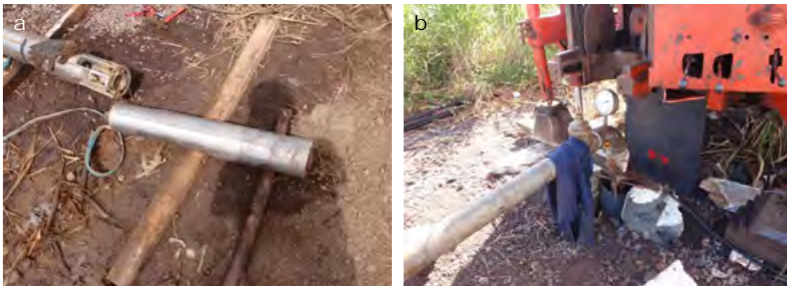
Figure 4.3-4 (a) Pump for Step Test; and (b) Measuring the Yield
