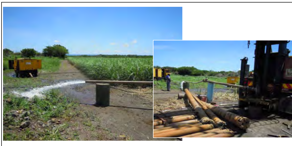
Figure S-9 Pumping Test (Tentative)
