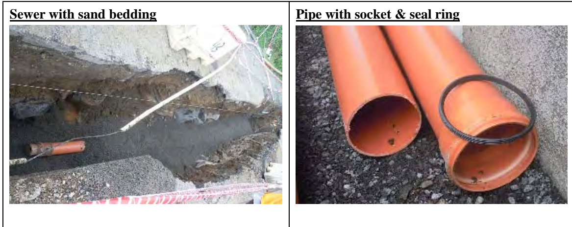
Figure S-11 Sewer Construction
