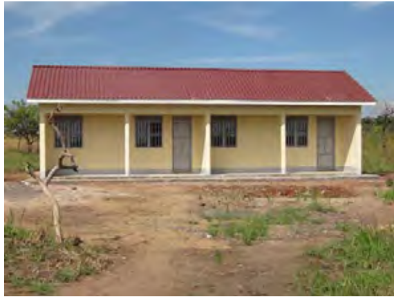
Teachers' quarter after the project (1 block, 2 houses)
