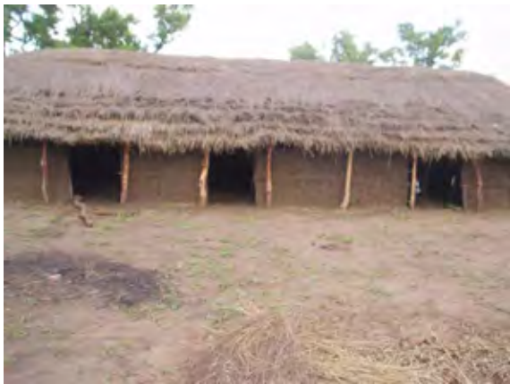
The existing classroom mad by the community
