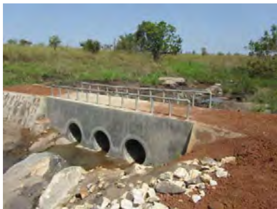
Pipe culvert after the project
