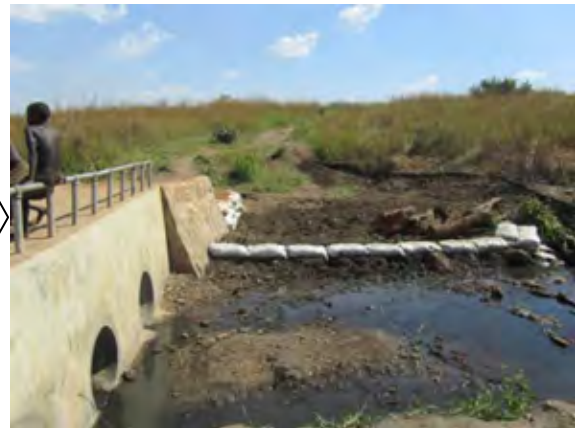
After the Project (Pipe Culver)
