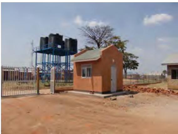
Water Storage Facility (40,000lt water tank)
