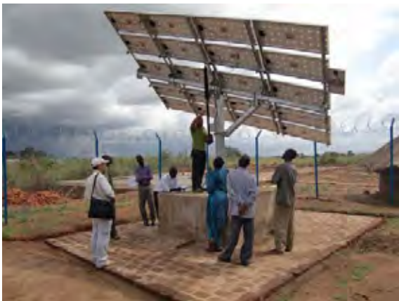
Installation of Solar Panel (For solar powered submersible pump)
