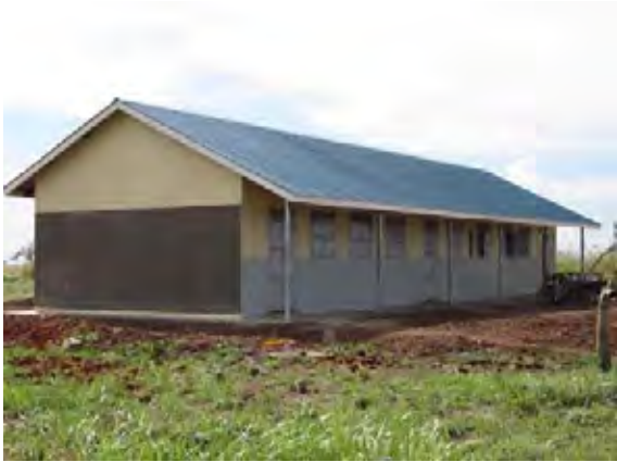
Classroom after the pilot Project (2classroom, 1 office)
