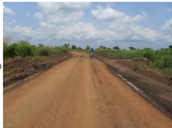
After the Project (Improvement on surface and side drainage)
