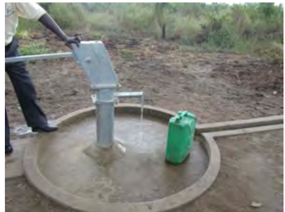
Improved water facility in Lulyango village after the Pilot Project
