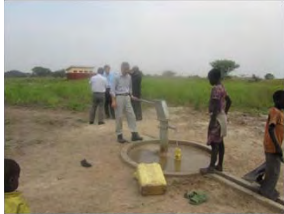
Water supply facility for the school
