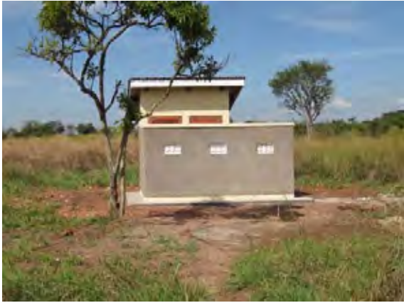
Pit Latrine after the Pilot Project
