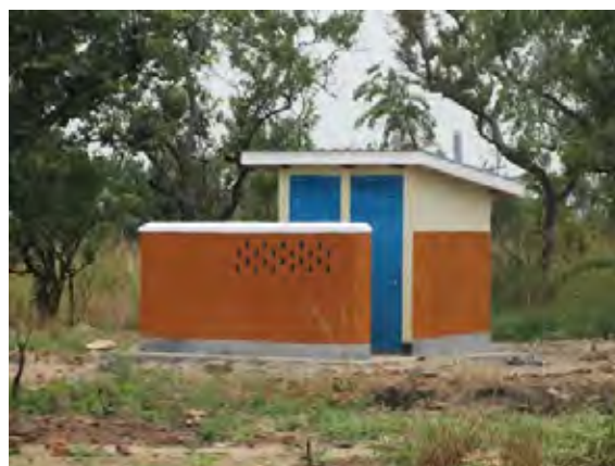
Pit-Latrine after the Project
