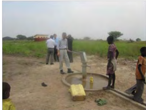
Water supply facility for the school
