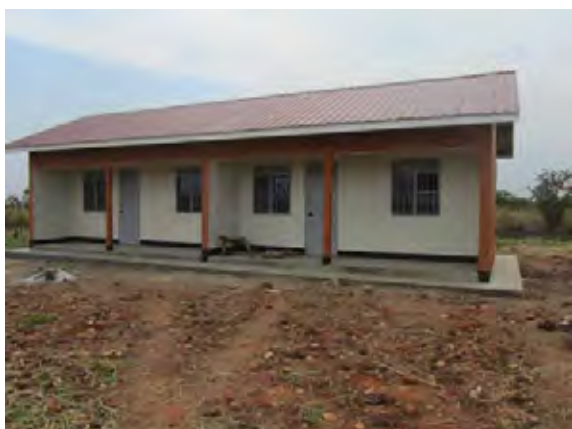
Staff-house after the Project
