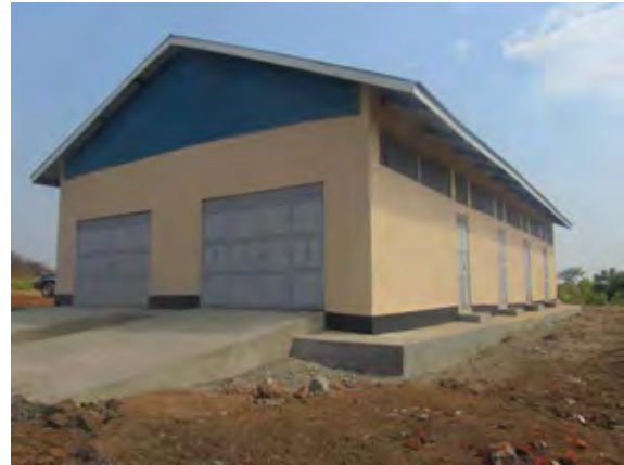
Outside view of the Workshop
