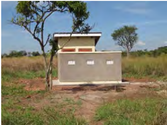
Pit Latrine after the Pilot Project
