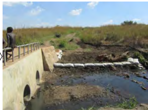
After the Project (Pipe Culver)
