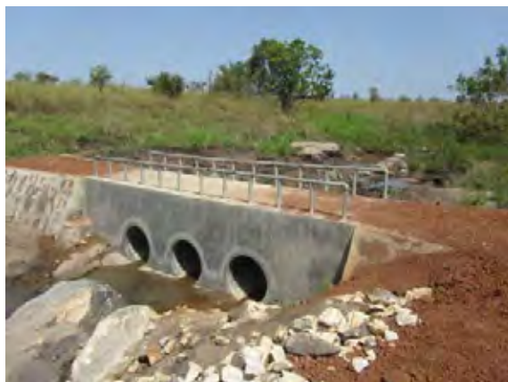
Pipe culvert after the project
