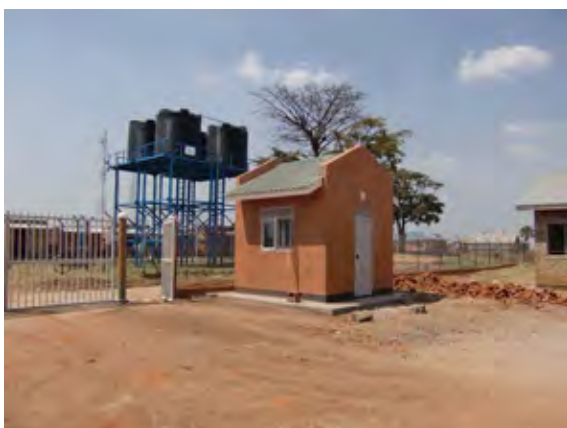
Water Storage Facility (40,000lt water tank)
