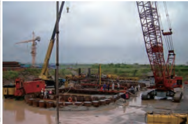
General view of construction of the pier P14
