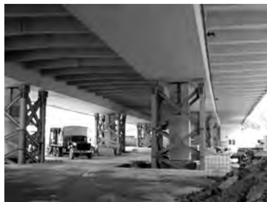
General view of Mecidiyeköy Viaduct
