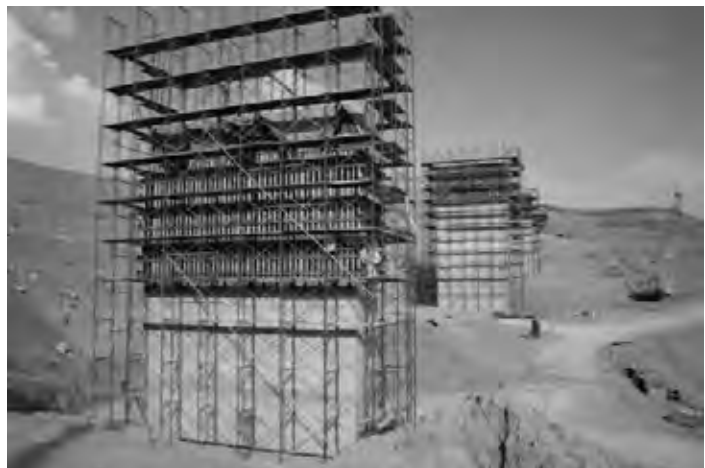
Formwork and scaffolding for bridge No.3
