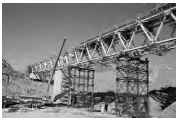
Erection of Steel Deck for Bridge No.5
