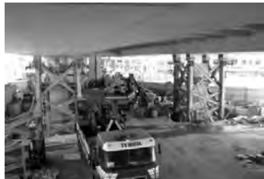
Installation of Bent at Mecidiyeköy
