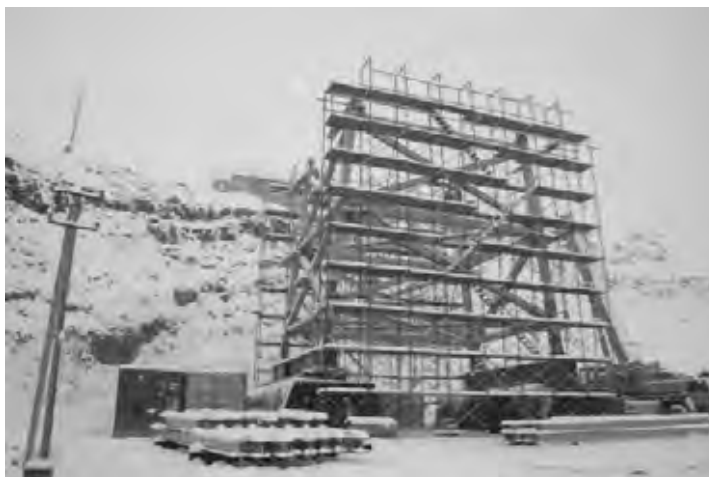
Truss Pier (Bridge No.4)
