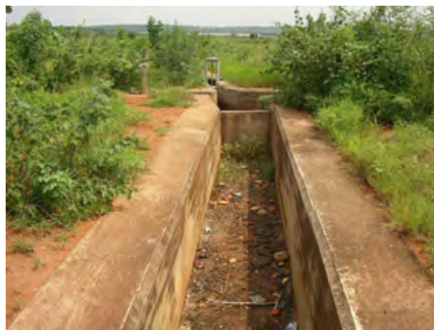
Existing canal originated from the Night Storage Reservoir
