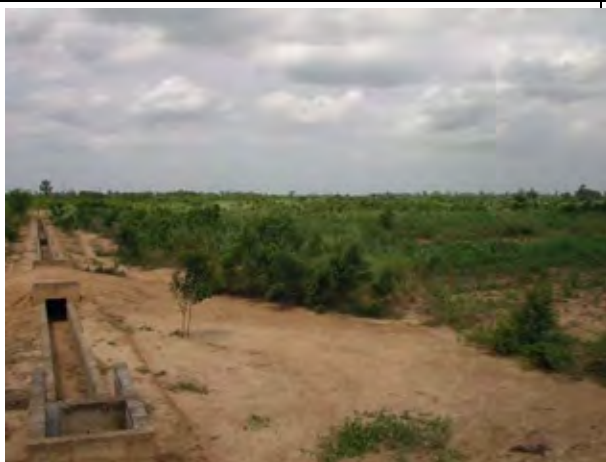
No.1 Secondary canal and its unused commanding area without land reclamation
