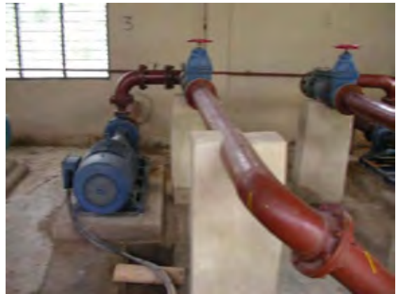
Two types of pump units were installed because of wrong delivery.
