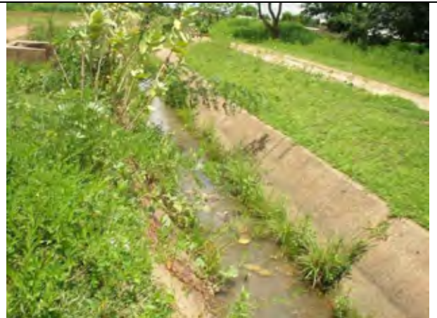
Right Main Canal in the middle part Condition of the canal is fair.
