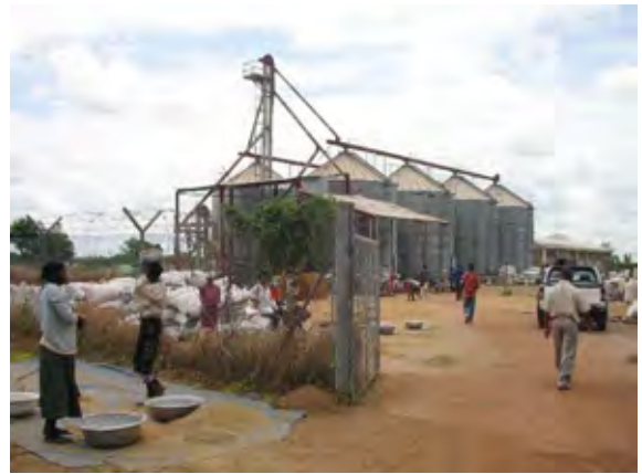
Post harvesting facilities. Silos lost their function due to aging.
