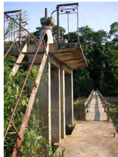
Block-B : Oweri headworks
