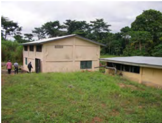
Completed Pump station
