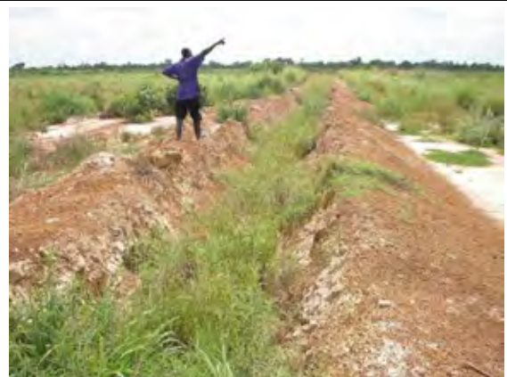
Secondary canal waiting for lining
