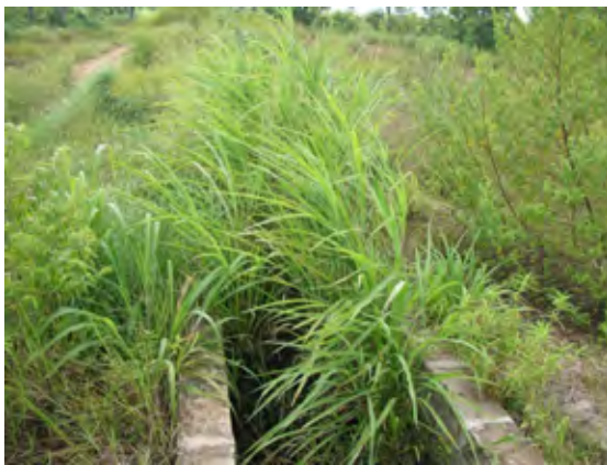
Main canal starting from the weir
