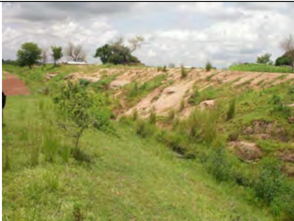
Right Main Canal: Excavated Section Maintenance of open canal system is difficult.
