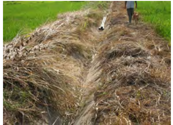
Block-A : a Secondary canal with concrete lining
