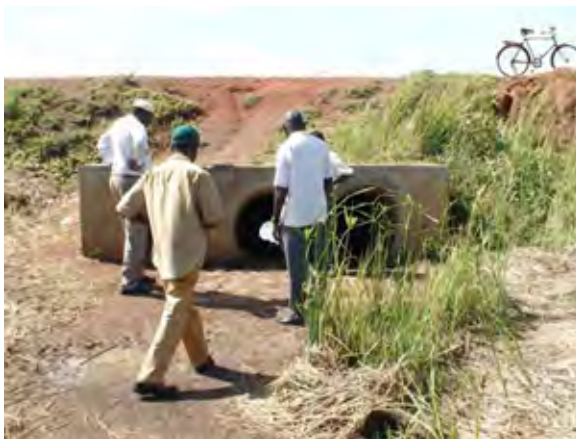
Outlet works for Itek Dam
