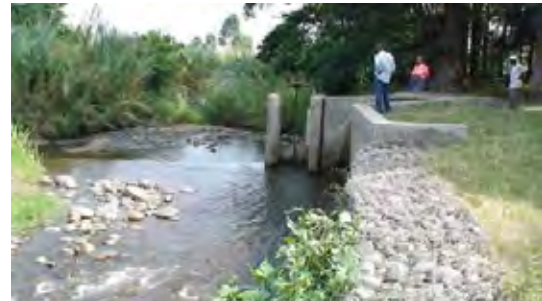
Intake at Mubuku headworks (pipeline)
