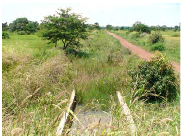
Outlet works and paddy fields downstream
