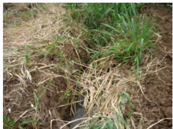
Secondary canal (full of sediment)
