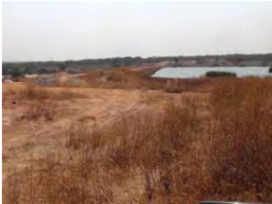
Existing dam and reservoir (aquaculture)
